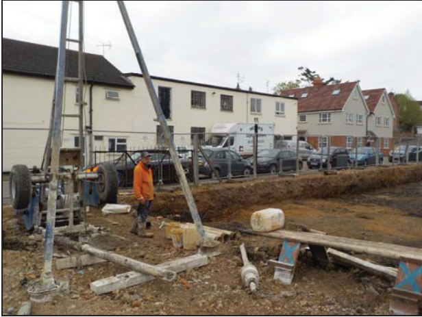
1 General site overview looking south-west
