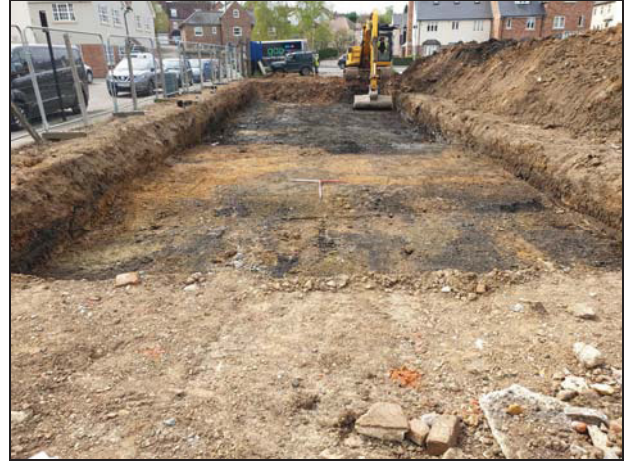
2 Area of excavation looking west
