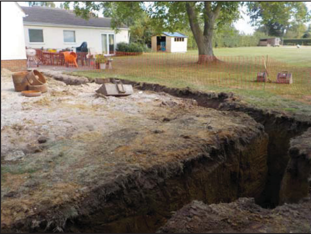
3 Footings trench looking south-east
