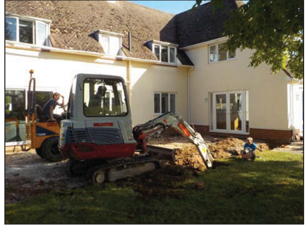
2 Excavation of footings looking north
