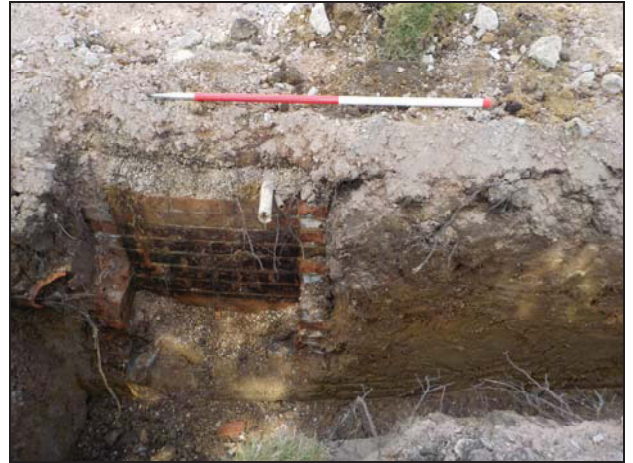
4 Manhole F1004 in Sample section 1 looking north-west
