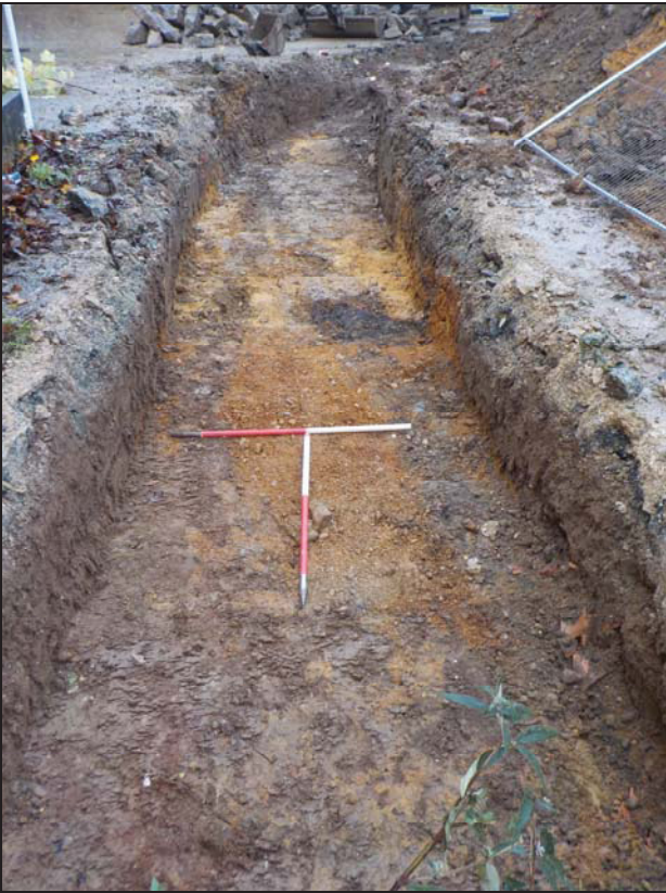
1 Trench 1 looking west
