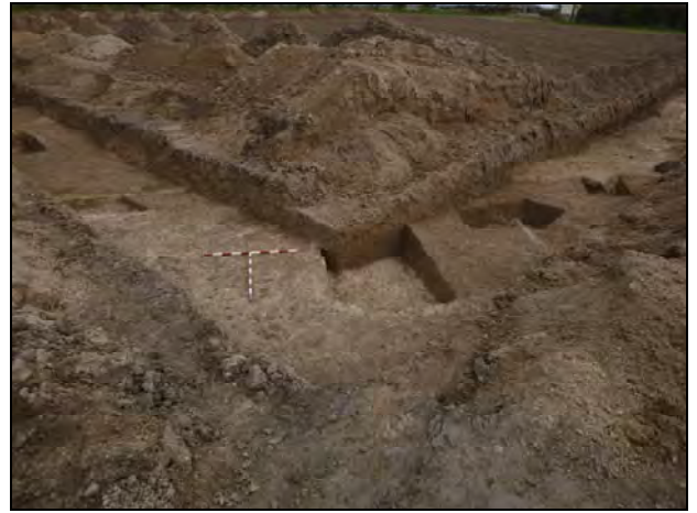
76 Junction of Trenches 30 and 31 looking east
