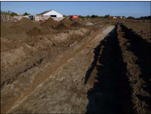
31 Layer 1060 in Trench 10
