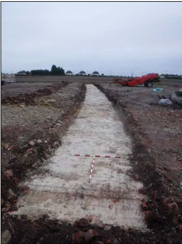
28 Trench 9 looking north-east
