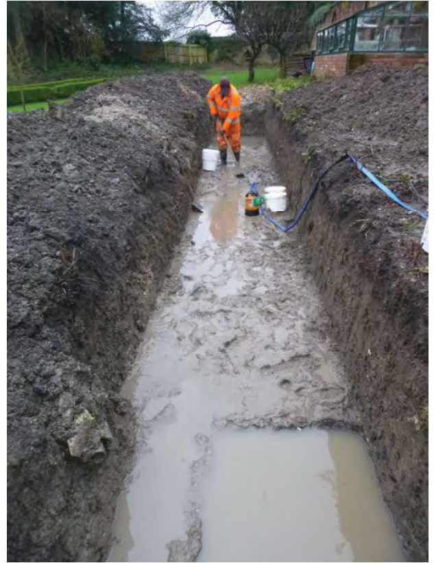
6 Working shot with Test Pit C in the foreground
