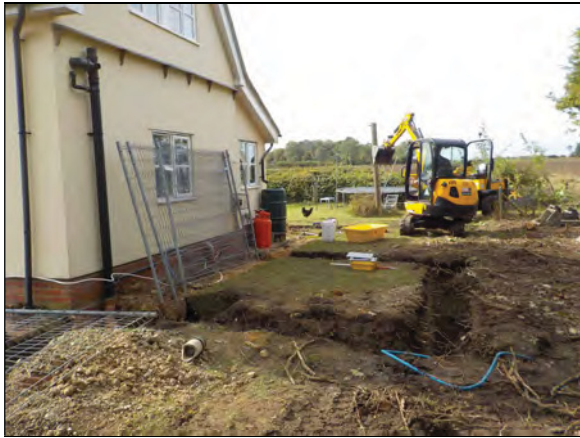
3 Extension footings looking south-west
