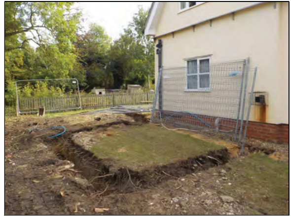
4 Extension footings looking north
