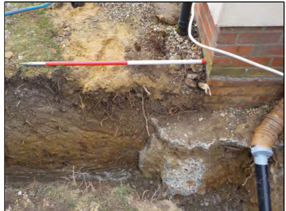
6 Sample section 2 looking south-east
