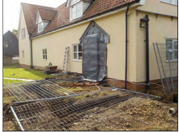
2 Extension footings looking south
