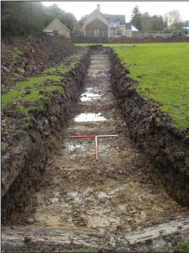
3 Trench 1 looking south
