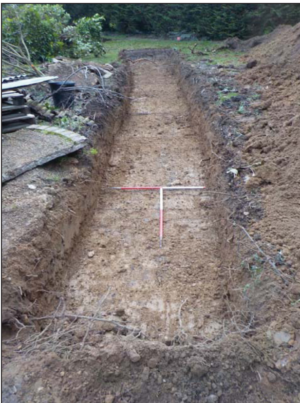
3 Trench 1 looking south-west
