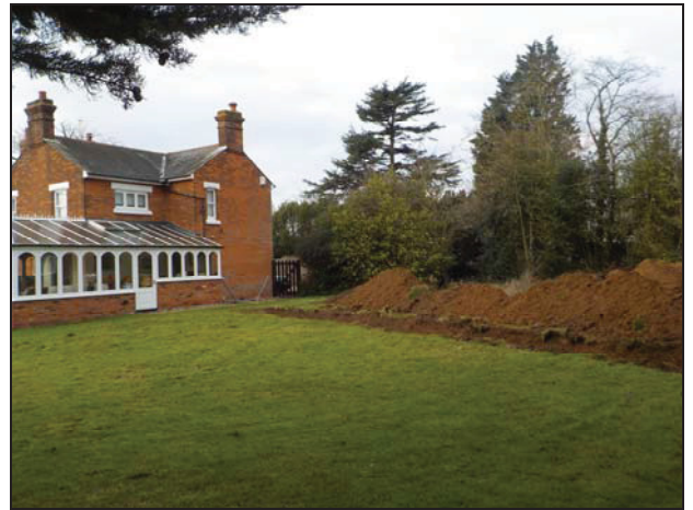
2 General view of site looking north-west
