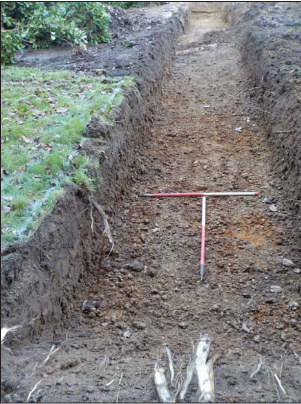
5 Trench 2 looking north-east
