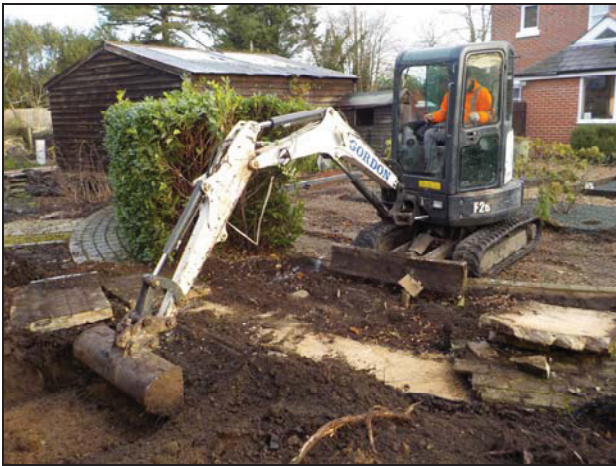
1 Ground being prepared for trench layout
