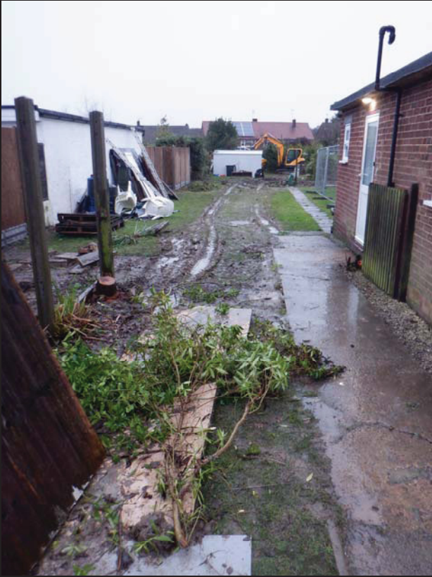
1 View of site entrance before excavation of trenches
