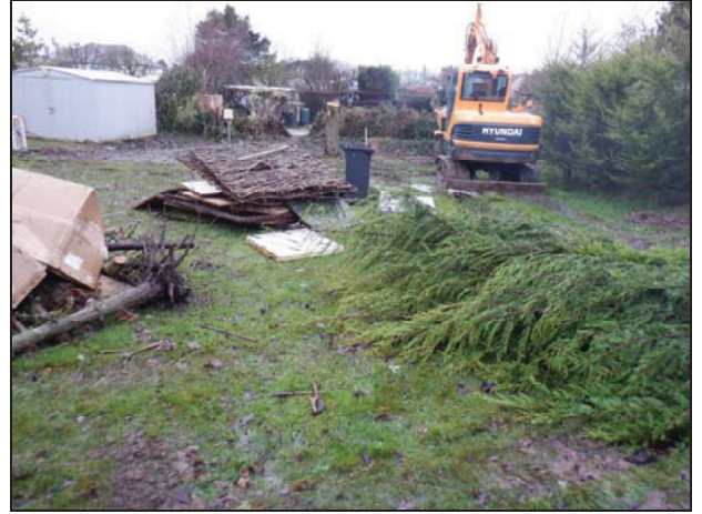
2 General view of site before excavation of trenches
