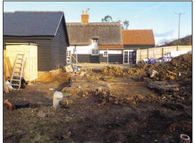
12 General view of site after excavation of trenches
