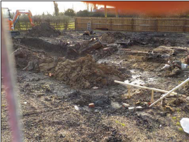
11 General view of site after excavation of trenches
