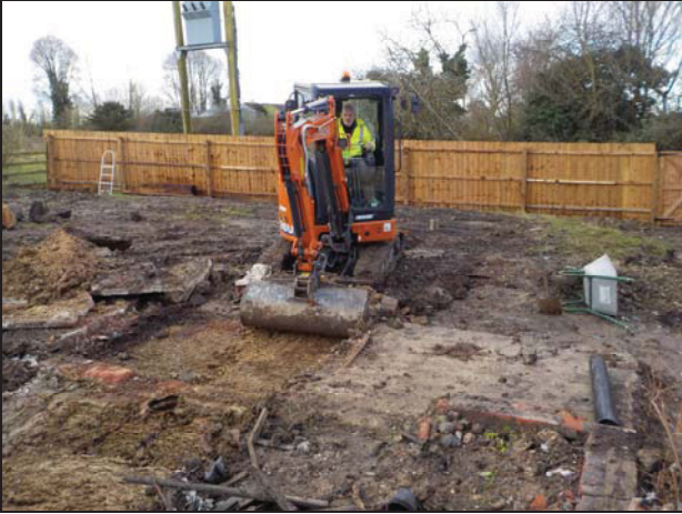
1 General view of site before excavation of trenches
