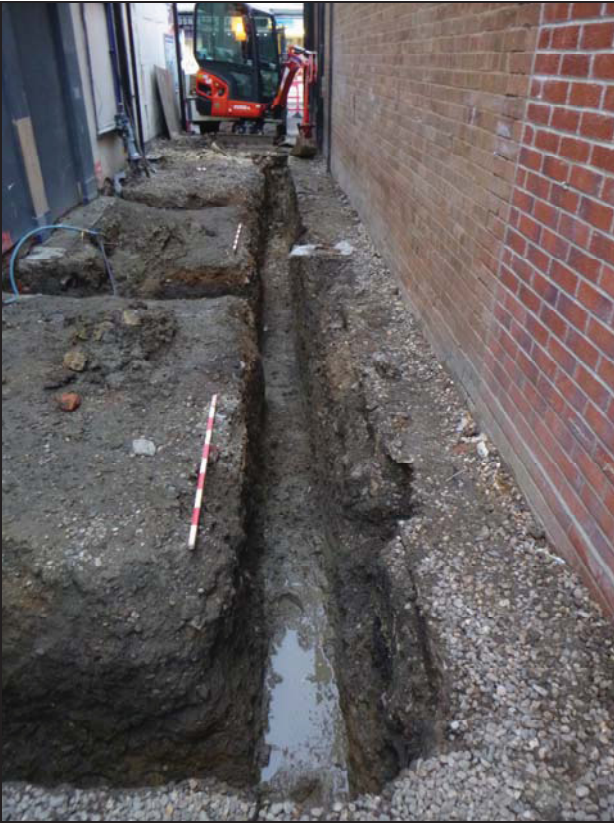
5 New footings looking north-west
