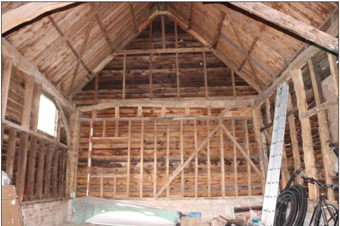
Plate 8 Eastern gable end of the barn, taken from the north-west. (DP 13)
