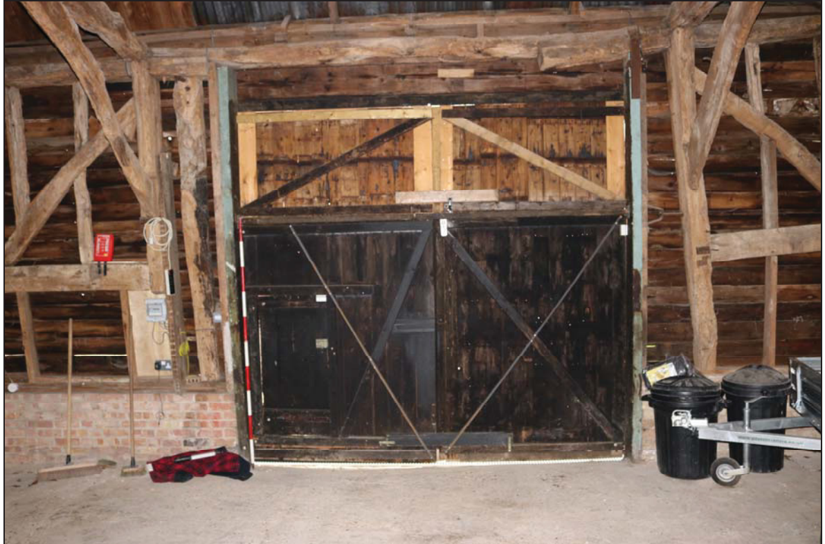
Plate 13 The southern side of Bay 3, taken from the north-east (DP 30)
