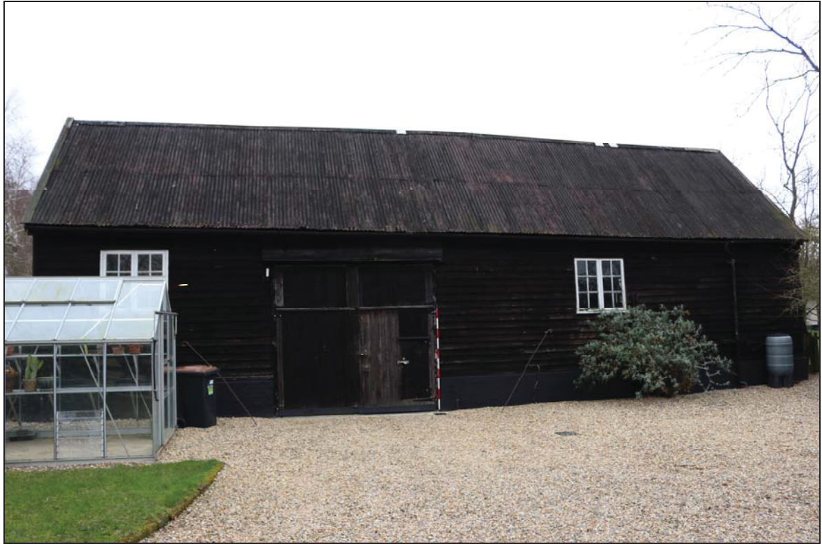
Plate 1 Exterior of the barn, taken from the south-west (DP 04)
