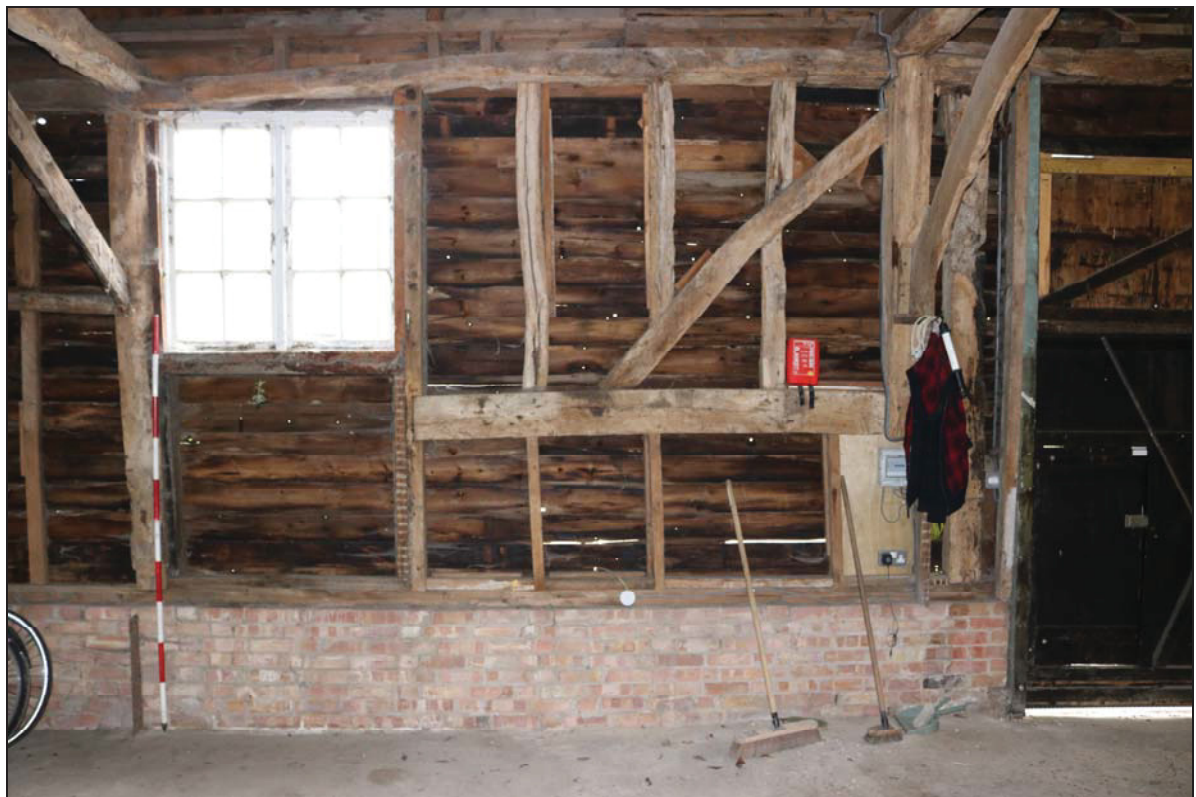
Plate 12 The southern side of Bay 2, taken from the north-east (DP 27)
