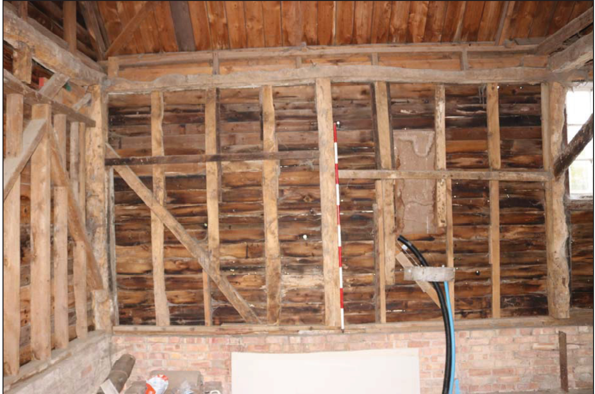
Plate 9 The southern side of Bay 1, taken from the north-east (DP 19)
