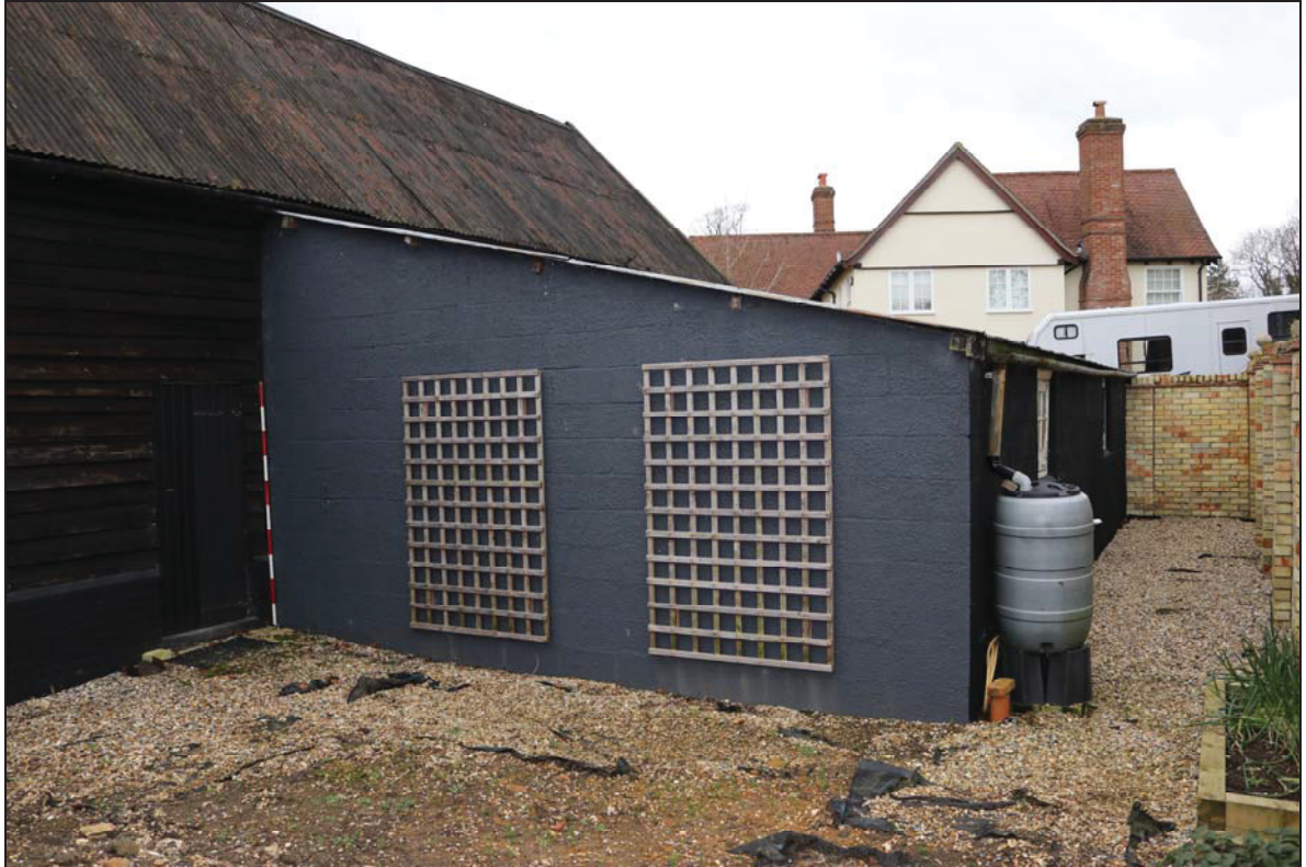
Plate 3 Exterior of the barn, taken from the south-east (DP 09)
