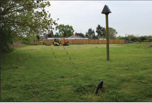
1 View of site looking south-east
