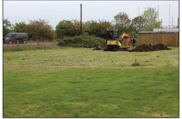
2 View of site looking south
