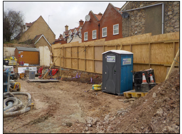
4 View of basement area at piling stage looking north-west
