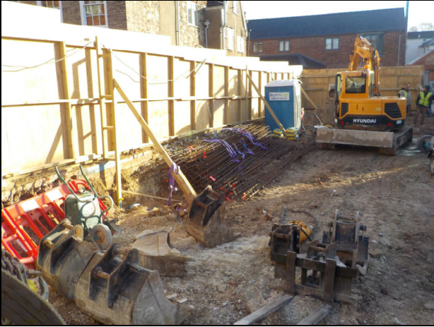
1 View of basement area at piling stage looking north-east
