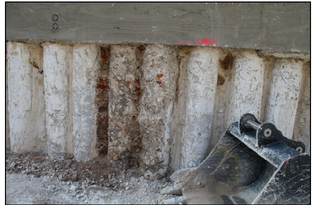
28 Pilings looking south
