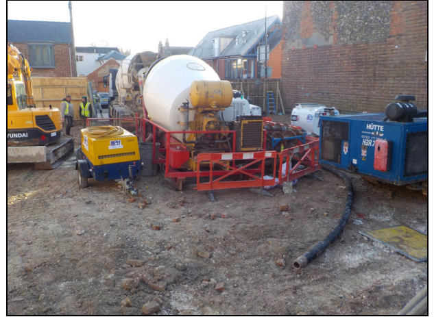
2 View of basement area at piling stage looking east
