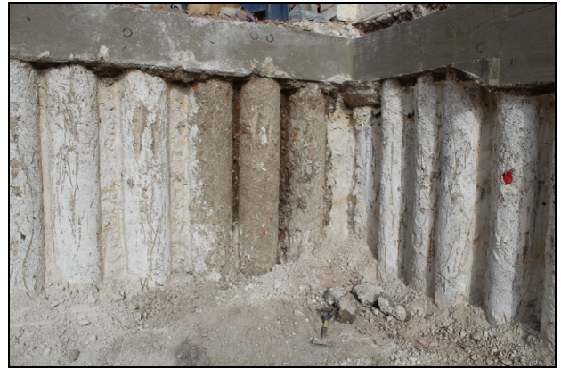
26 Pilings looking west
