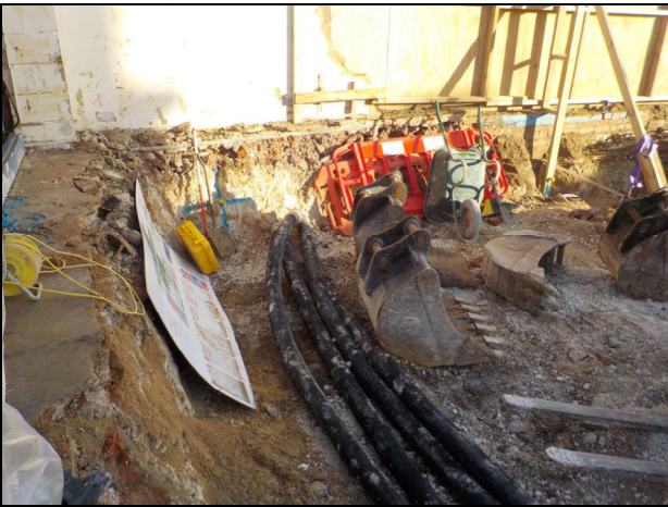
3 View of basement area at piling stage looking north
