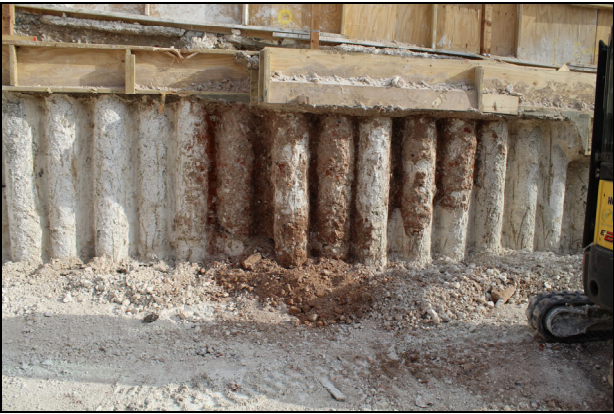
25 Pilings looking north
