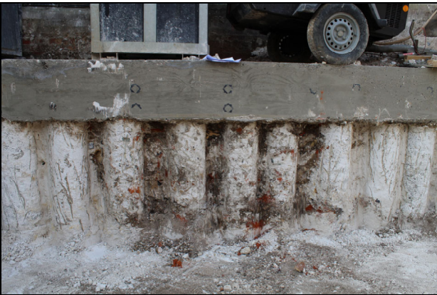
27 Pilings looking south
