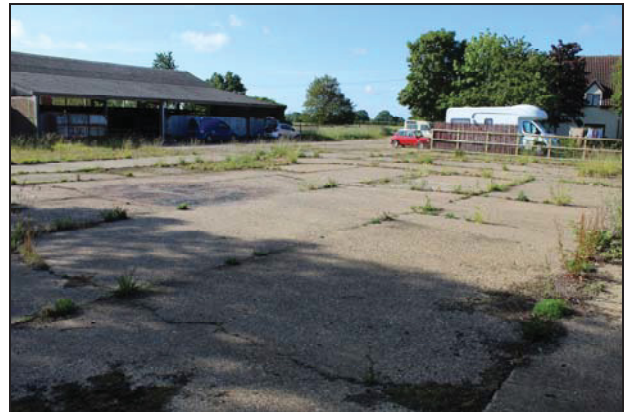
4 View of site looking south-east
