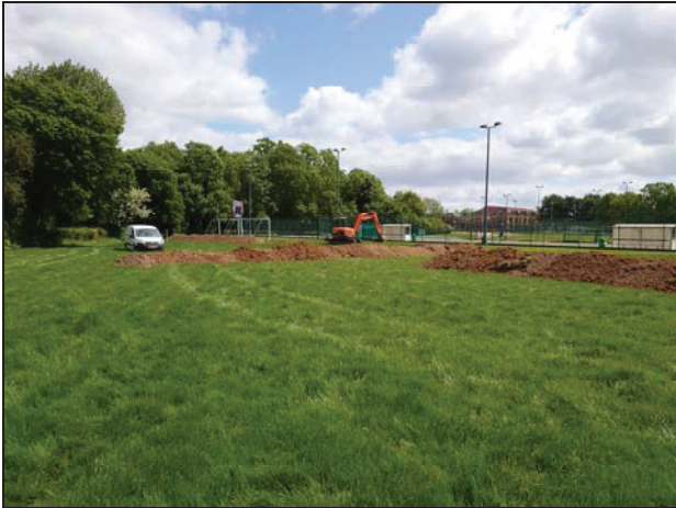
1 General site overview
