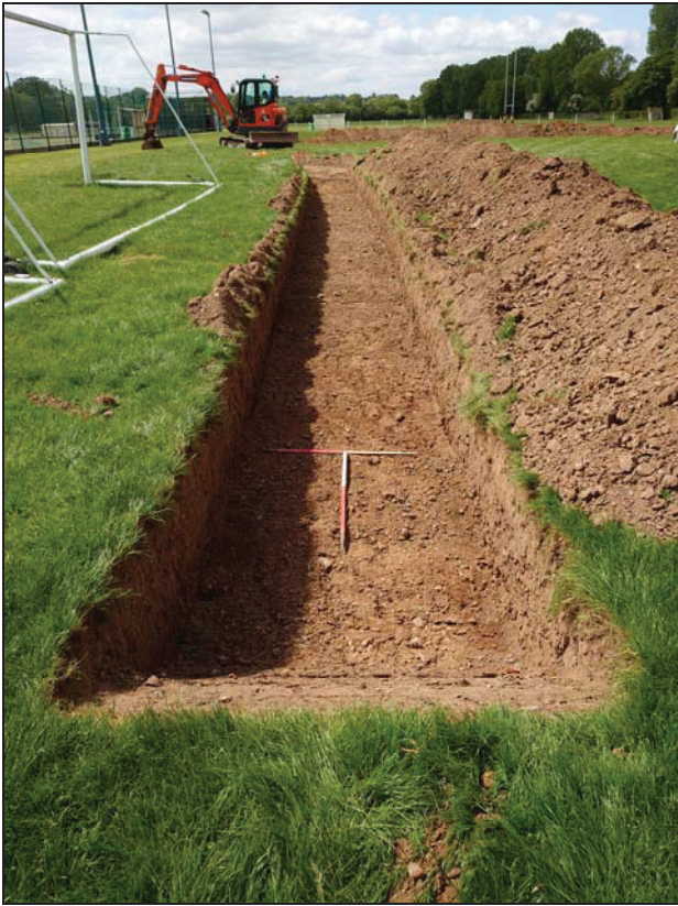
9 Trench 3 looking south-west
