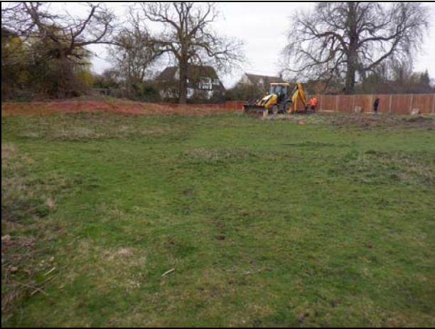
1 General site overview
