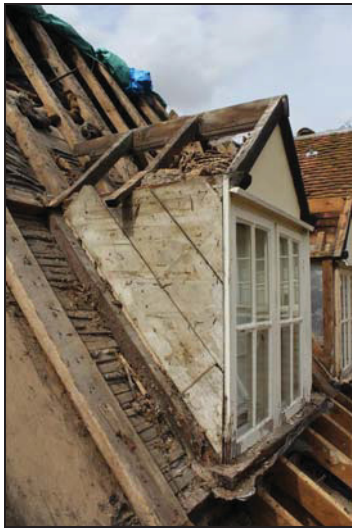
East side of Range 1 (Bay 1: north end) showing wall-plate with surviving studs, taken from the east
