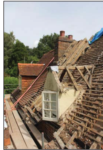
64 West roof pitch of Ranges 1 and 4, taken from the south-west
