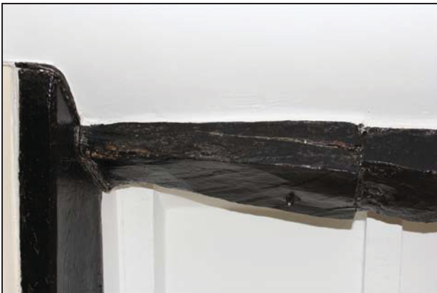
Cupboard in the south-east corner of Room FF07 (Range 1) showing timber-framing including a corner post with tie-beam and wall-plate and section of brace visible on the left, taken from the north-west
