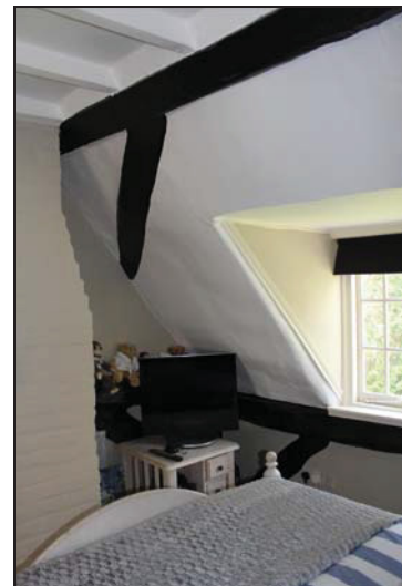
West side of Room FF07 (Range 1) showing exposed timber elements including a wind brace, taken from the north-east
