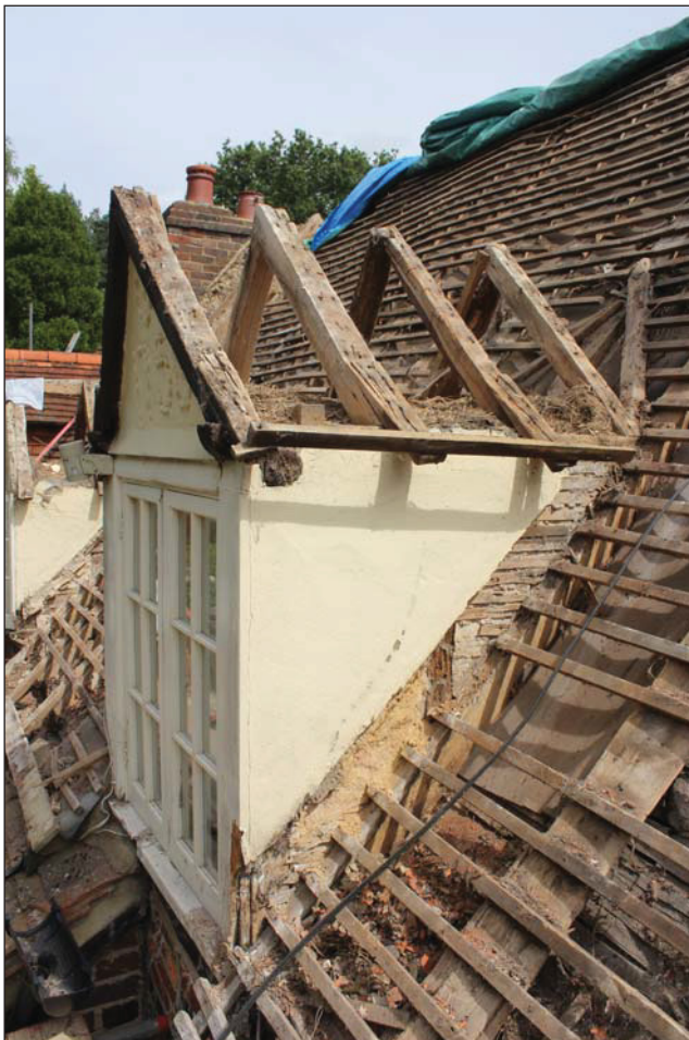
Plate 10 Dormer window (Bay 2: west side), taken from the south (DP 61)
