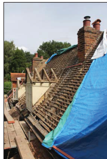
66 West roof pitch, taken from the south-west
