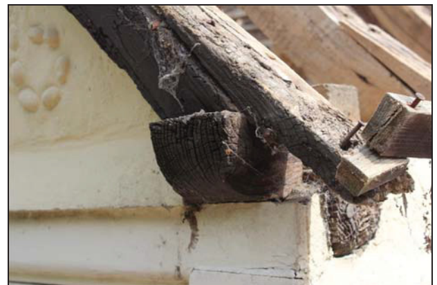
Detail of the dormer window (Range 1: Bay 2, west side) showing rafter couples with no ridgeboard, taken from the north-west
