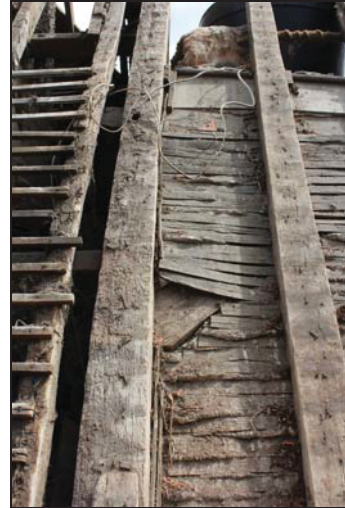
West roof pitch of Range 1 (Bay 1: north end) showing principal rafter and adjoining rafter with wind brace behind the lath and plaster, taken from the west
