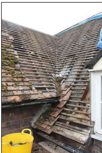
Detail of the dormer window (Range 4: west side) showing rafter couples to a ridgeboard, taken from the south-west
