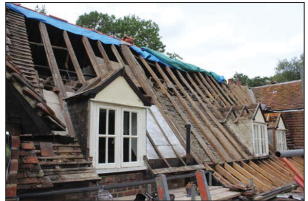
West roof pitch of Range 1 (Bay 1: north end) showing principal rafter and adjoining rafter with wind brace behind the lath and plaster, taken from the west
