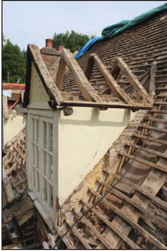
61 Dormer window (Range 1: Bay 2, west side), taken from the south
