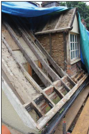
View of the west side of Ranges 1 and 2 during removal of the roof cladding, taken from the west
