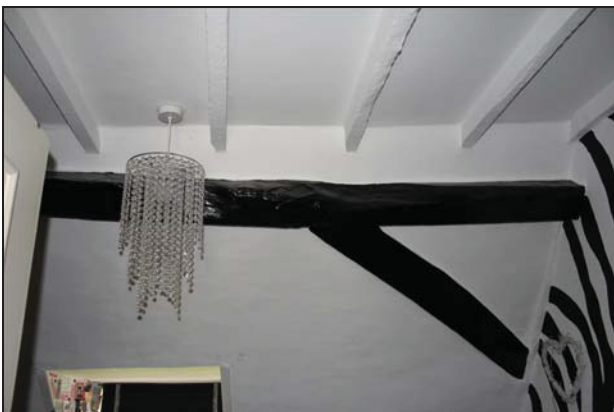
Crude scarf joint in the purlin on the east side of Range 1 (FF05), taken from the west
