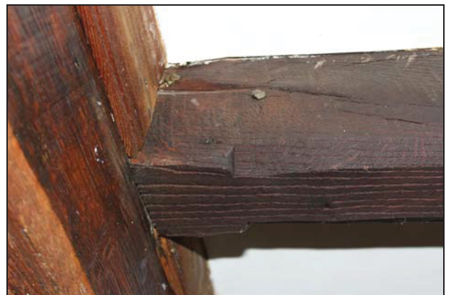
Lambs tongue chamfer stop on the ceiling joists in Room GF03 (Range 1), taken from the east
