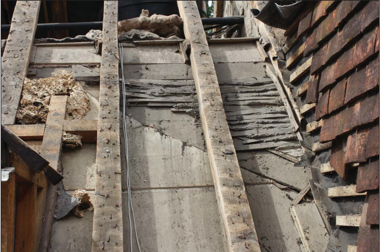
Plate 8 East roof pitch of the historic core (Bay 1: north end) showing wind brace with lath and plaster above and replacement boarding below, taken from the east (DP 77)
