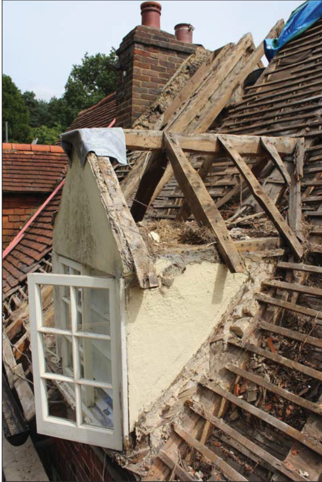
Plate 9 Dormer window (Bay 1: west side), taken from the south (DP 56)
