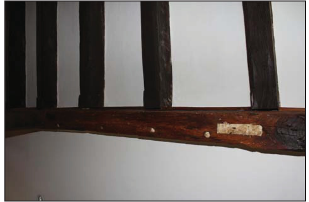
Binding joist between Rooms GF03 and 04 showing redundant mortices for staves and studs (Range 1), taken from the east
