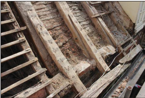
West roof pitch of Range 1 (Bay 1: south end) showing principal rafter with pegged collar and weathered projecting purlin end, taken from the west
