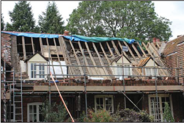
View of the east side of Ranges 1 and 2 during removal of the roof cladding, taken from the east
