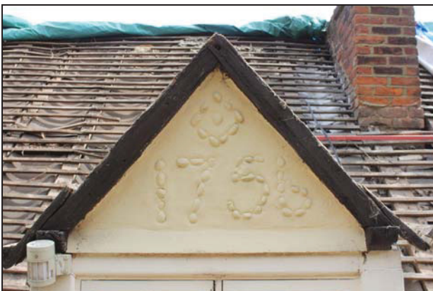
Detail of the dormer window (Range 1: Bay 2, west side) showing gable with modern cement render infill, taken from the west
