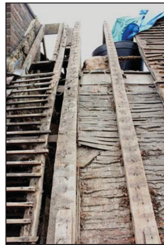
Binding joist between Rooms GF03 and 04 showing redundant mortices for staves and studs (Range 1), taken from the east
