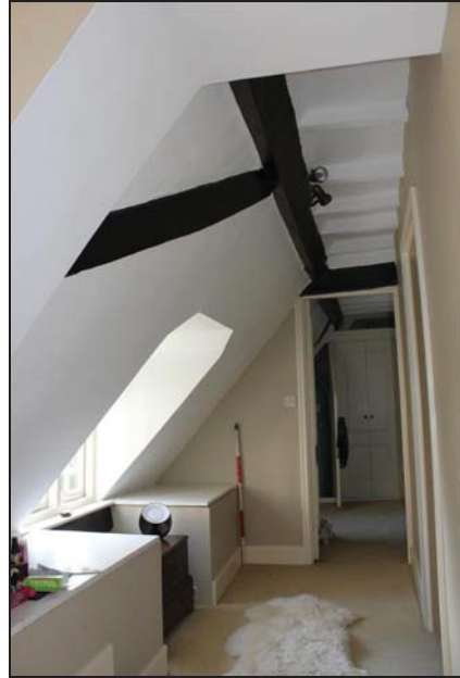
Corridor FF05 on the east side of Range 1 showing exposed roof timbers including a wind brace, taken from the north
