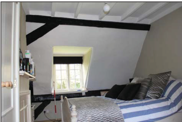
View of the timber-framing of the south end of Range 1 visible within Room FF08 (Range 2), taken from the south
