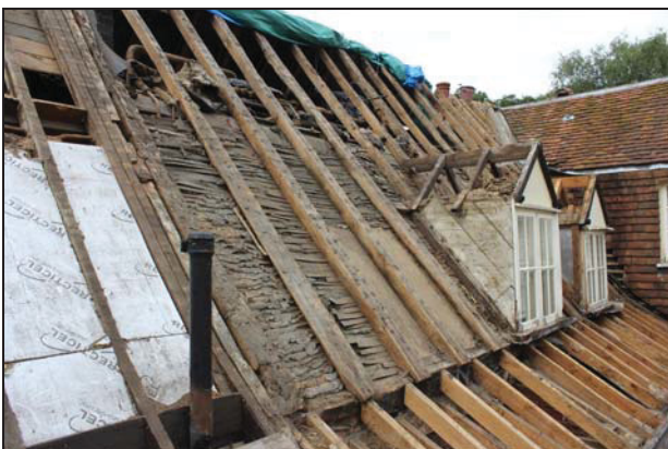
West roof pitch of Range 1 (Bay 1: north end) showing nailed rafter feet, taken from the north-west
