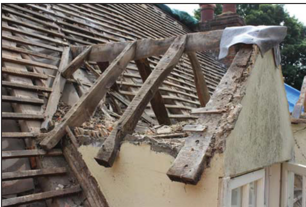
Detail of the dormer window (Range 1: Bay 1, west side) showing slender rafter couples to a ridgeboard, taken from the north
