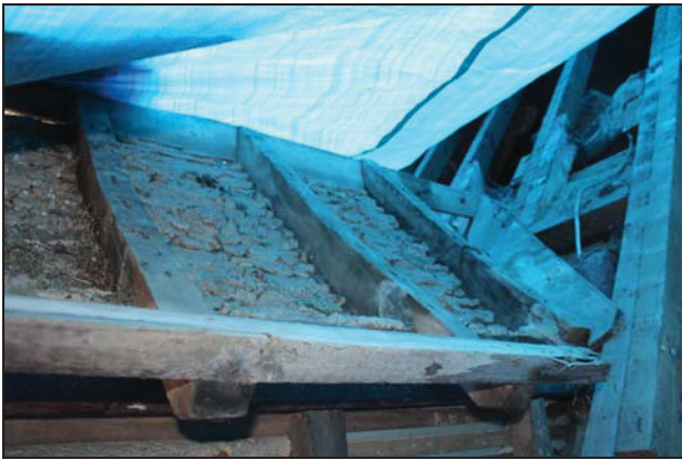
Detail of the dormer window (Range 4: west side) showing rafter couples to a ridgeboard, taken from the south-west
