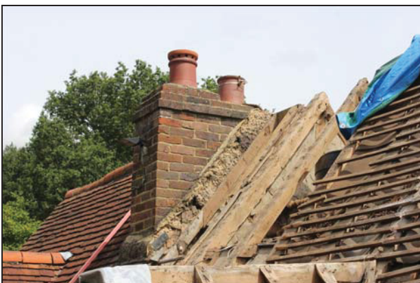
63 West roof pitch of the historic core (Range 1: Bay 2, south end) showing rafters truncated by the insertion of the chimney stack, taken from the west
