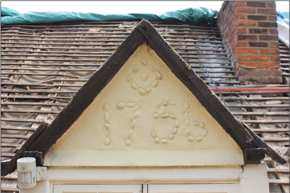
Plate 11 Detail of the dormer window (Bay 2: west side) showing gable with modern cement render infill and an early date, taken from the west (DP 59)
