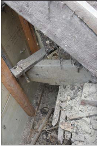
Detail of the west roof pitch Range 4 showing truncated tie-beam, taken from the north
