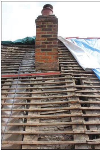
63 West roof pitch of the historic core (Range 1: Bay 2, south end) showing rafters truncated by the insertion of the chimney stack, taken from the west
