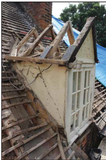
West roof pitch of Range 1 (Bay 1) showing principal rafters above the dormer window, taken from the west
