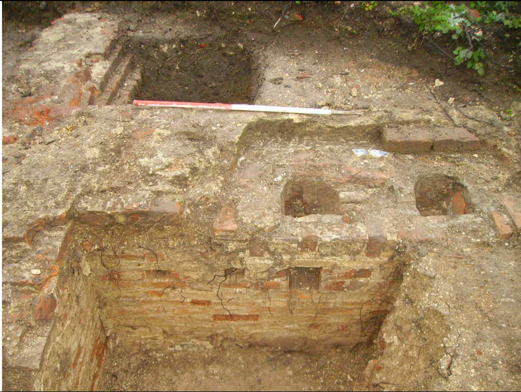
Plate 10: Phase 6 Wall M1786 with possible plumbing features, from south
