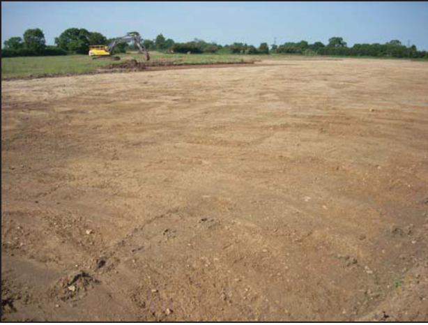
DP1 Area 1: Topsoil stripping, view south-west
