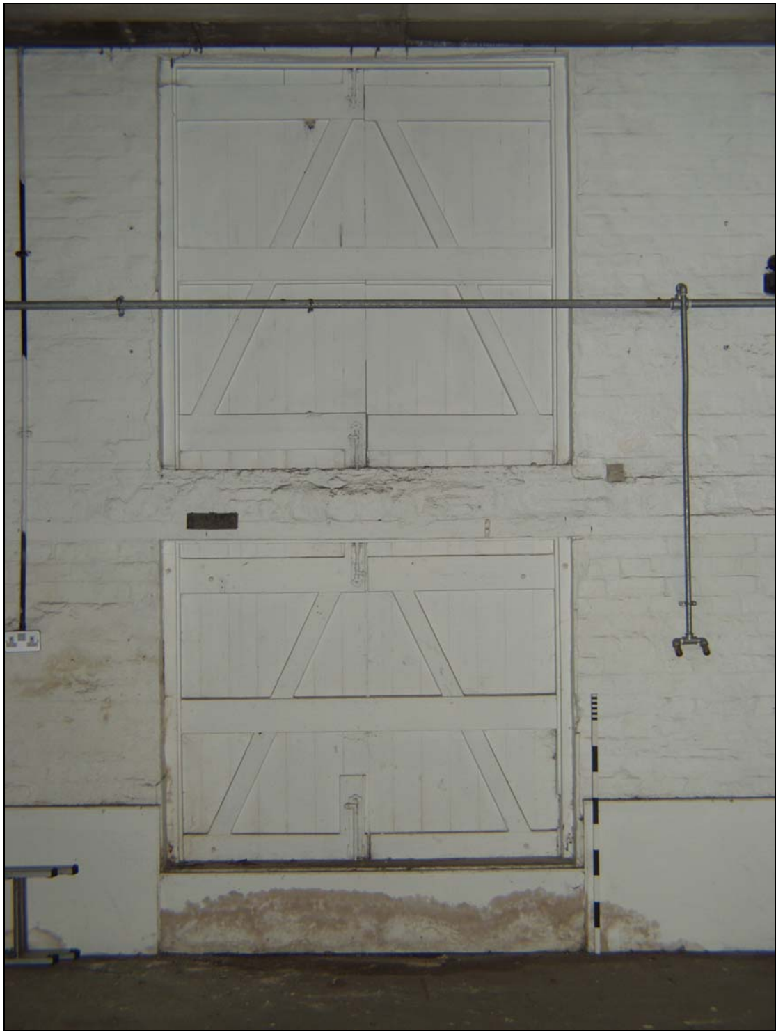
9 Loading doors to central section, taken from the south (40)
