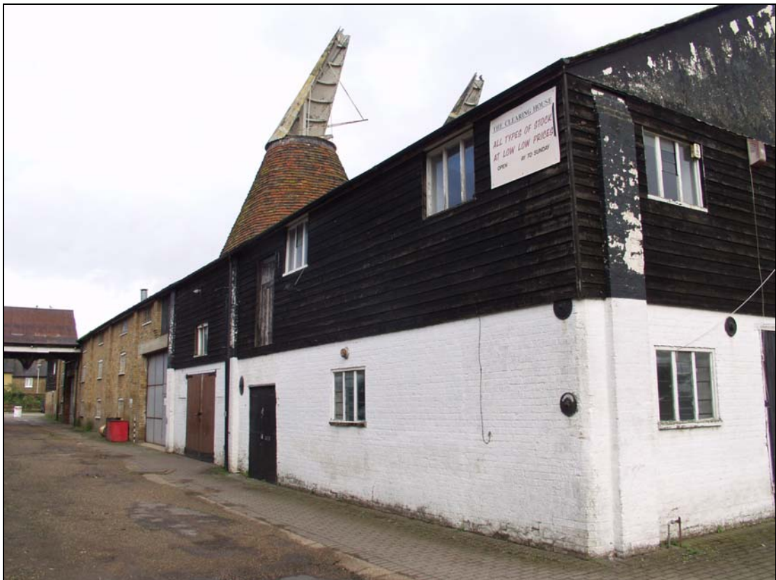
2 Southern elevation taken from the south-east (3)
