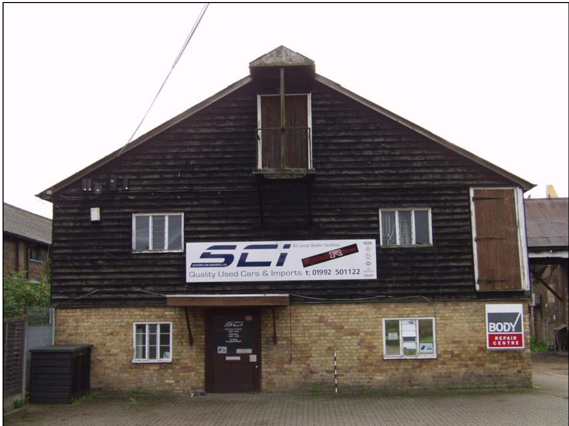
5 Western elevation taken from the west (1)
