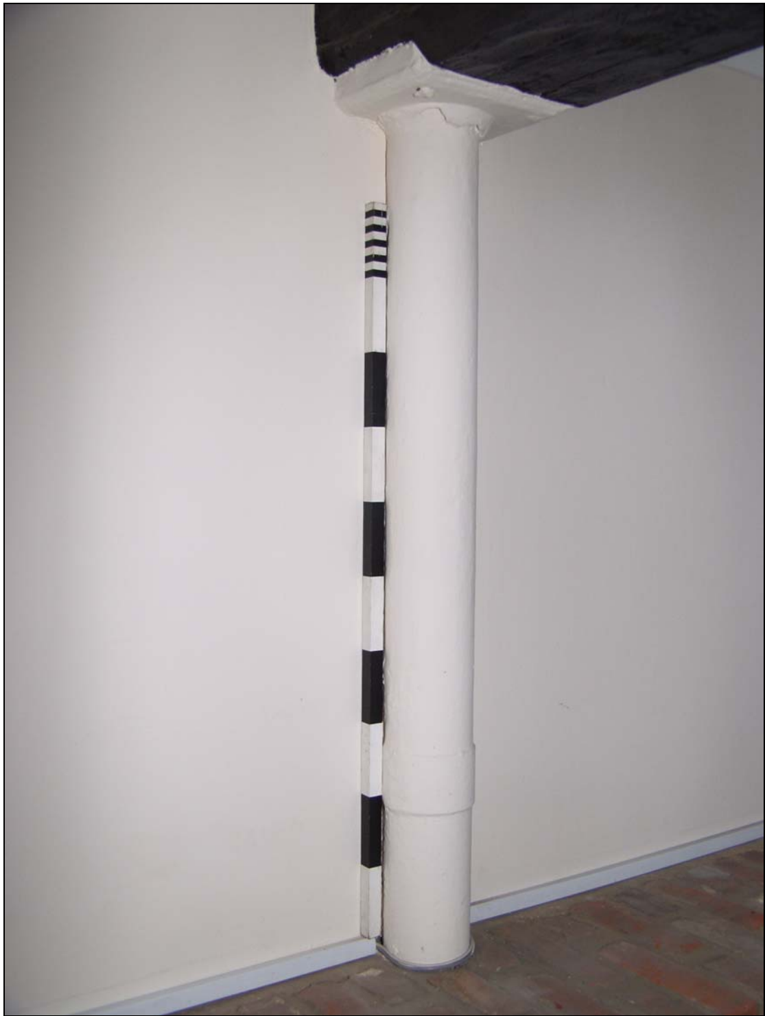
13 Detail of surviving iron stanchion (42)
