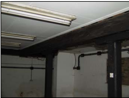
Wooden columns and [?] joist to ground floor of eastern section, taken from the south-east
