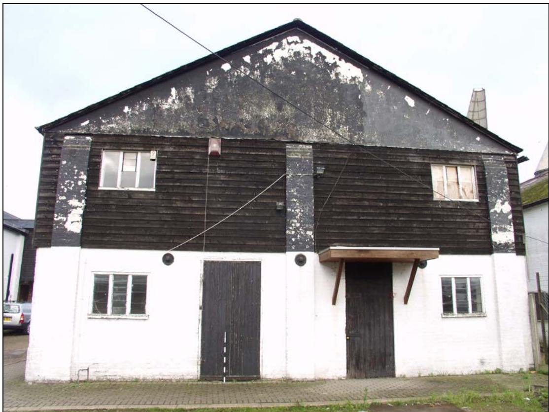
6 Eastern elevation taken from the east (4)
