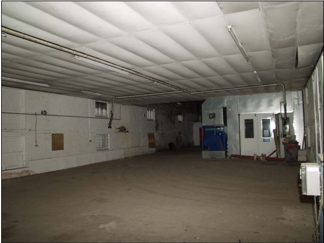
7 Internal view of central area taken from the south-west (6)
