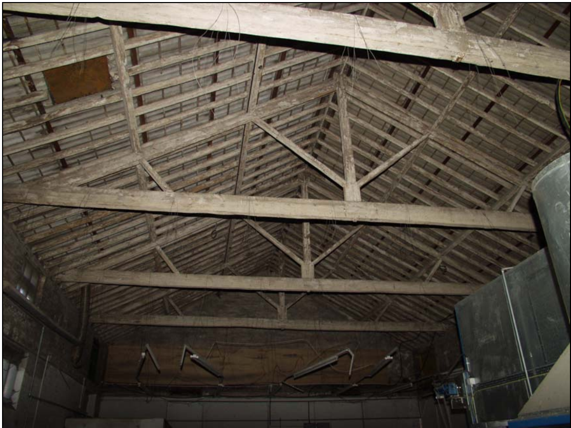
12 Roof trusses in the central section taken from the west (13)
