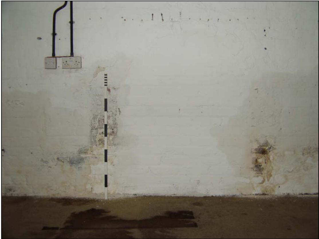
20 Blocked archway to west wall of ground floor of eastern section, taken from the east (31)
