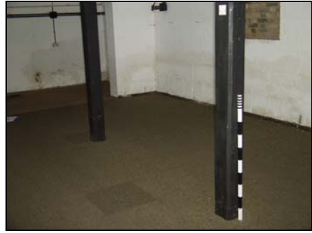
Wooden columns and slate damp proof course to ground floor of eastern section, taken from the south-east
