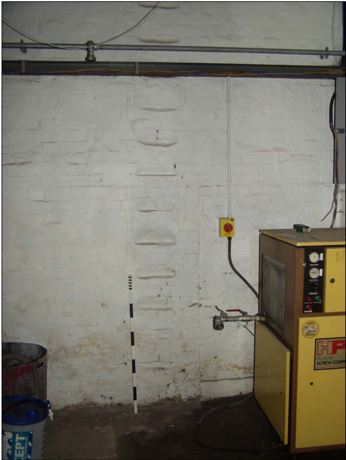
10 Detail of former position of ladder (41)
