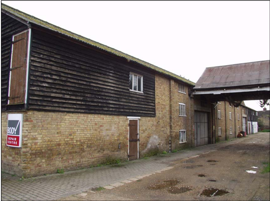
1 Southern elevation taken from the south-west (2)
