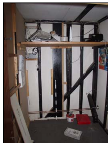
Modern timber framed partition to north of staircase on first floor of west section taken from the east
