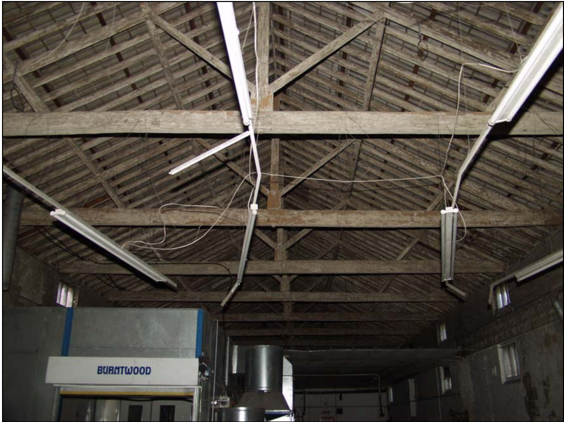
11 Roof trusses in the central section taken from the east (14)
