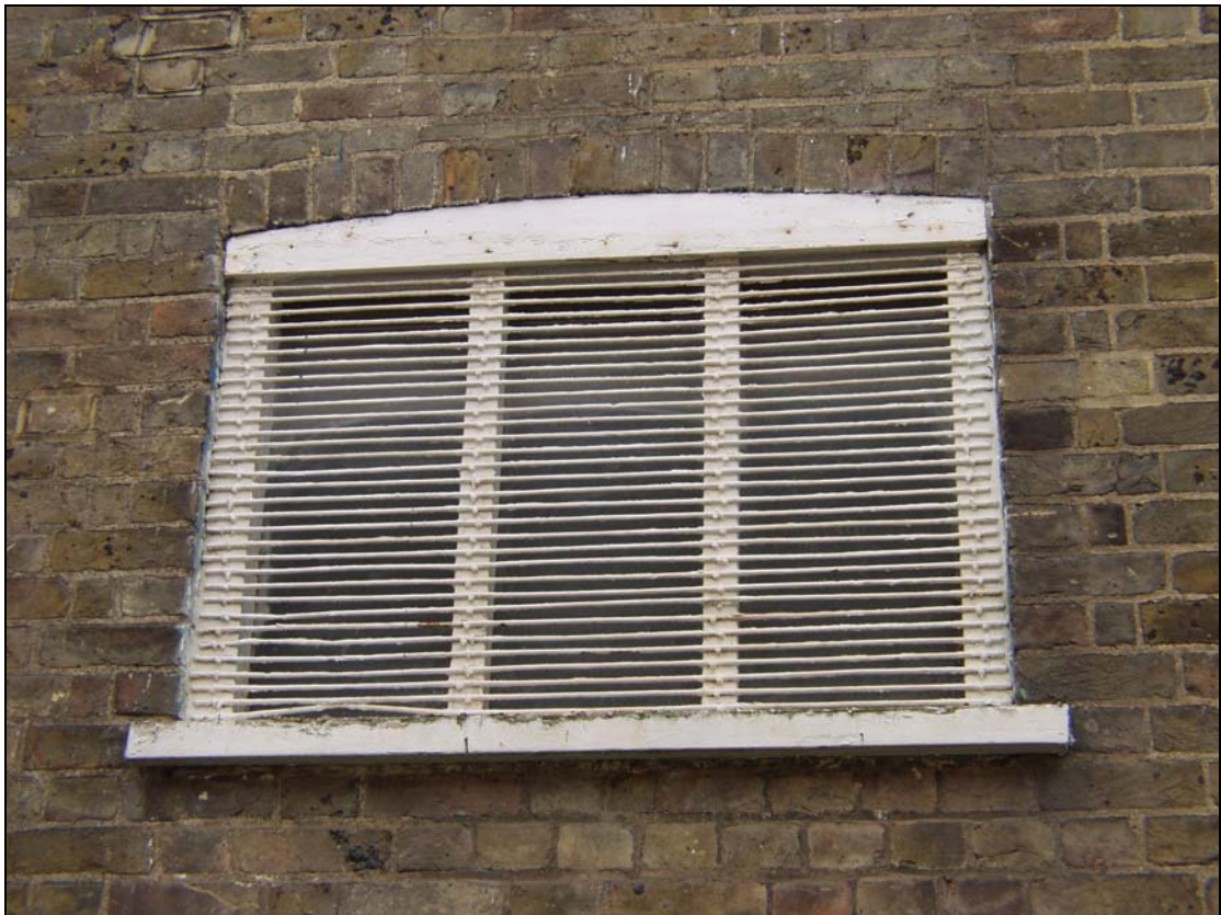
4 Typical central section window taken from the north (39)
