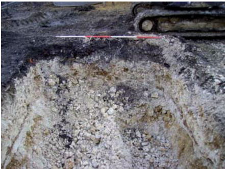
DP 5 Sample Section 8 (Soakaway), view south-east
