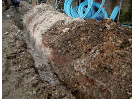
DP 2 Service trench excavated 17/02/07, view north
