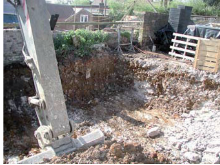
DP 8 Excavation of garden/car park area, view south-west
