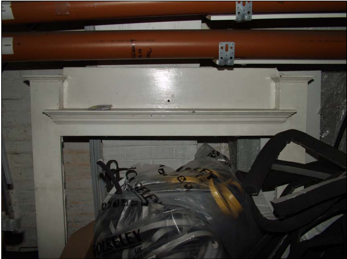
25 Redundant early 20th century fireplace in garage (10)
