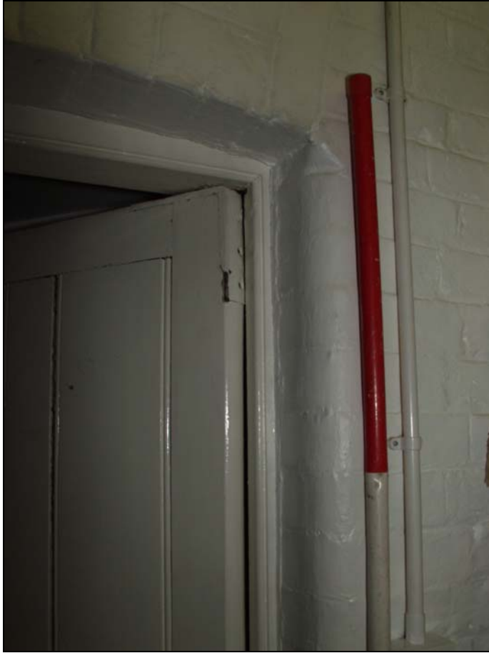
23 Pintle-hung, non-locking door to possible former lavatory (27)
