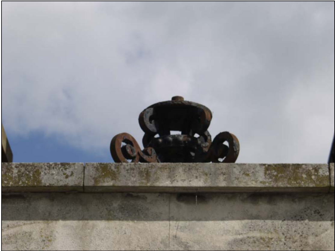
7 Lamp fitting taken from the west (54)
