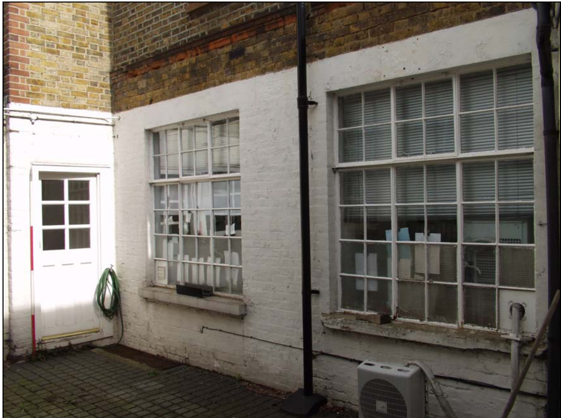
16 Ground floor of the eastern range from the central yard (9)
