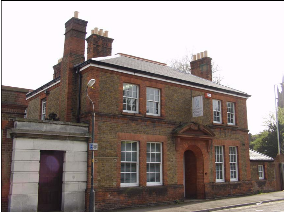
1 Western elevation of domestic range, taken from the north-west (1)
