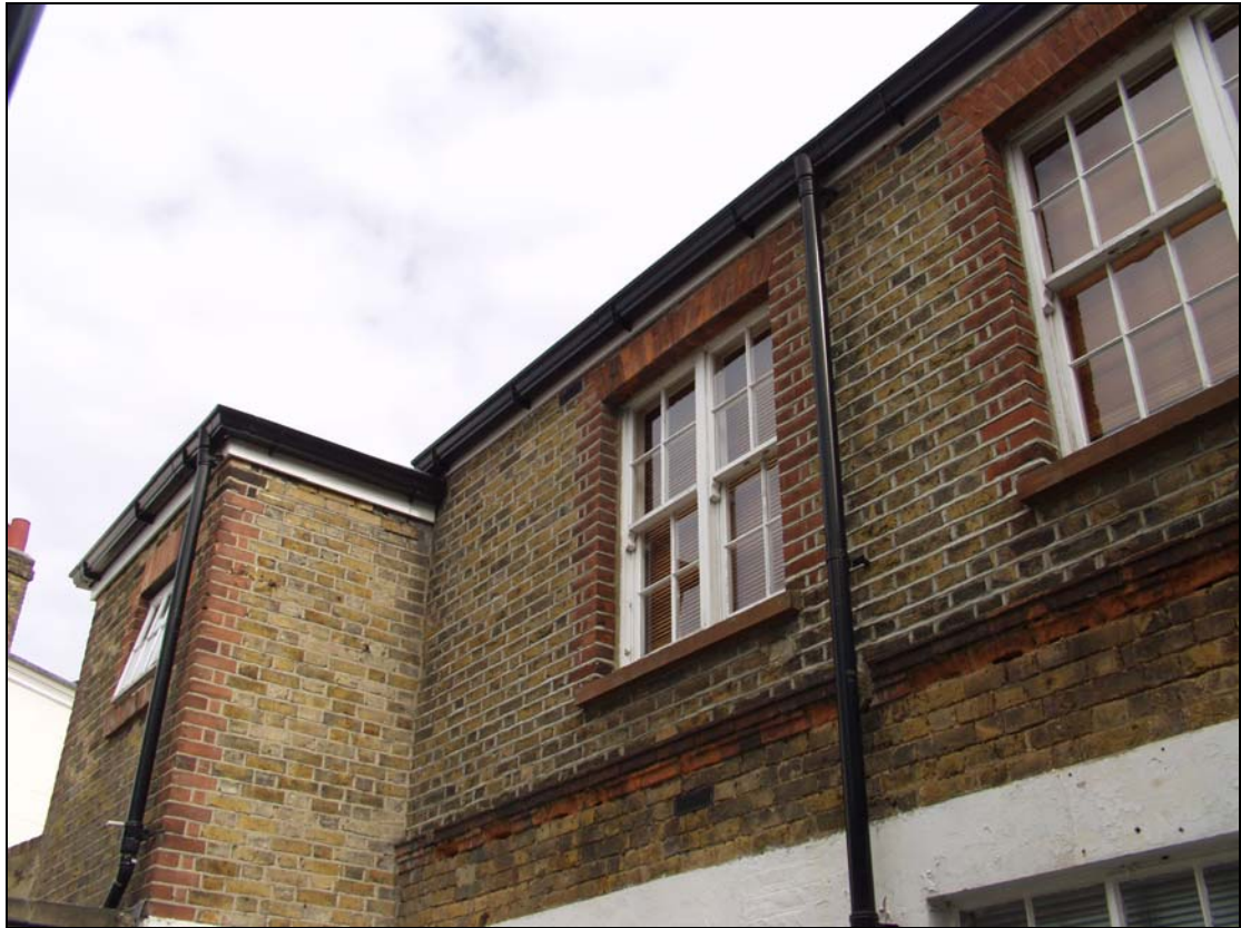
15 First floor of the eastern range from the central yard (8)
