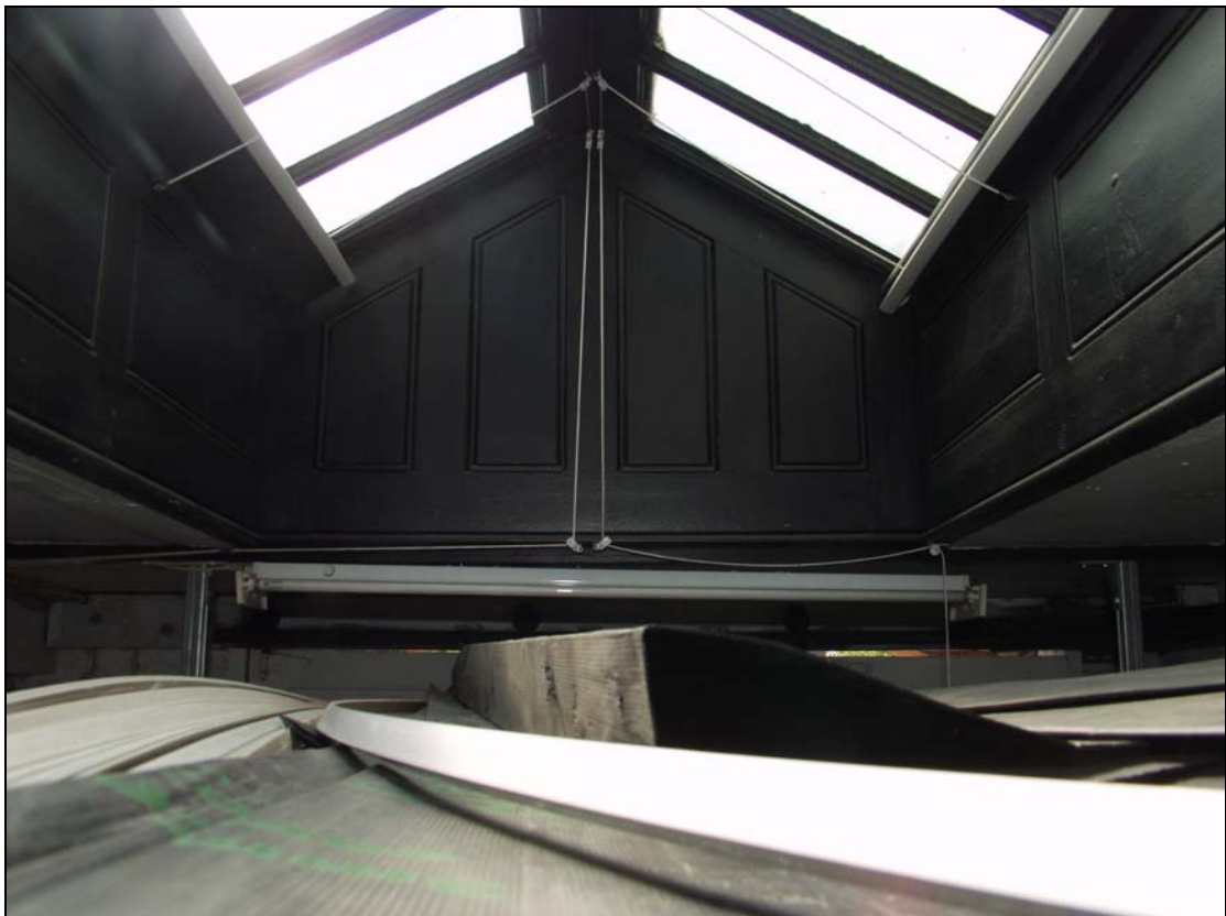
24 Internal roof structure of garage (12)
