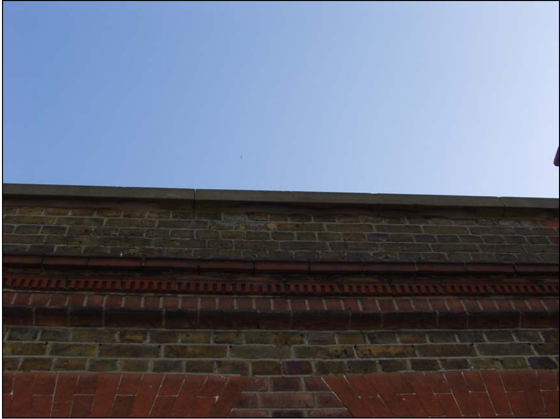
4 Square modillion decoration on western elevation of northern range (17)
