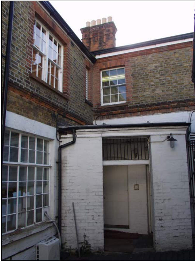
9 Porch and central yard, taken from the north (15)
