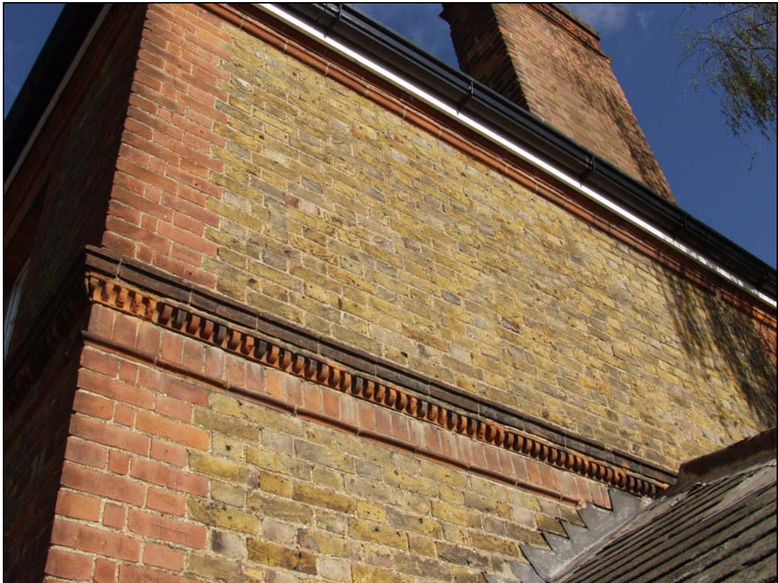
5 Rounded modillion decoration on southern elevation of domestic range (18)
