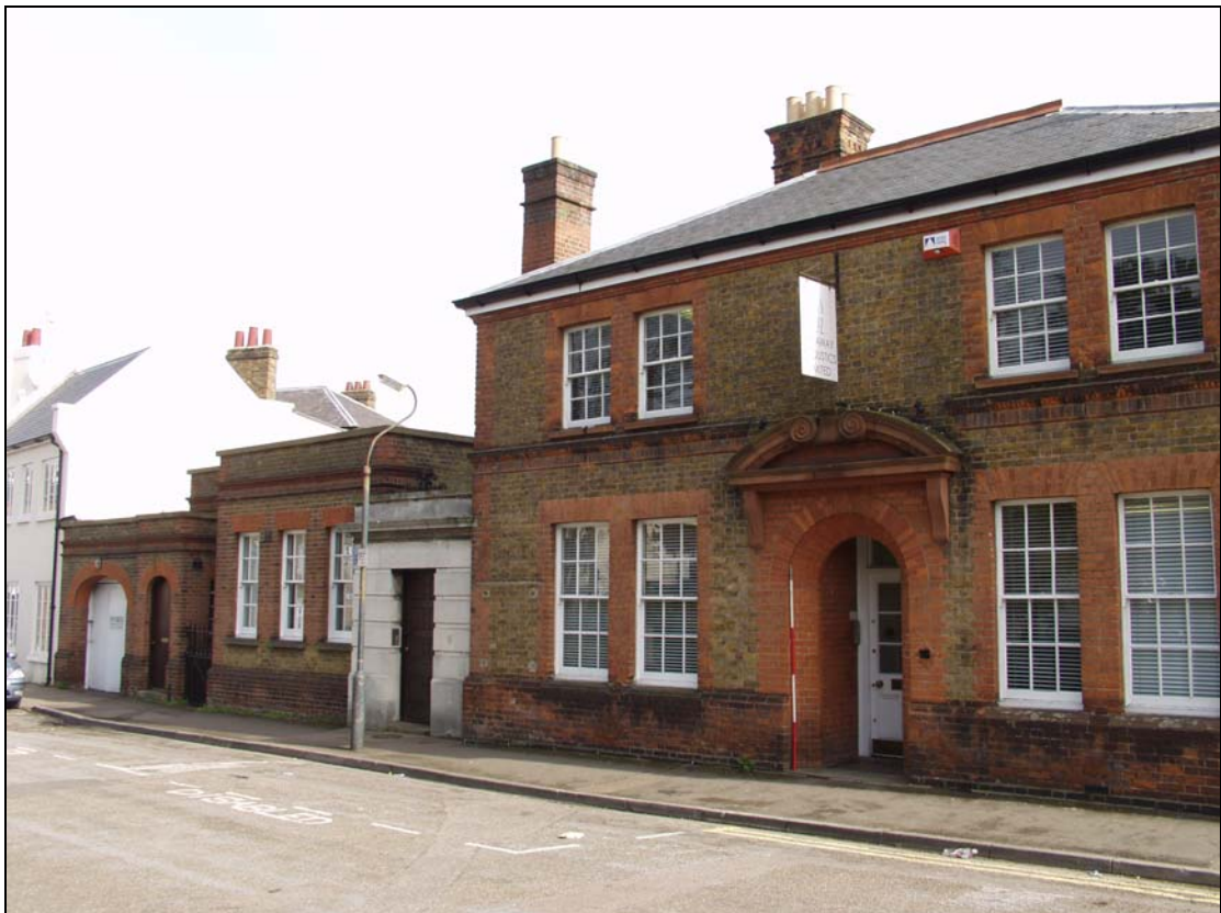
2 General view of western elevation, taken from the south-west (2)
