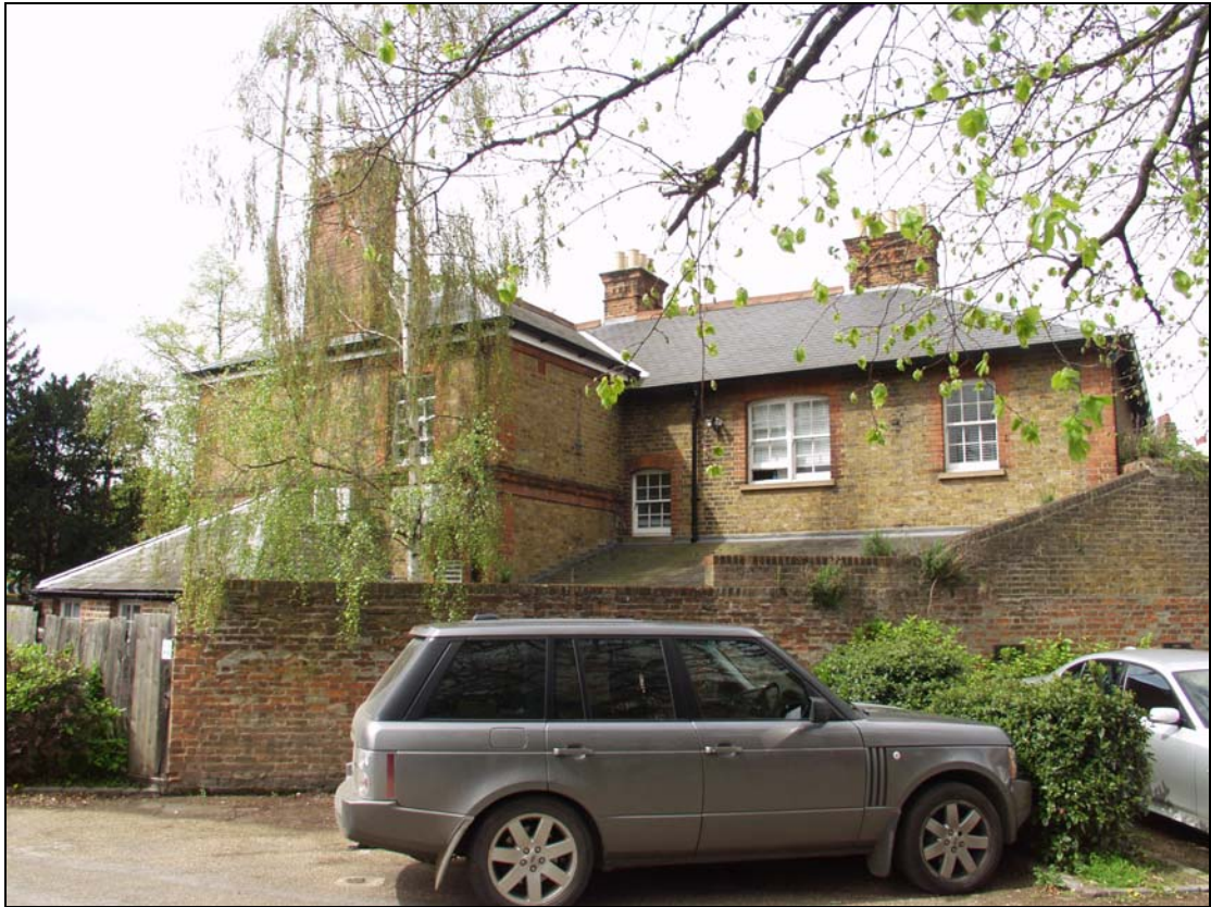
17 South elevation as seen from Bayley Mews Car Park, taken from the south (57)
