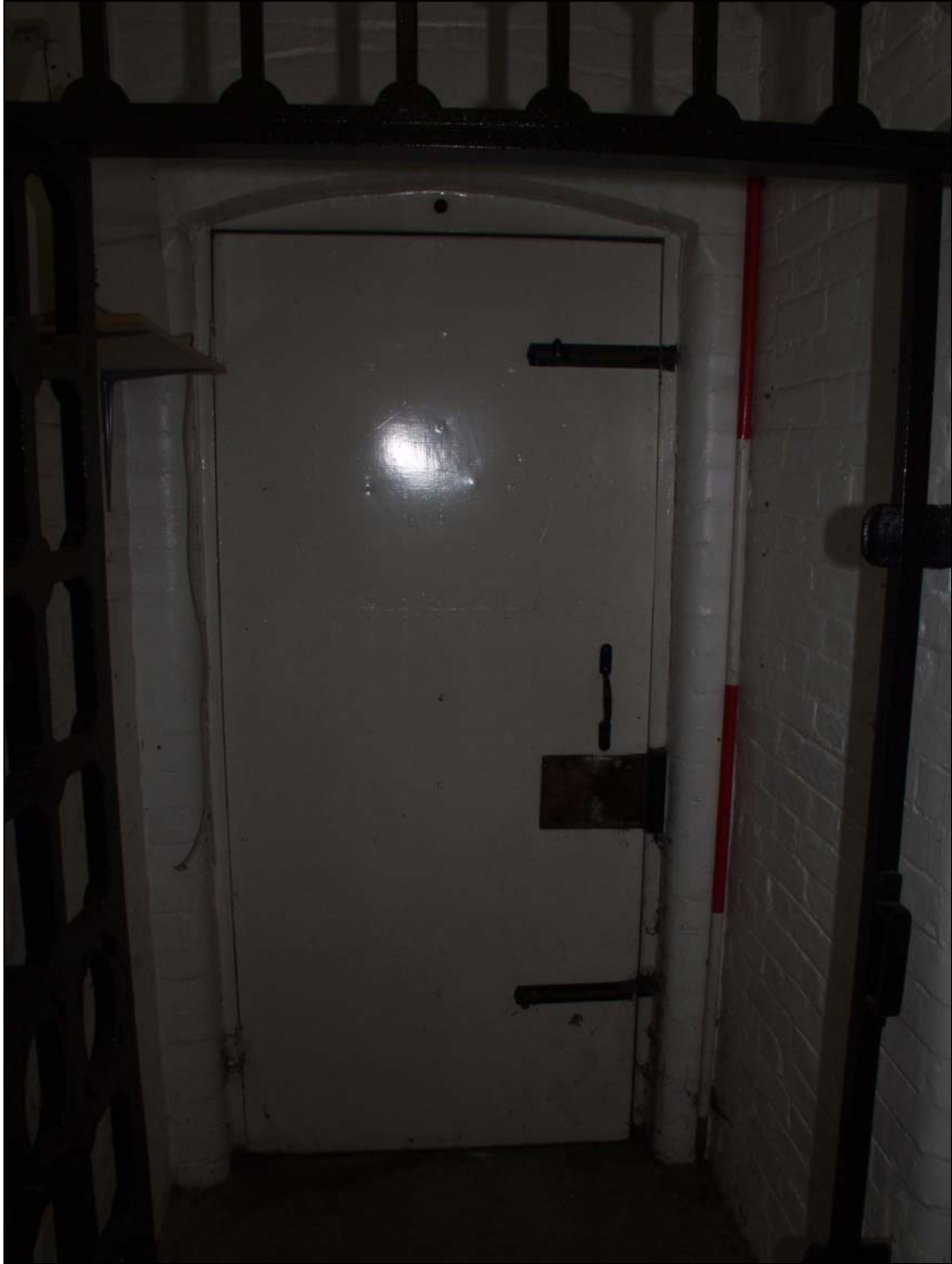
22 Metal plated door to rear yard at east end of principal corridor showing traces of former rim lock mechanism (29)
