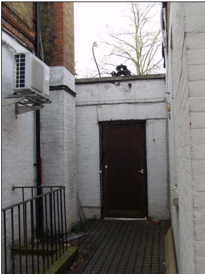
8 Rear of Portland stone door case from the east (7)
