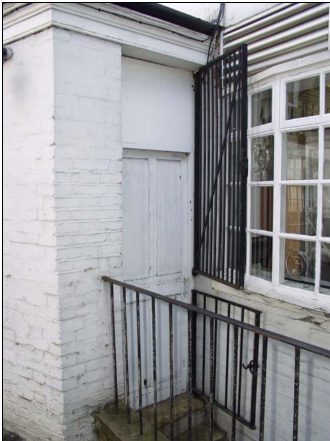
10 Iron gate protecting entrance to cellar from porch (22)
