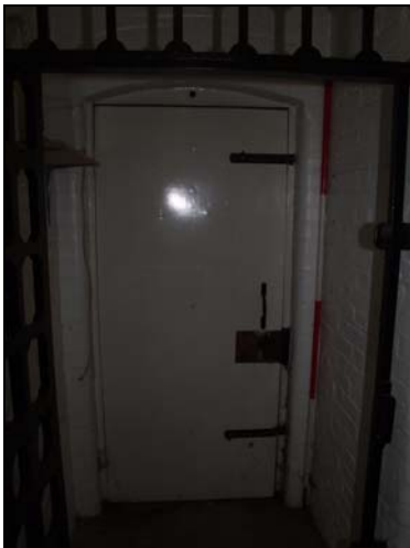
Pintle-hung, non-locking door to possible former lavatory
