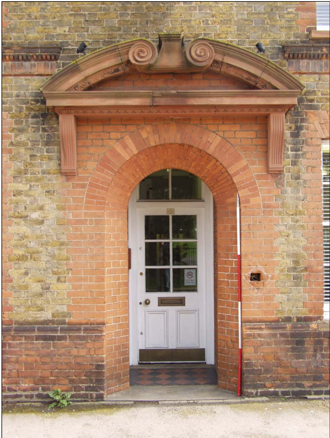
3 Principal doorway to domestic range (6)
