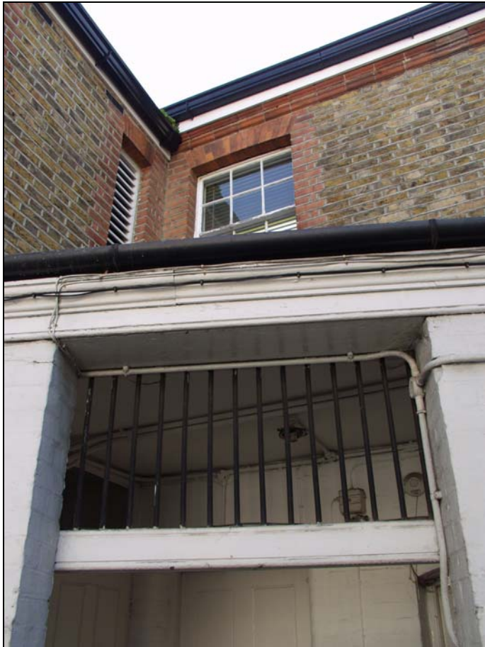
13 Cornice of porch in central yard (19)
