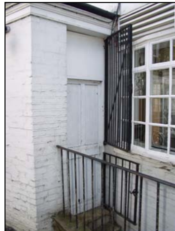
Fitting for former double doors in porch
