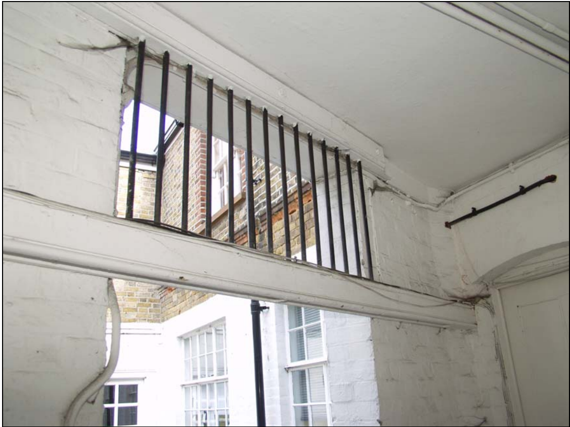
11 Fitting for former double doors in porch (20)
