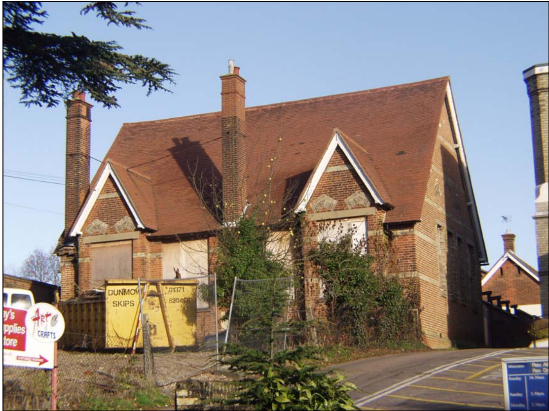
Plate 1 View of the assessment structure, taken from the south-east (14)
