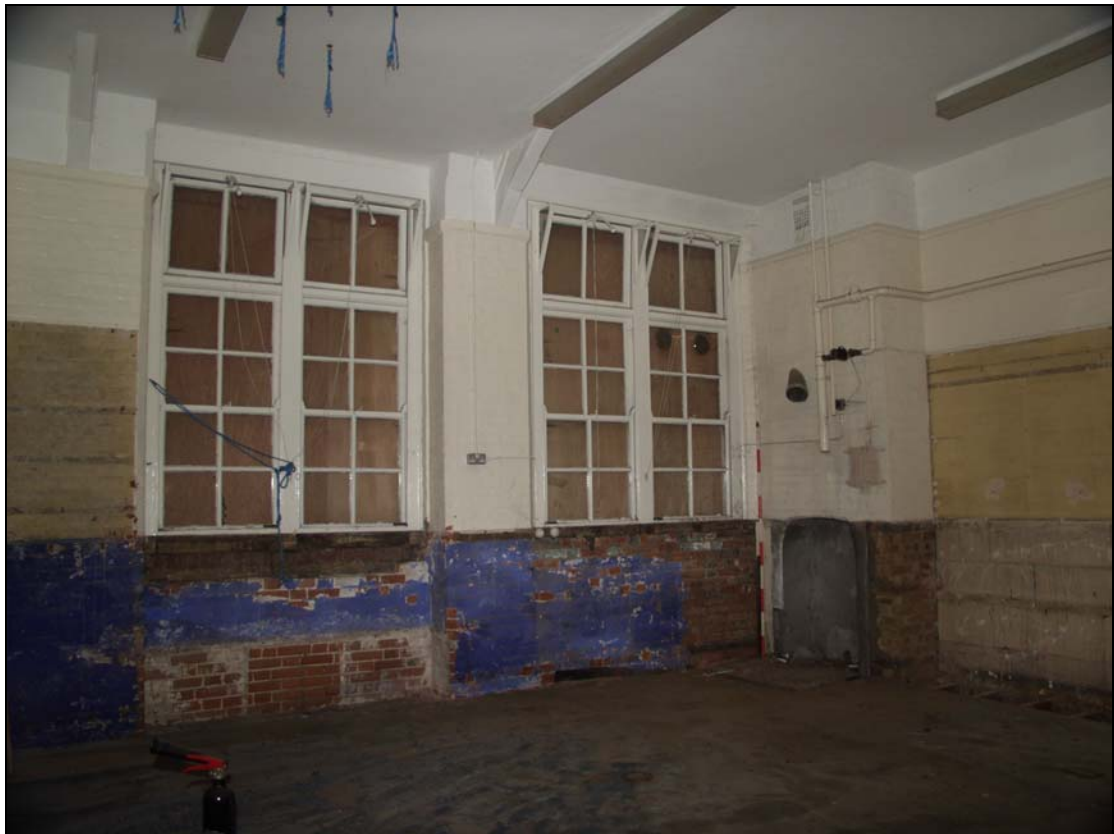
Plate 4 South wall of Room 1, taken from the north-east (22)
