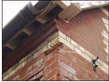
Brick banding on the rear range with typical Arleseey brick characteristics, taken from the north-east
