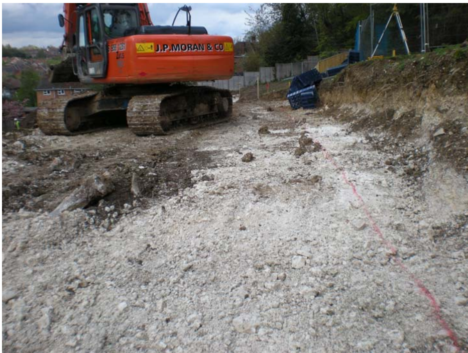
DP 2: South end of the area subject to monitoring, view N.
