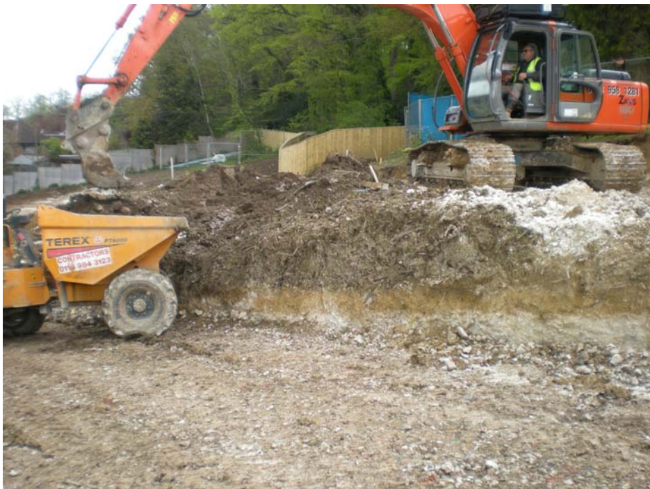
DP 4: Topsoil being removed from the area subject to monitoring, view N.
