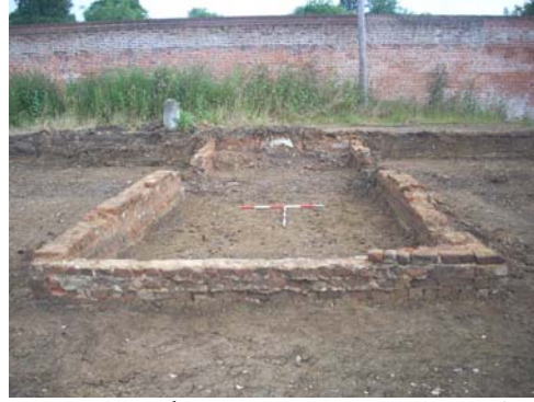
DP 14. Phase 3 Structure S2070, looking west.
