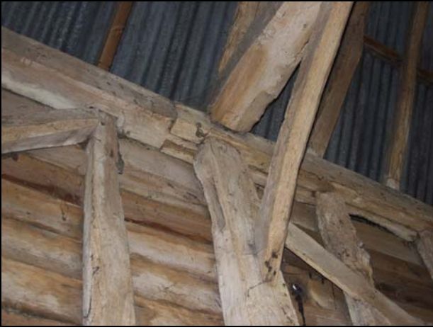
97 Carpentry joint on the north wall-plate of Building 2 (Bay 1), taken from the south
