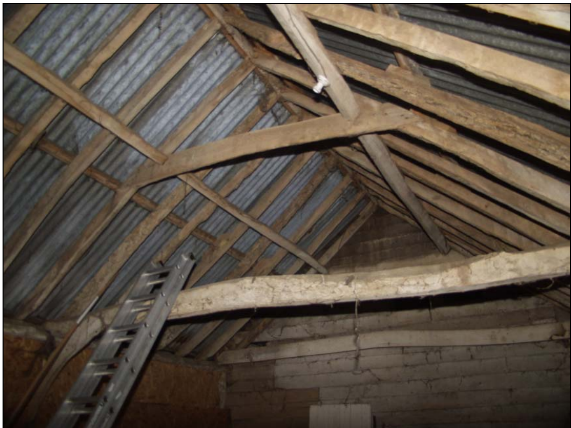
Plate 12 View of roof structure of Building 5, taken from the south-west (75)
