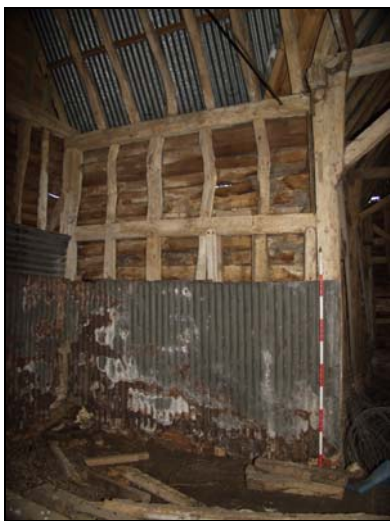
65 East wall of the porch (Building 2), taken from the west
