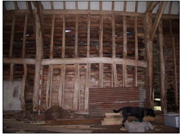
View of the south gable with former half-hip rafters surviving, taken from the north-east
