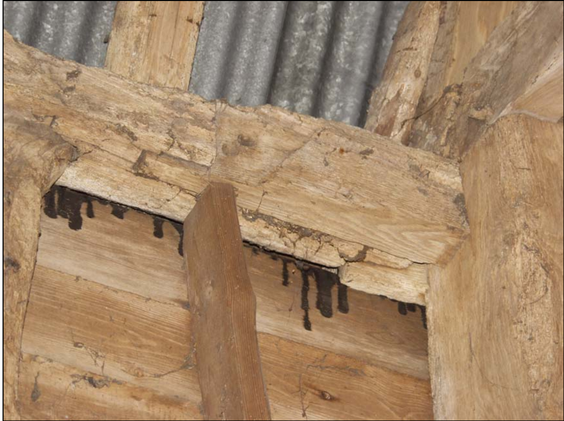
Plate 9 Face-halved and bladed scarf joint in the north wall-plate of Building 2 (Bay 4), taken from the south (96)
