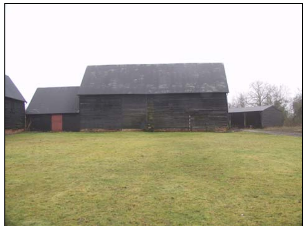
6 East range including Buildings 3 and 1, taken from the west
