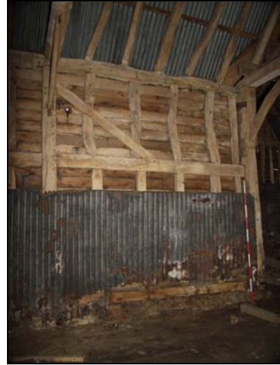
62 North wall of Bay 2 (Building 2), taken from the south
