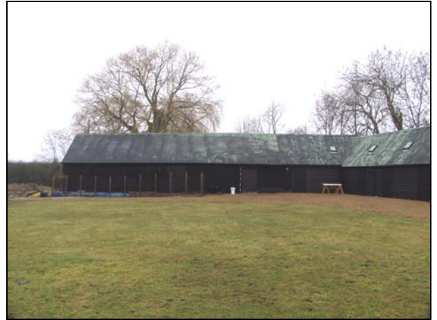
2 West range (Building 6) with residential unit on the right, taken from the east
