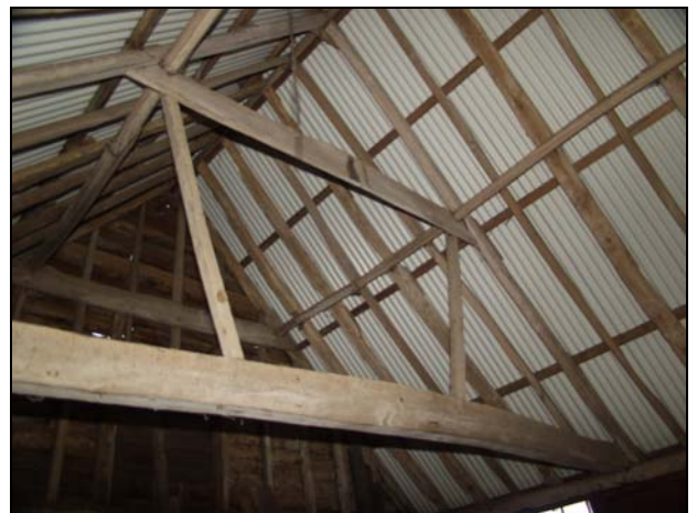
48 View of roof structure of Building 3, taken from the south-west
