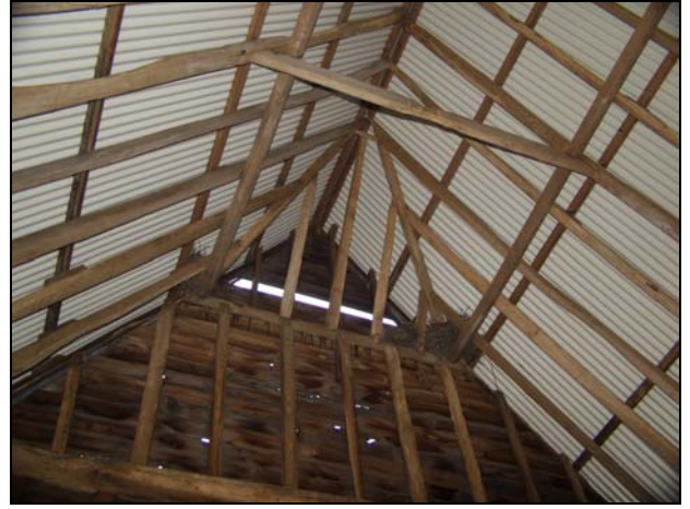
View of the south gable with former half-hip rafters surviving, taken from the north-east
