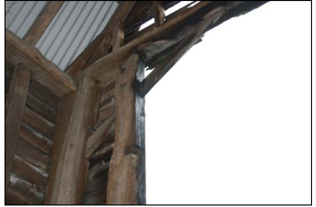
86 Detail view of brace threaded through the north doorjamb of the porch (Building 1), taken from the south-west
