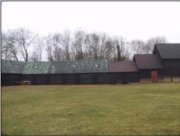
3 North range including residential unit on the left and Building 5 and 4 on the right, taken from the south
