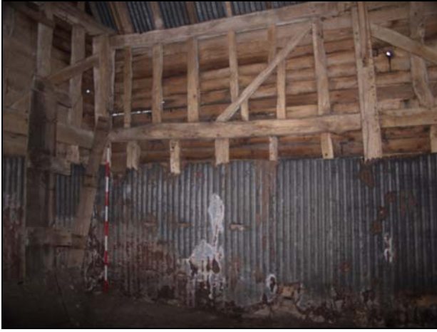
61 North wall of Bay 1 (Building 2), taken from the south
