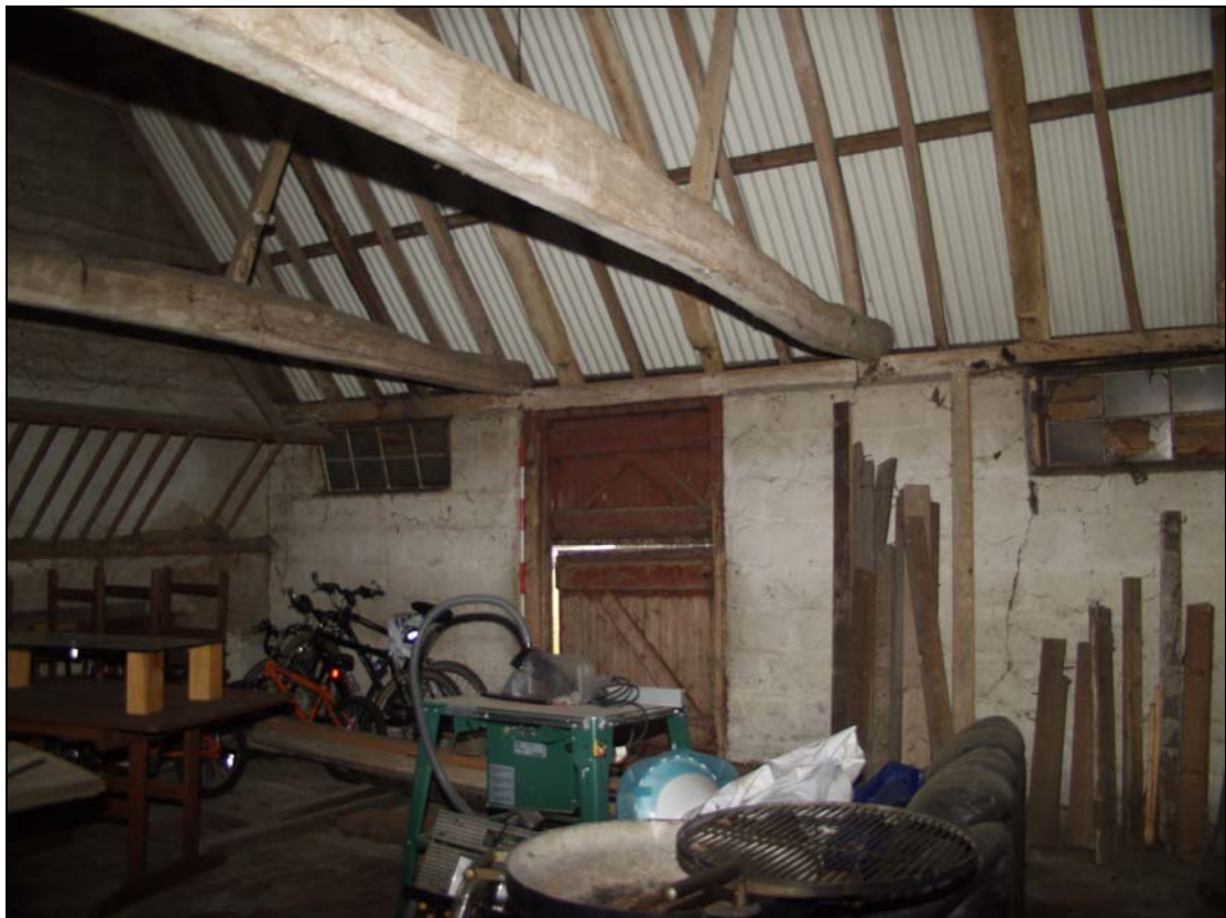
Plate 10 Interior of Building 3, taken from the north-east (46)
