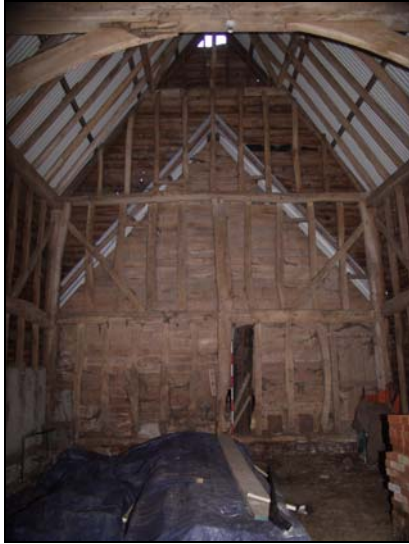
43 North wall of Building 1, taken from the south
