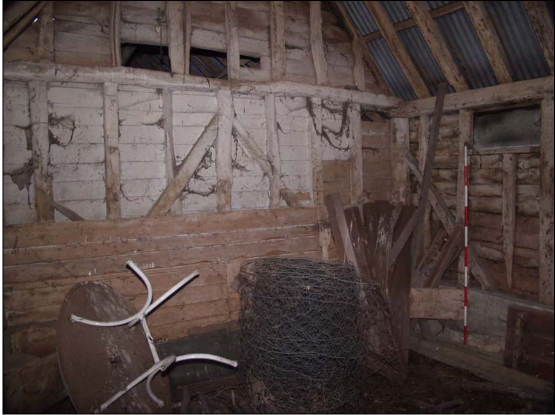
Plate 11 Interior of Building 4 showing west wall, taken from the east (72)
