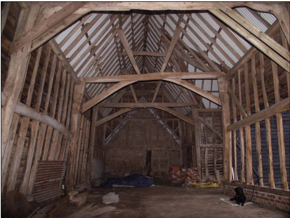
Plate 2 Interior of Building 1, taken from the south (25)
