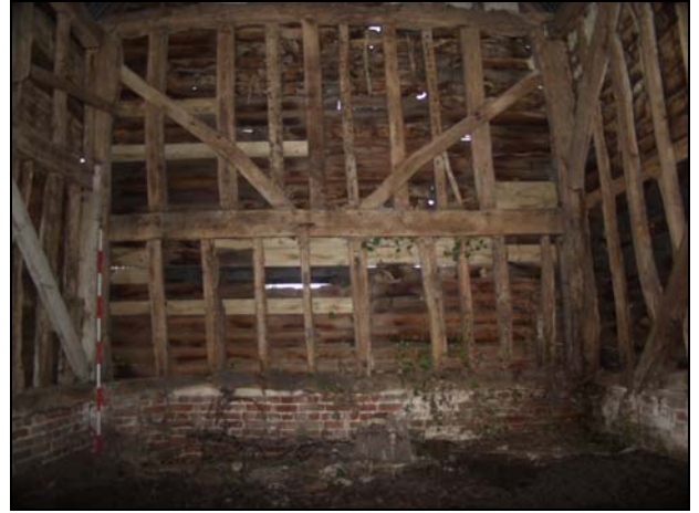
68 East wall of Building 2, taken from the west
