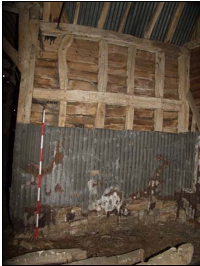
63 West wall of the porch (Building 2), taken from the east
