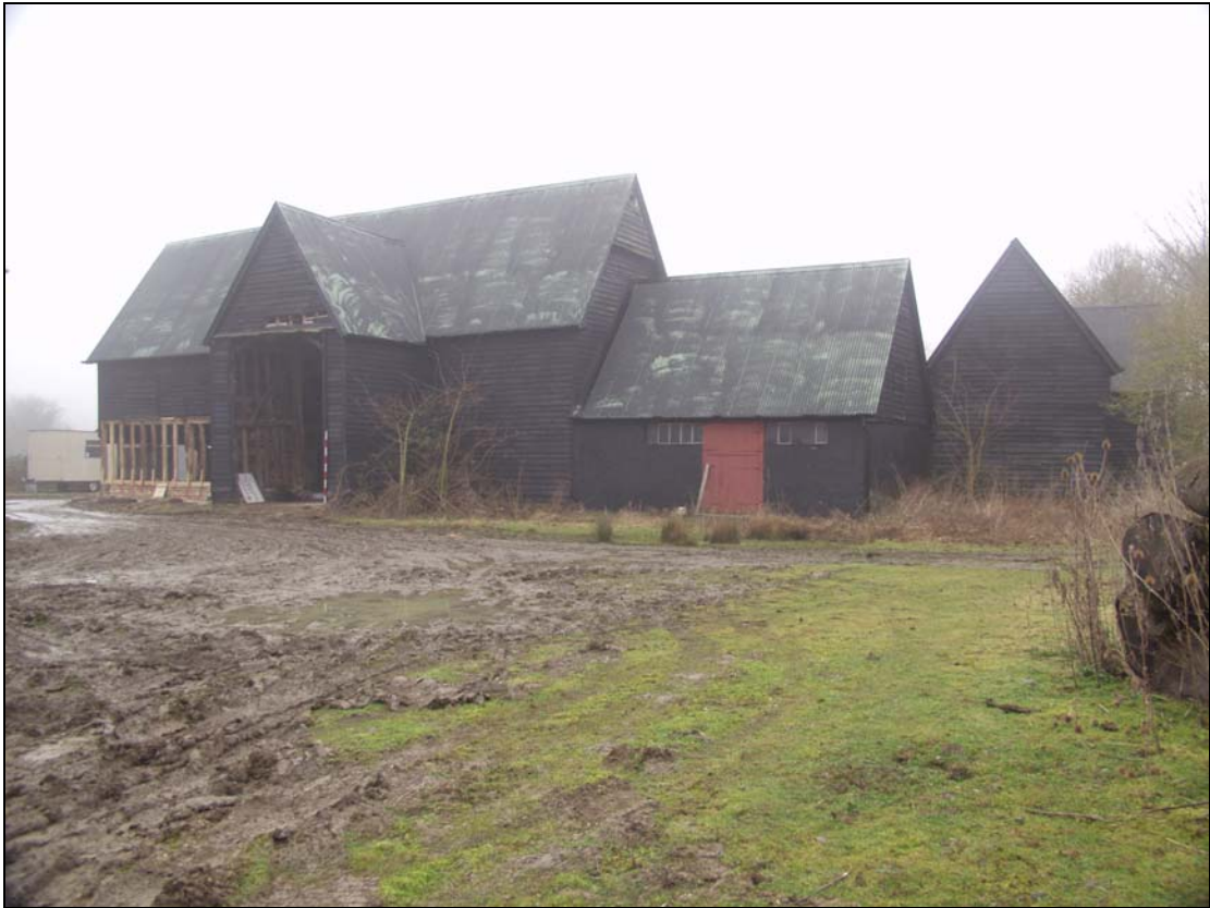
Plate 1 East elevation of Buildings 1 and 3, taken from the north-east (11)
