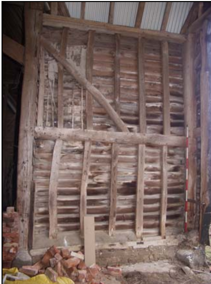
45 North wall of the porch (Building 1), taken from the south
