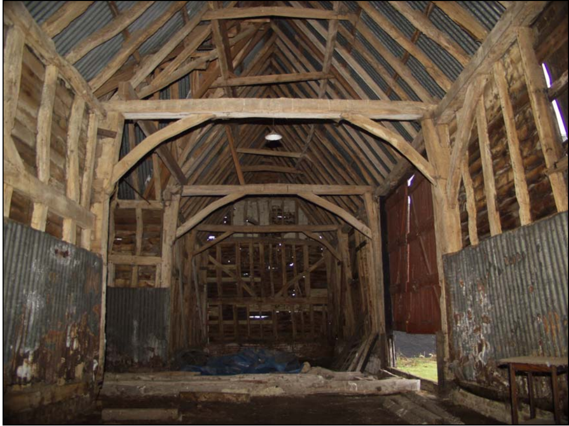
Plate 7 Interior of Building 2, taken from the west (49)
