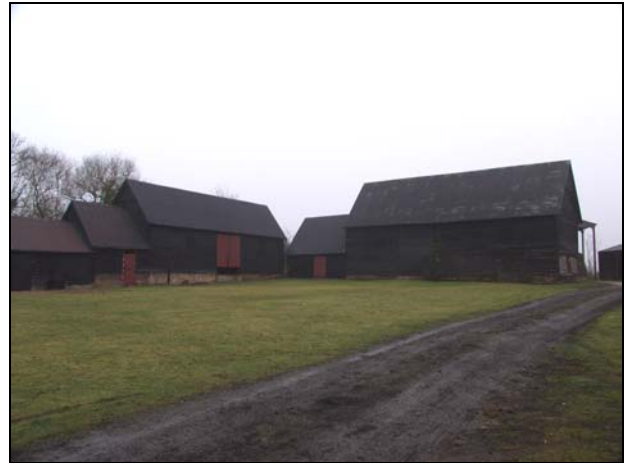
4 North range with Buildings 5, 4 and 2 and east range with Buildings 3 and 1, taken from the south-west
