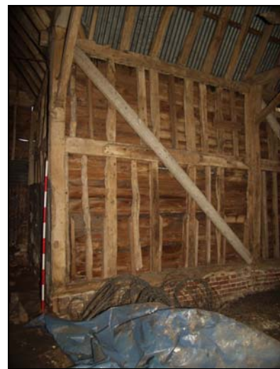
66 North wall of Bay 4 (Building 2), taken from the south
