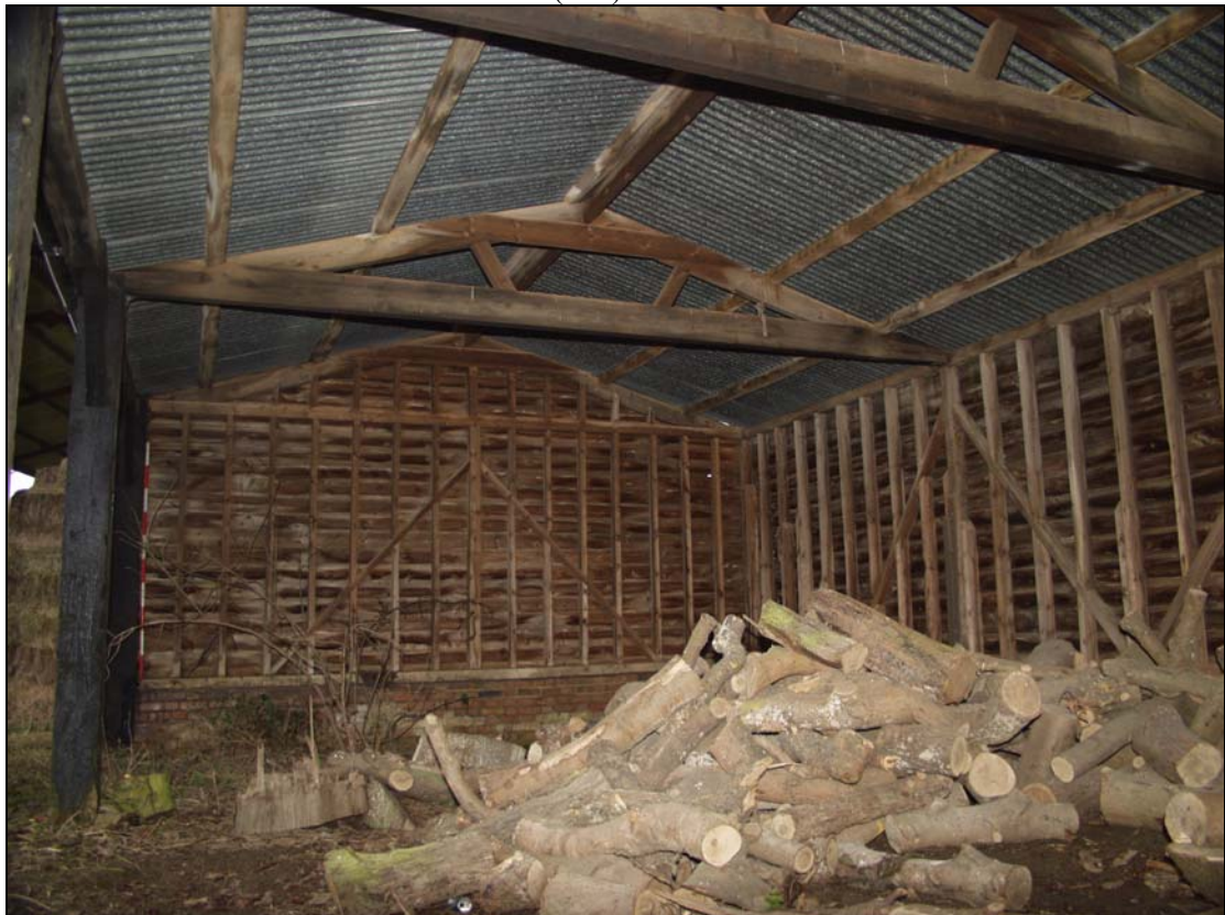
Plate 14 Interior of Building 7, taken from the west (82)
