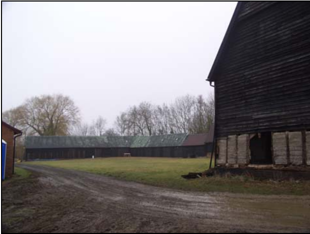
1 West and north ranges with Building 1 of the east range on the right, taken from the south
