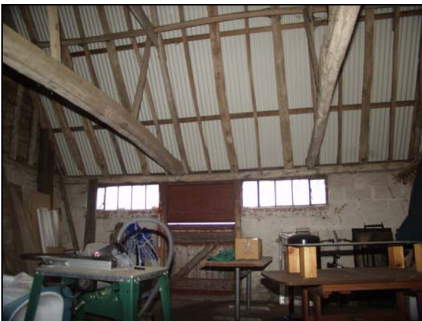
47 East wall of Building 3, taken from the west
