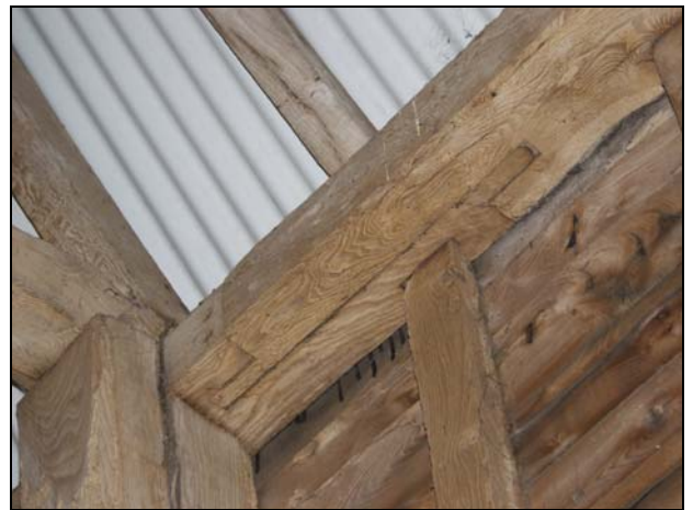
86 Detail view of brace threaded through the north doorjamb of the porch (Building 1), taken from the south-west
