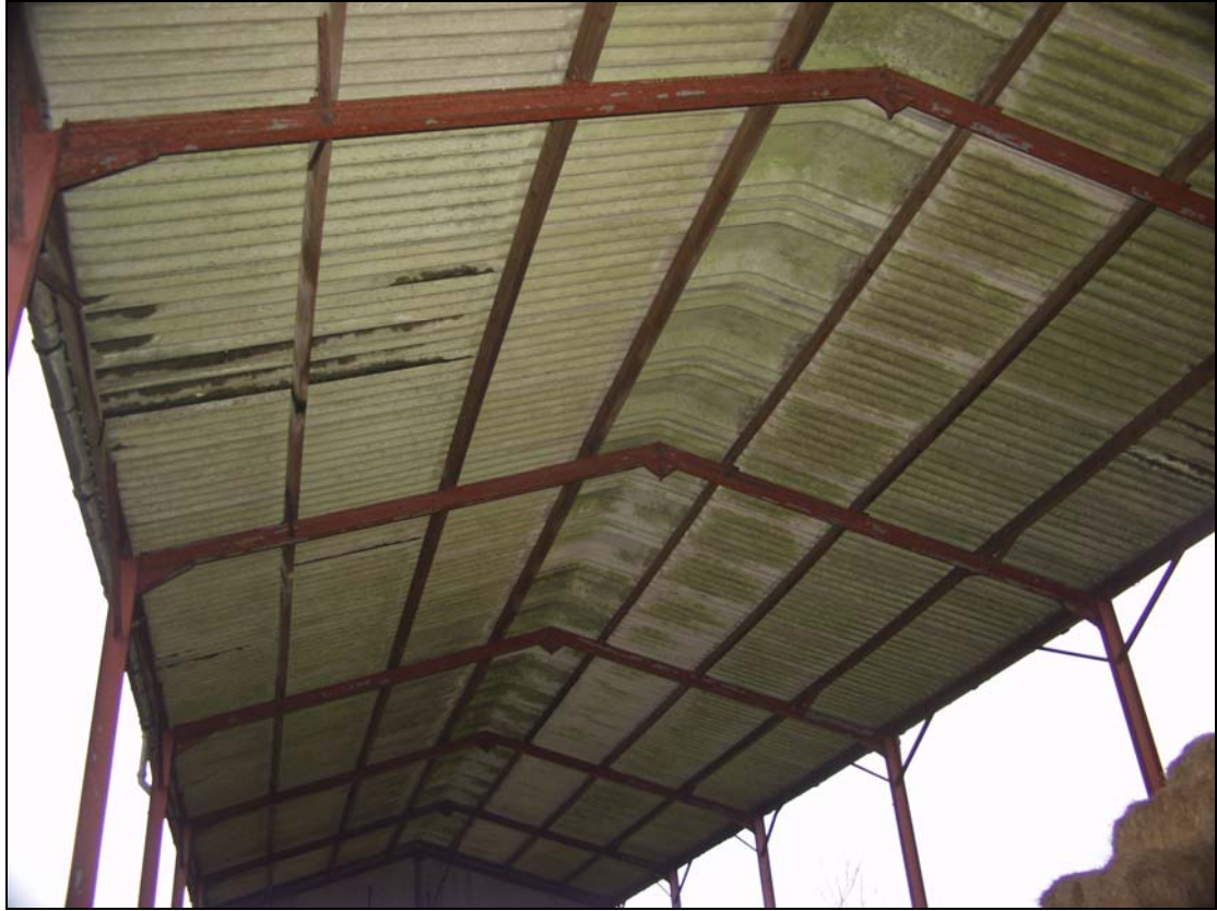
Plate 15 View of the roof structure of Building 8, taken from the west (84)
