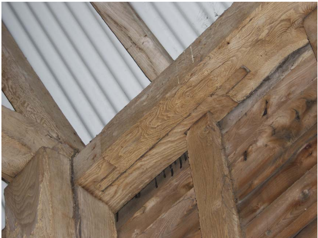
Plate 4 Face-halved and bladed scarf joint in west wall-plate of Building 1 (Bay 1), taken from the north-east (88)
