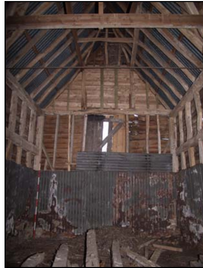
64 North wall of the porch (Building 2), taken from the south
