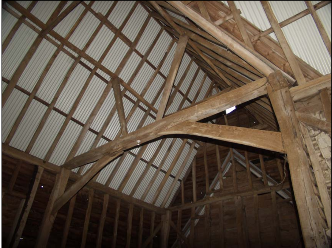
Plate 3 View of Truss 1 (Building 1), taken from the south-east (28)
