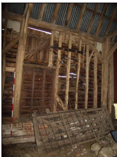
71 South wall of Bay 4 (Building 2), taken from the north
