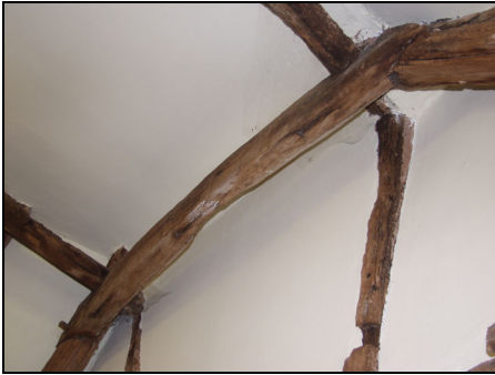
Redundant wattle slots on the south collar of Room 2 (extension), taken from the north-west
