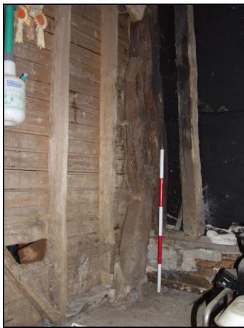
Scarf joint in the north sill-beam of the barn (Bay 5), taken from the south
