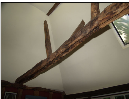
Detail of tie-beam in Room 1 showing groove and redundant mortices, taken from the north-east
