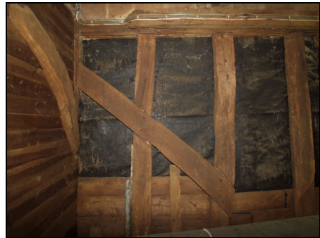
Redundant mortice on west door jamb of the barn, taken from the south
