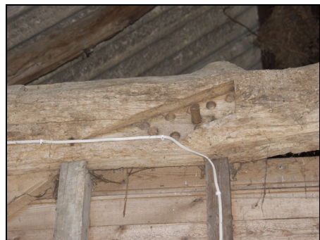
Scarf joint in the south sill-beam of the barn (Bay 4), taken from the north
