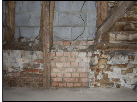
Detail of the dwarf wall of the west gable end of the barn, taken from the east
