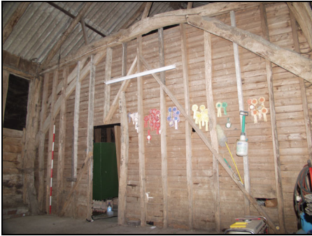
Studwork partition between Bays 4 and 5 in the barn, taken from the south-west
