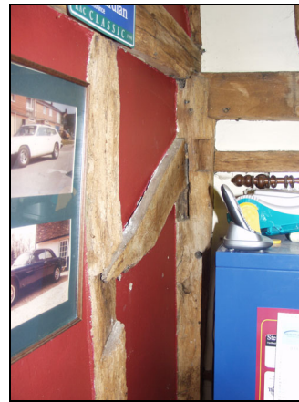
64 Detail of replaced brace on north wall of Room 2 (extension), taken from the south-west
