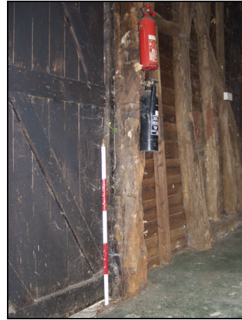
East door jamb of barn entrance showing mortices for locking bars and a threshing leap, taken from the south-west
