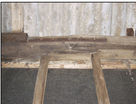
Detail of the north end of Truss 2 showing assembly marks, taken from the south-west
