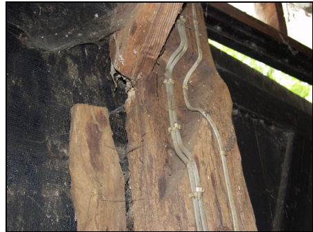
Redundant mortice on west door jamb of the barn, taken from the south
