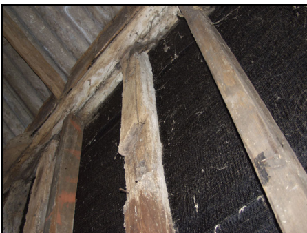
Cranked timber support to the south end of Truss 5 of the barn, taken from the north-west
