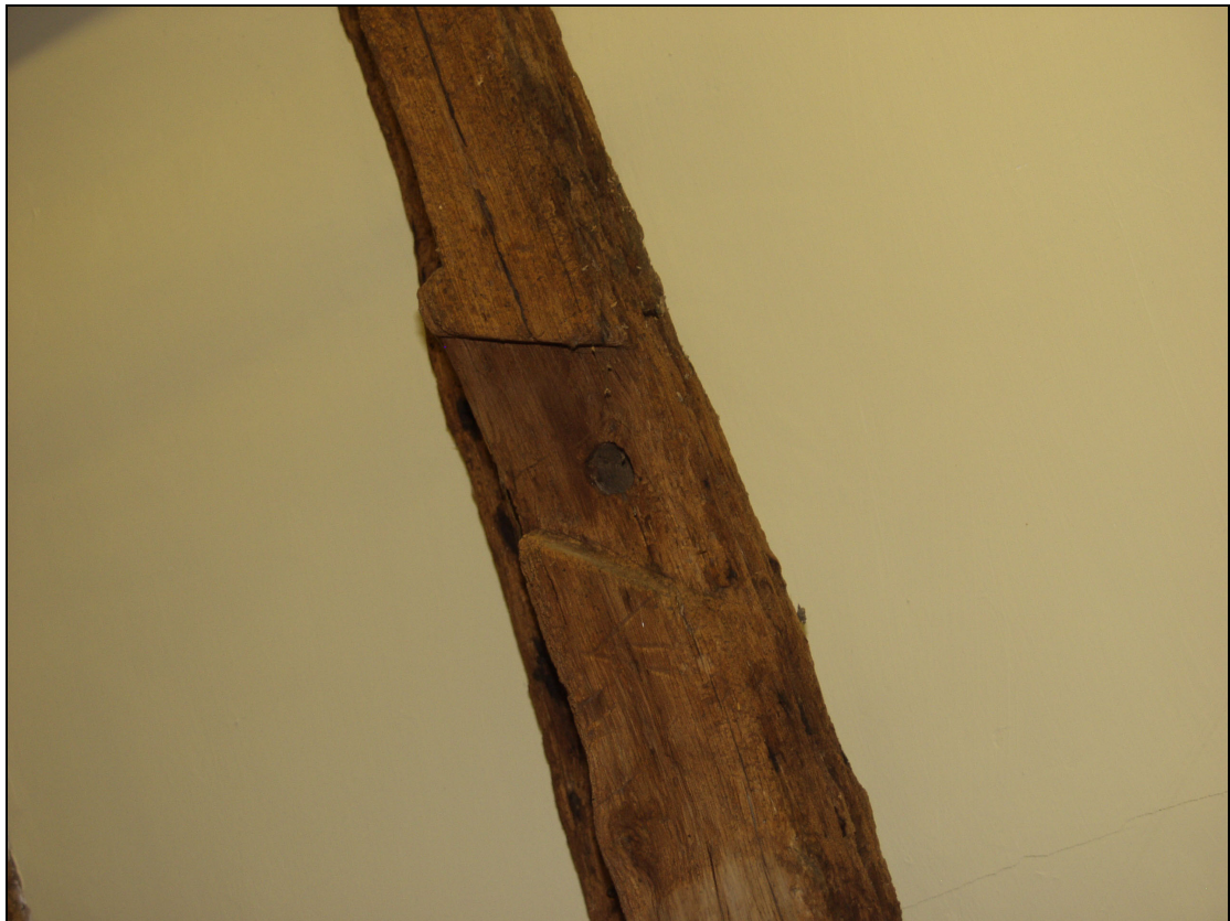
Plate 10 Redundant mortice and assembly mark on east subsidiary rafter in Room 2 (extension), taken from the west (65)
