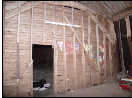
Studwork partition between Bays 4 and 5 in the barn, taken from the north-west
