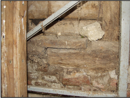
Scarf joint in the north sill-beam of the barn (Bay 5), taken from the south
