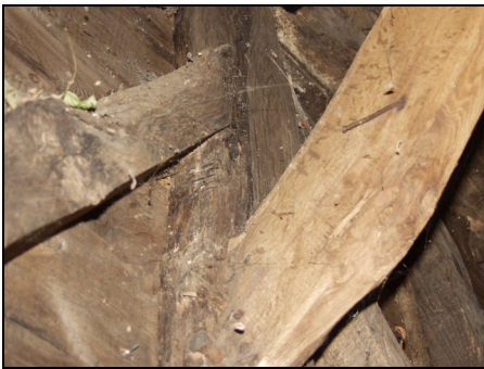
Detail of the north end of Truss 2 showing assembly marks, taken from the south-west
