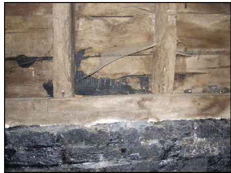
East door jamb of barn entrance showing mortices for locking bars and a threshing leap, taken from the south-west
