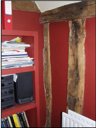
61 Redundant mortices on studs of the south wall of Room 1, taken from the north-west
