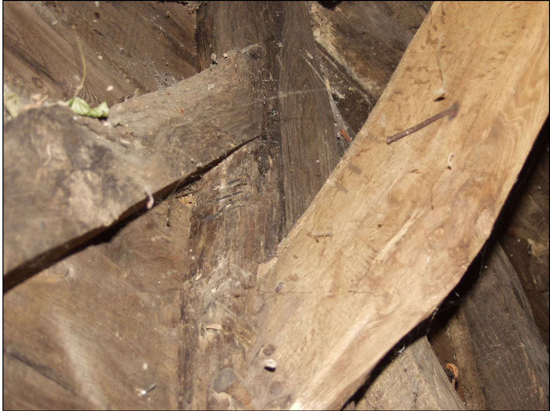
Plate 3 Detail of the north end of Truss 2 showing assembly marks, taken from the southwest (33)
