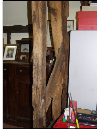
62 Brace on south wall of Room 2 (extension), taken from the north-east
