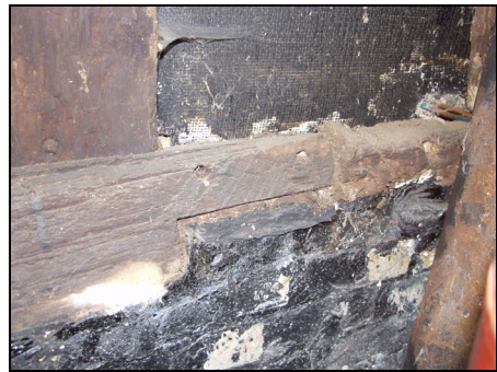
Scarf joint in the south sill-beam of the barn (Bay 4), taken from the north
