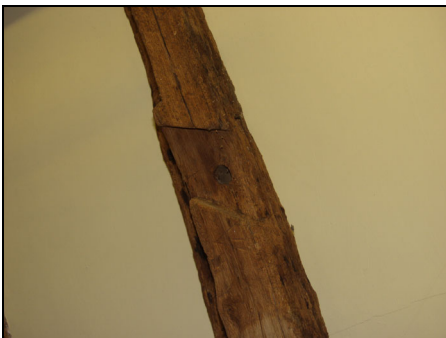
65 Redundant mortice and assembly mark on east subsidiary rafter in Room 2 (extension), taken from the west
