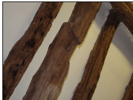
66 Redundant mortice and assembly mark on east subsidiary rafter in Room 2 (extension), taken from the north-west
