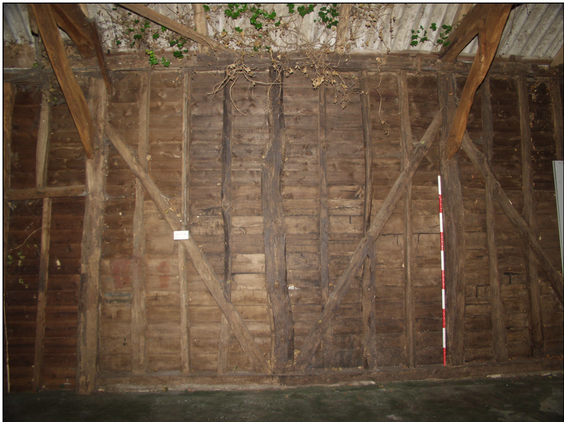
Plate 2 North wall of the barn (Bay 2), taken from the south (18)
