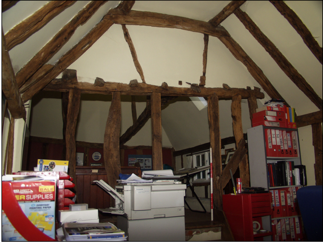
Plate 9 Open studwork of the south wall of Room 2 (extension), taken from the north (55)
