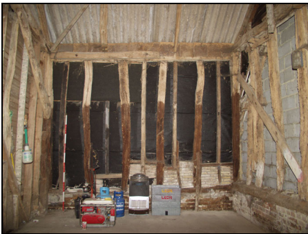
Studwork partition between Bays 4 and 5 in the barn, taken from the south-west
