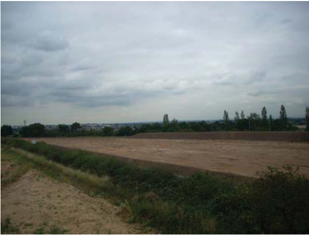
DP 3. General view – central and eastern part of the site. SE facing.
