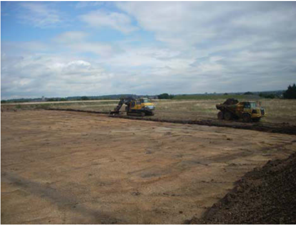
DP 1. Soil stripping. NE facing.
