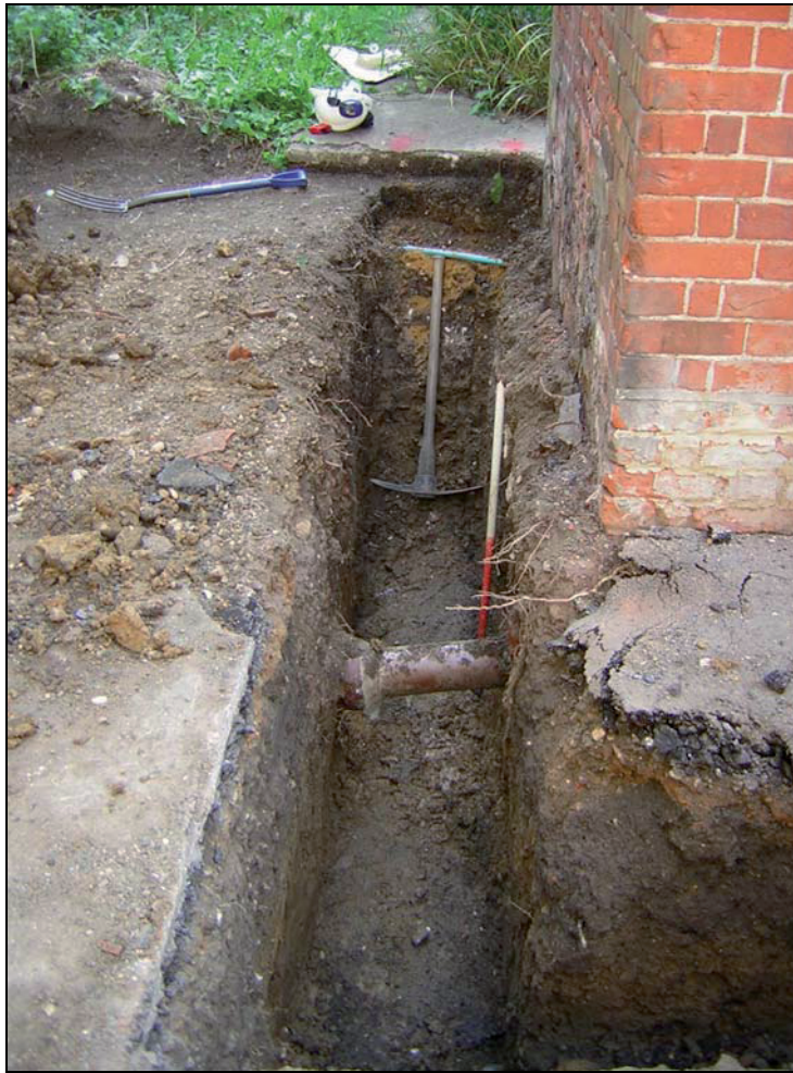
Plate 1 North-eastern section of foundation trench. View to the southeast.
