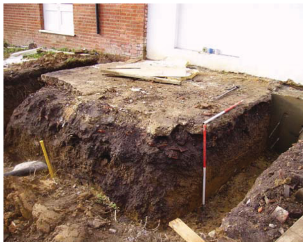
DP 2. Excavation of foundation trenches for new conservatory attached to farmhouse. Looking SW. Sample Section 8 visible on right-hand side.
