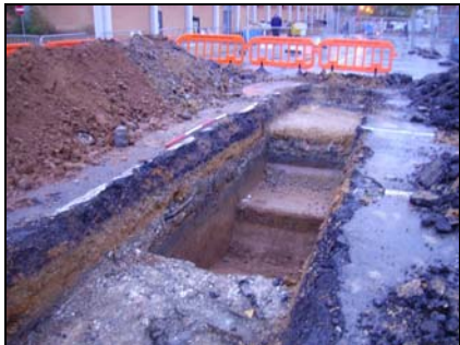
4 View of Trench 3 looking south east
