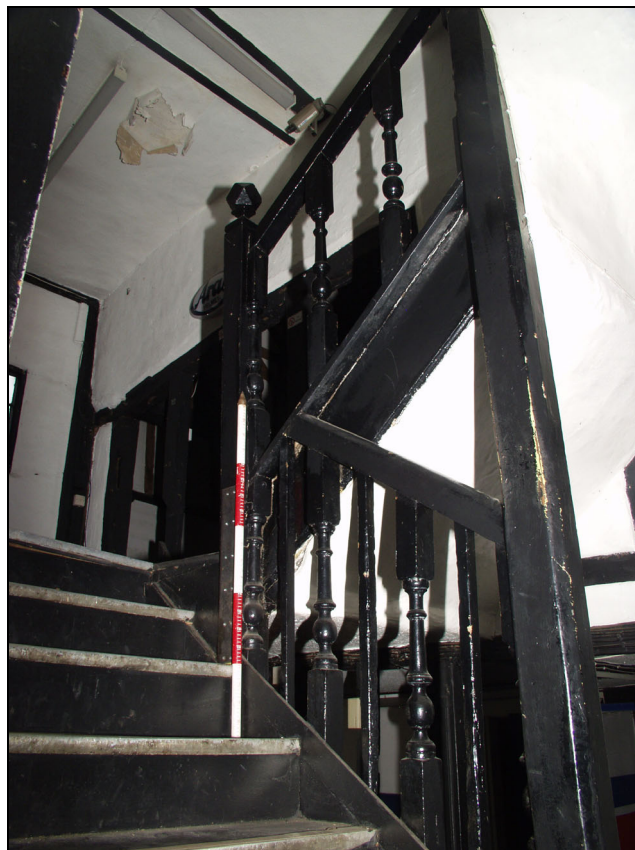
Plate 4 Detail of staircase, north range, taken from the north-west (26)
