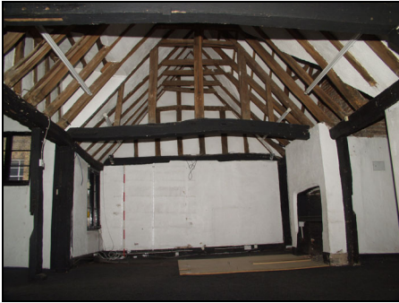
Detail of weathered crown-purlin in roof of the central range, taken from the north-east
