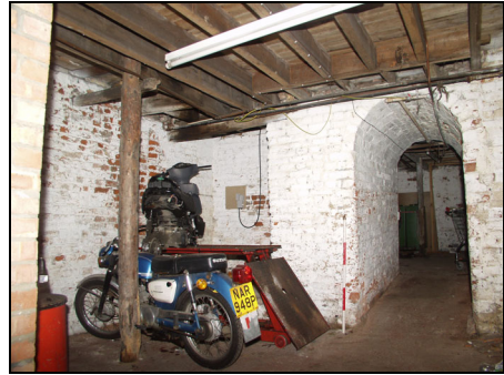
North area of the south range cellar, with arch supporting the chimneystack above, taken from the south
