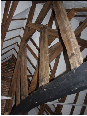
Detail of weathered crown-purlin in roof of the central range, taken from the north-east
