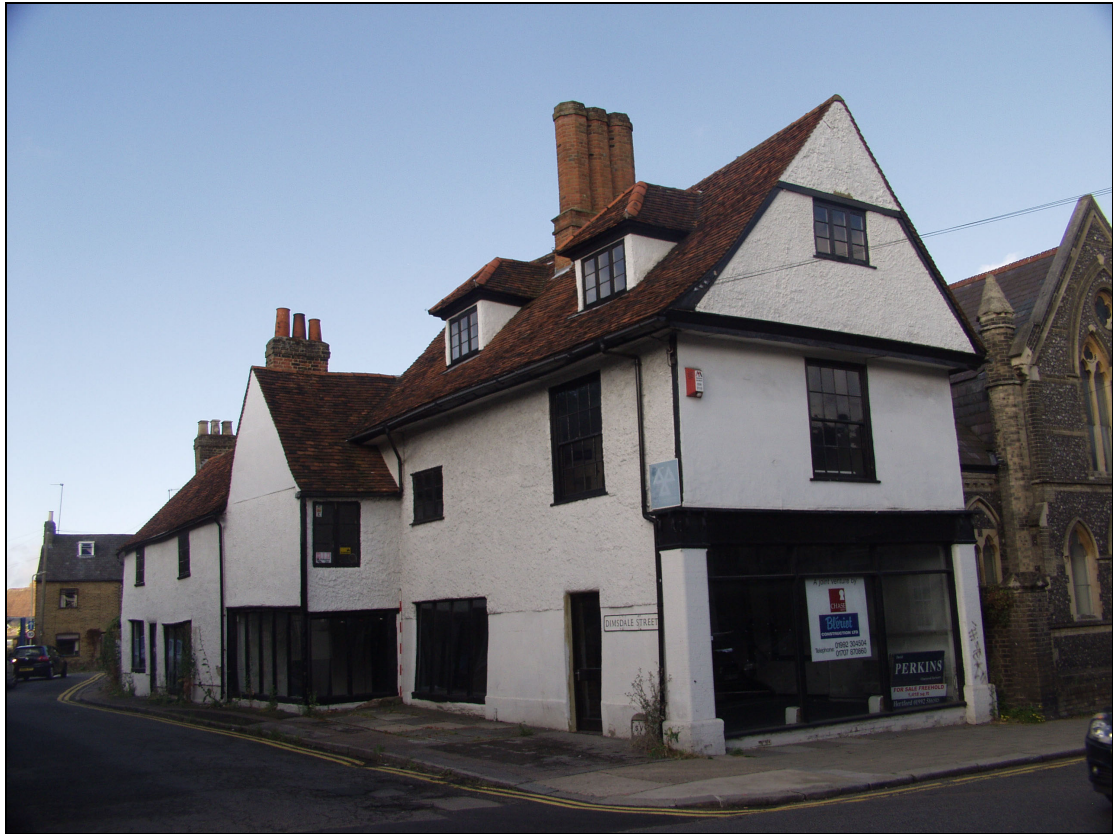
Plate 1 View of assessment building, taken from the north-east (6)
