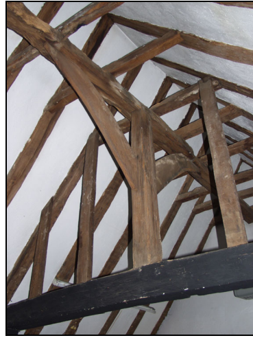
Detail of crown-post in roof of the central range, taken from the north-east
