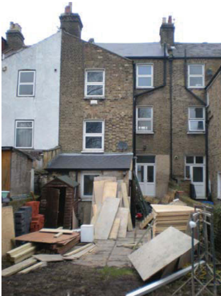
DP 3. View to the rear of the house. Taken from SSE.
