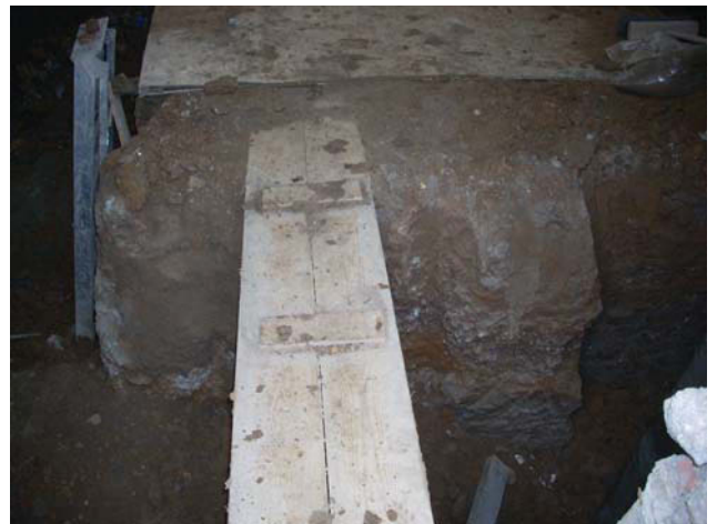
DP 6. N part of the basement. Taken from NNW.
