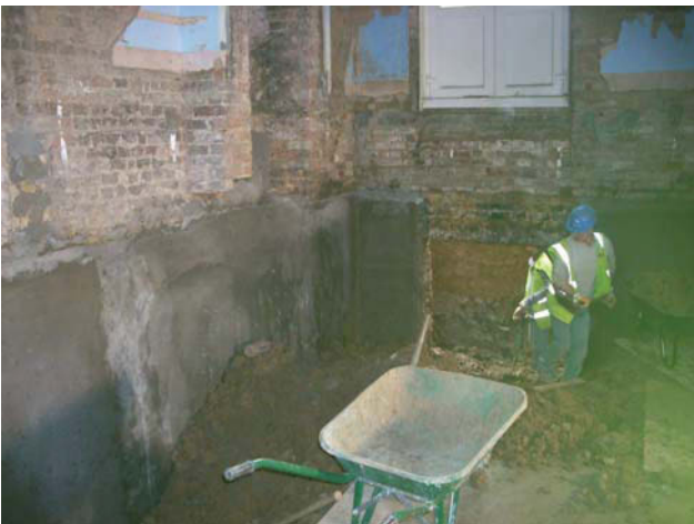
DP 5. Ground works inside the basement. Taken from NW.
