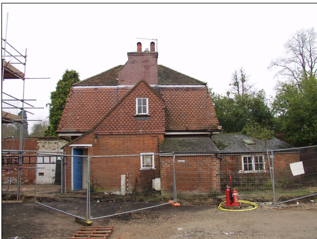
2 East elevation of Lime Cottage, taken from the east (3)
