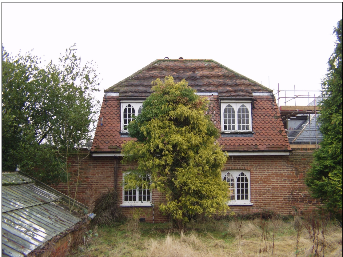
4 West elevation of Lime Cottage, taken from the west (6)
