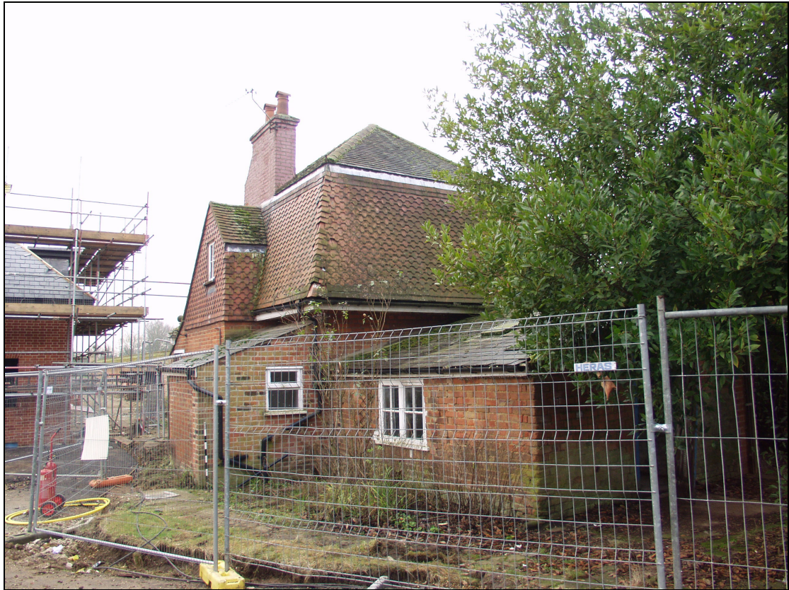
3 East elevation of Lime Cottage, taken from the north-east (5)
