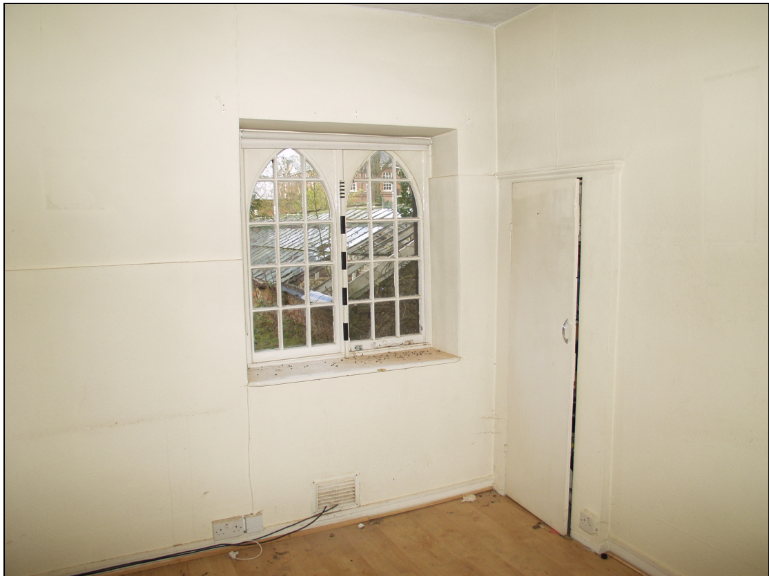
5 Ground floor living room in Lime Cottage, taken from the south-east (12)
