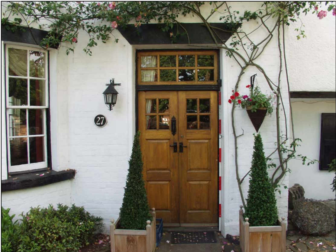
8 Entrance to 1830s wing, taken from the east (47)
