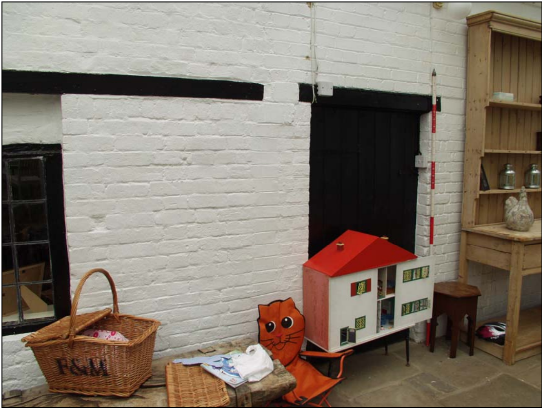
7 Doorway between barn and conservatory, taken from the north-west (13)
