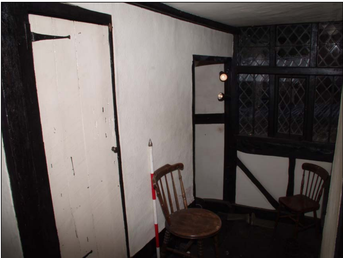
16 Cupboard door on landing in stair-turret, taken from the south-east (45)
