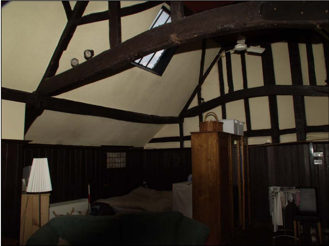
21 View of barn, looking into west extension, taken from the south-east (27)
