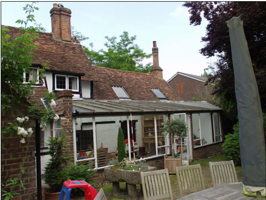
6 View of the conservatory, taken from the north-west (12)
