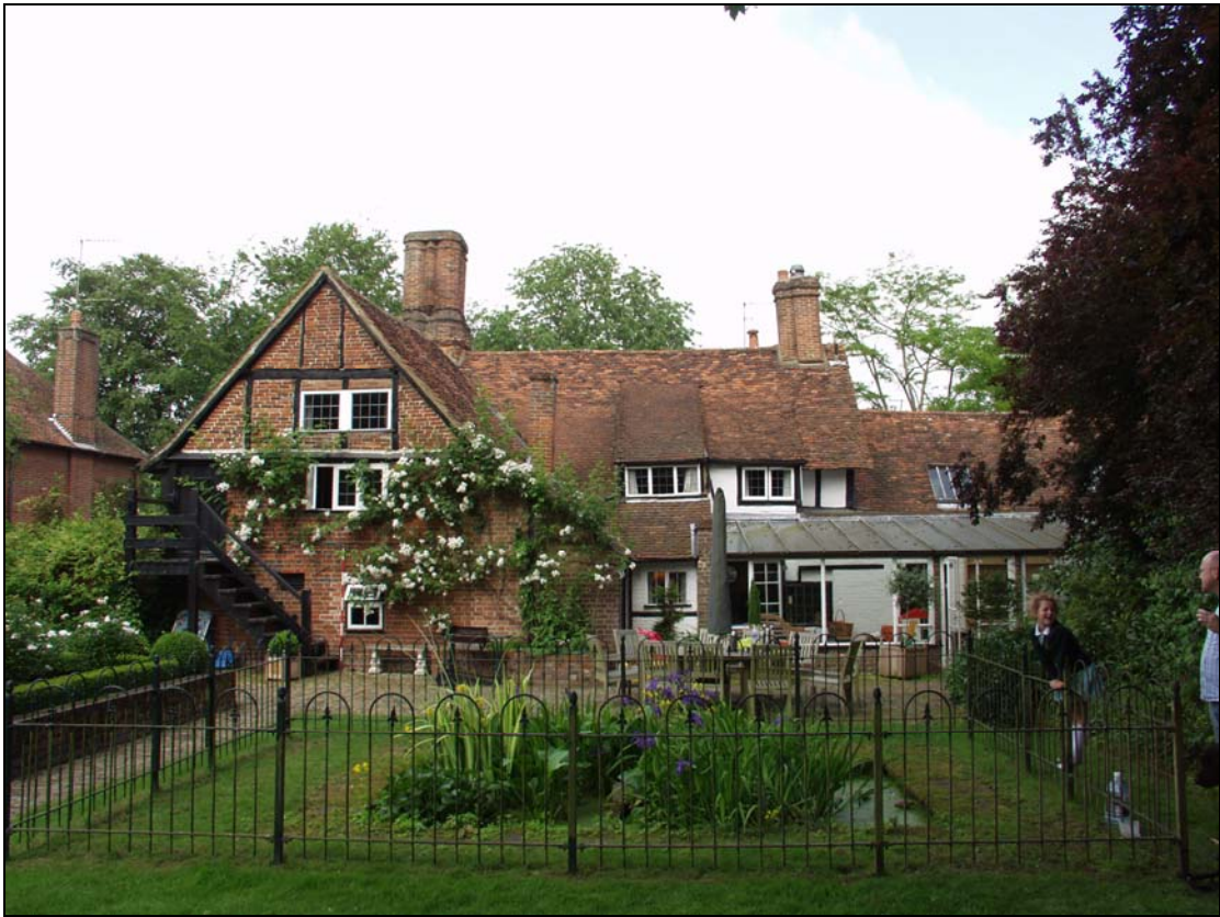
5 West elevation of the building, taken from the west (11)
