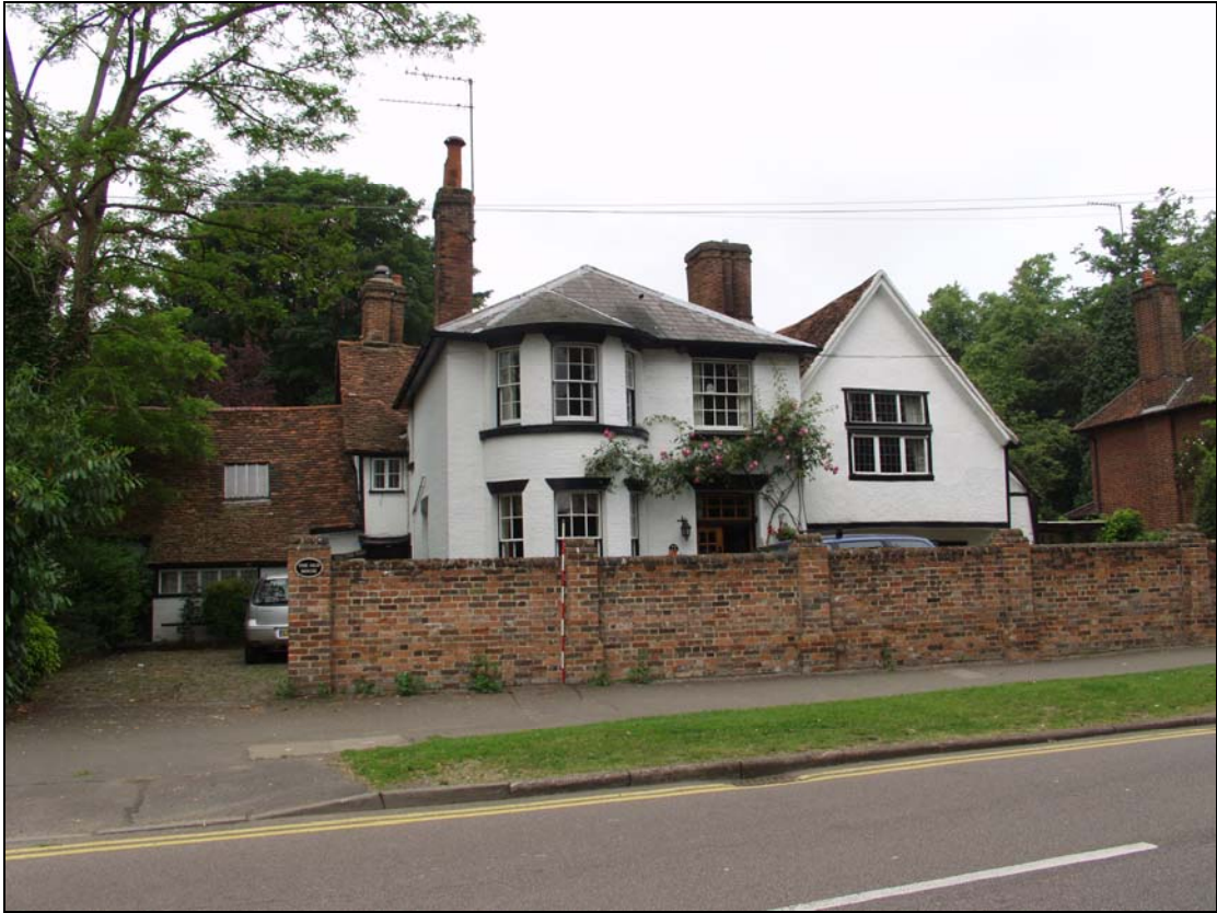
1 East elevation of the building, taken from the east (2)
