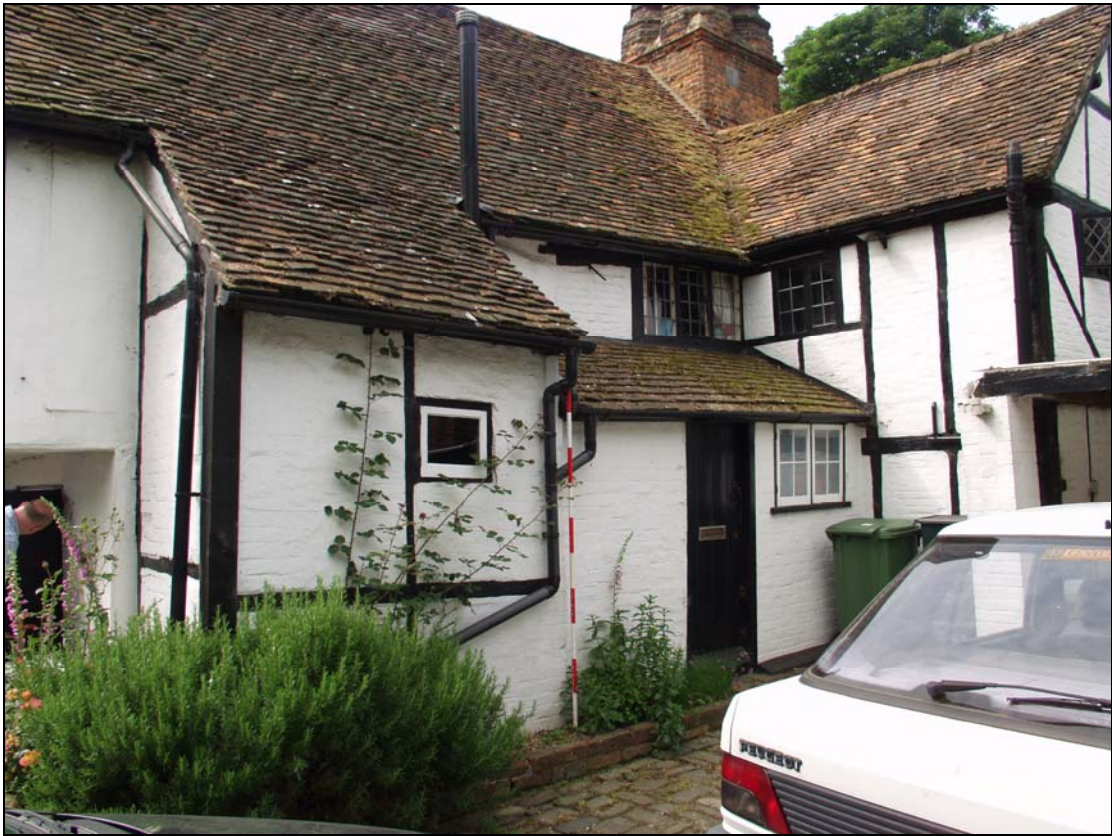
19 Outshuts to north of 16 th century range, taken from the north-east (6)
