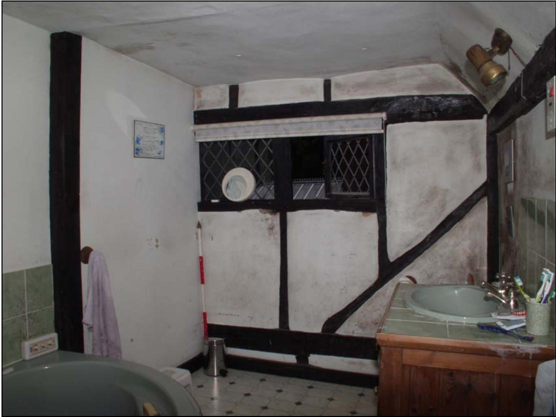
17 Bathroom on first floor of stair-turret, taken from the south (34)
