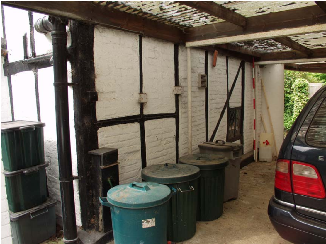
4 Lower part of north wall of stair-turret, taken from the north-east (7)
