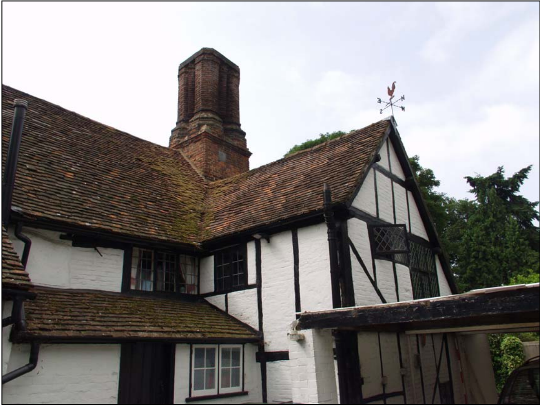
3 Stair-turret and chimney stack, taken from the north-east (8)
