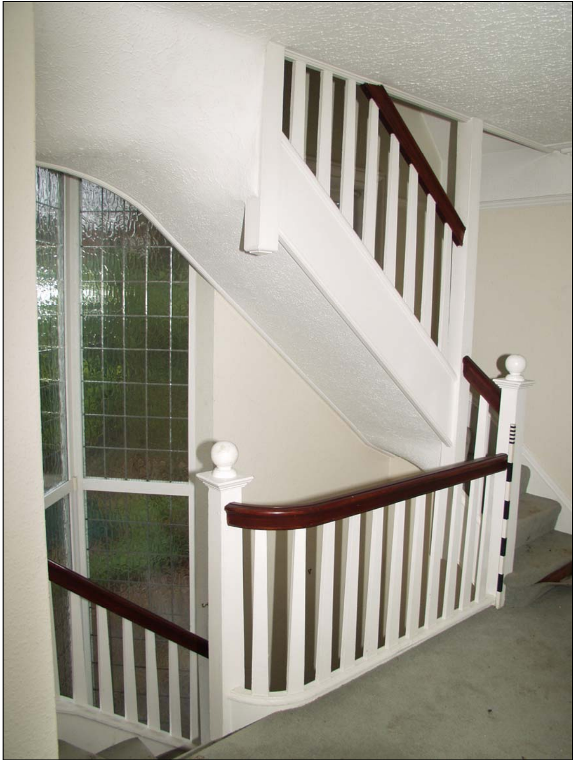
7 First floor landing and staircase, taken from the west (13)
