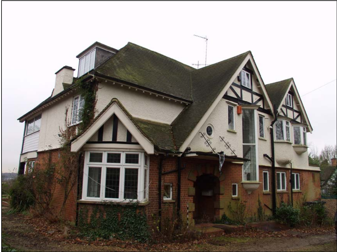
1 North-east and south-east elevations, taken from the east (1)
