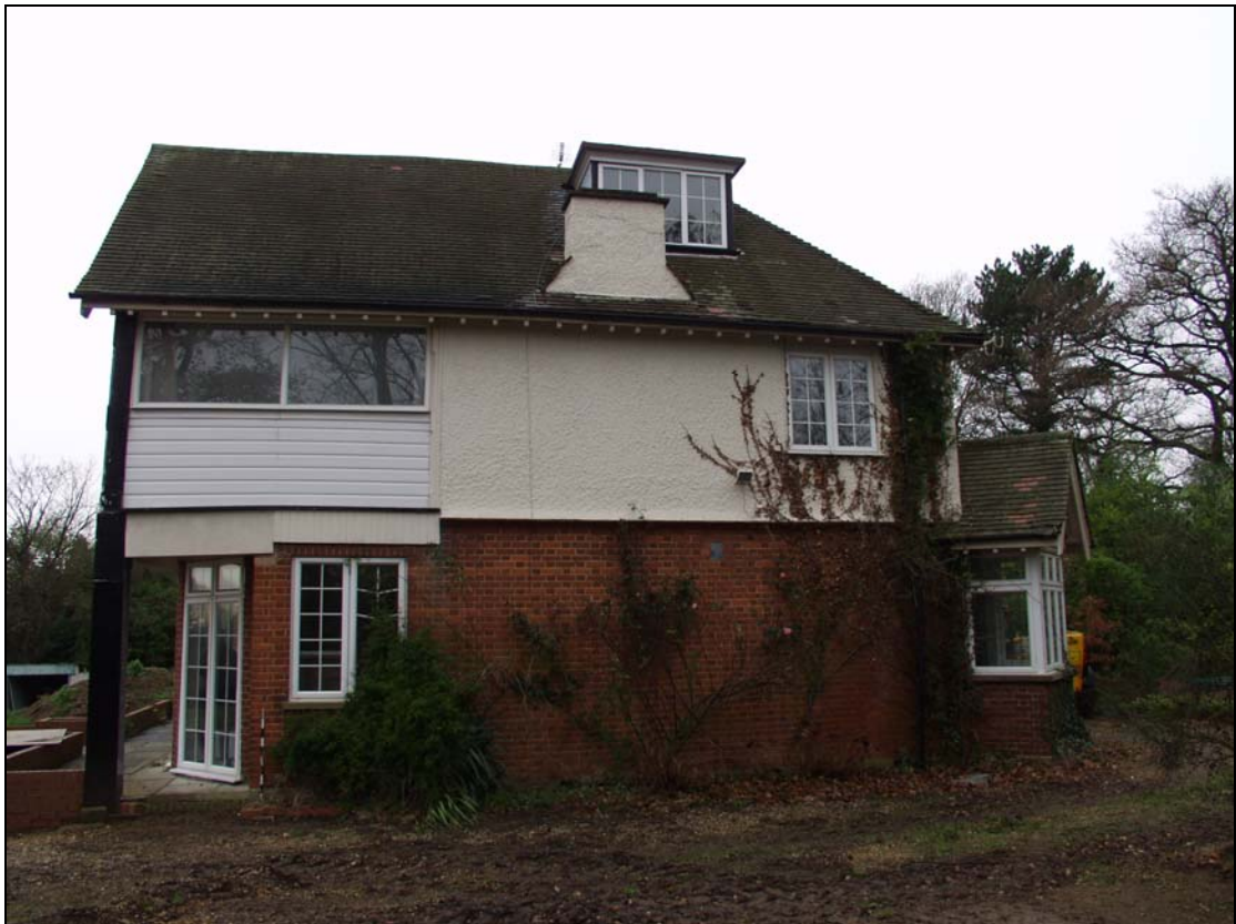
4 South-east elevation, taken from the south-east (5)
