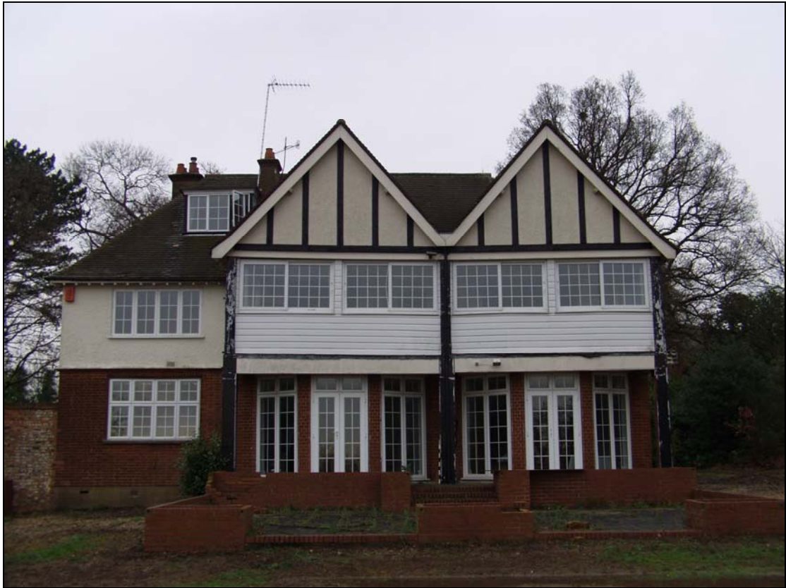
3 South-west elevation, taken from the south-west (4)
