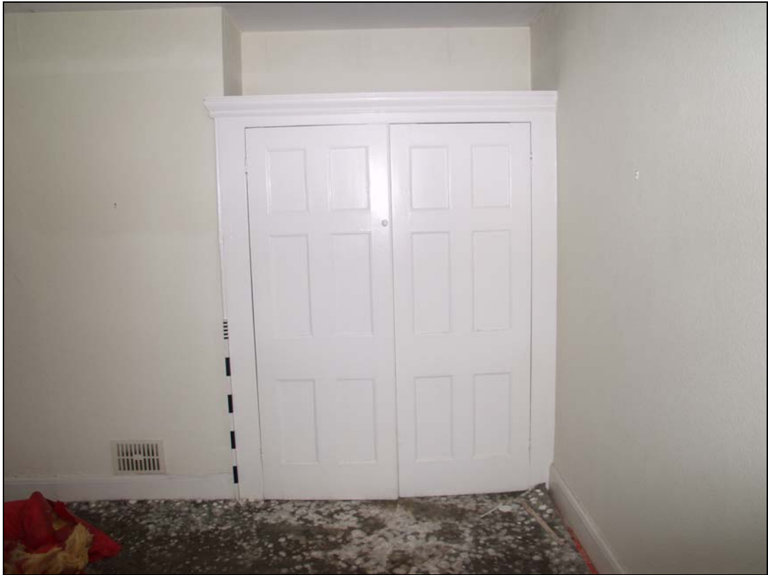
8 Detail of built-in cupboard to bedroom four, taken from the north-east (19)
