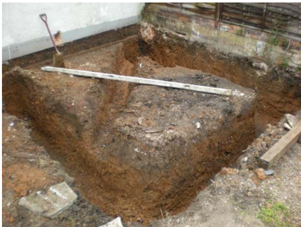
DP 38 General view of groundworks. Looking SW.
