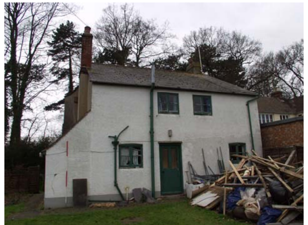
DP 39 Hillside cottage. View of the rear of the building before groundworks commence.
