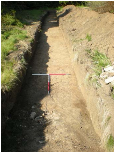
DP 15. Trench 3. Taken from NE.
