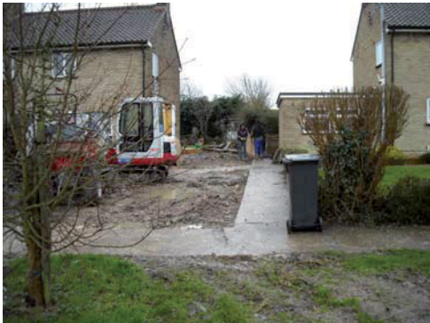
DP1. Site. From NW.
