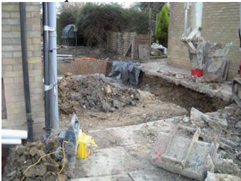
DP5. Foundation Trench. From N.
