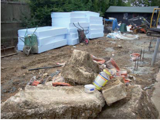
1 General Site Shot, view south-east.
