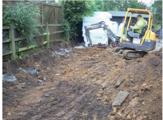
2 General site shot, view south-east.
