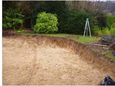
DP 2 Monitored Area, view north
