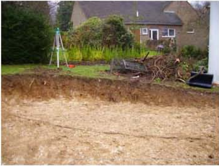
DP 1 Monitored Area, view east
