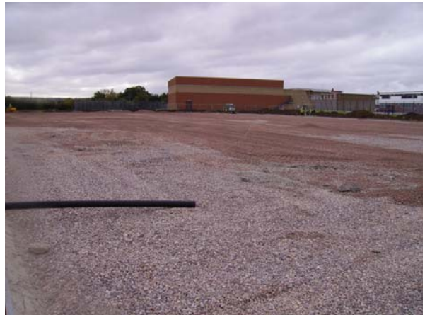
DP 4 Completed construction pre-final surfaces facing south
