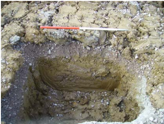
DP 3 Floodlight base 1 facing north west
