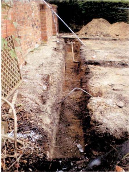
1 Northernmost trench of footings looking east
