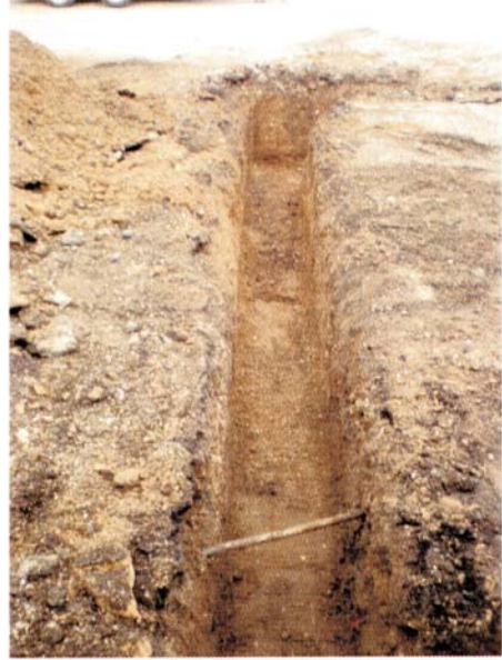
2 Westernmost trench of footings looking south
