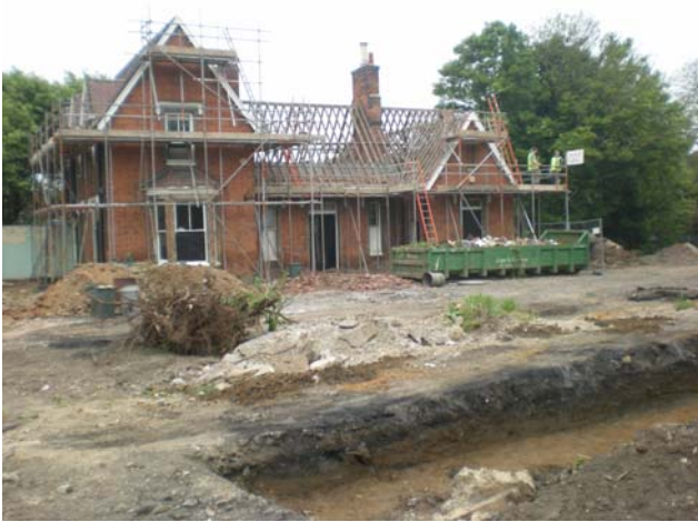
DP 1. Station House, Aspenden Road, Buntingford. Taken from E.
