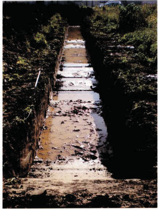
DP 6. Post excavation, Trench 2, view S
