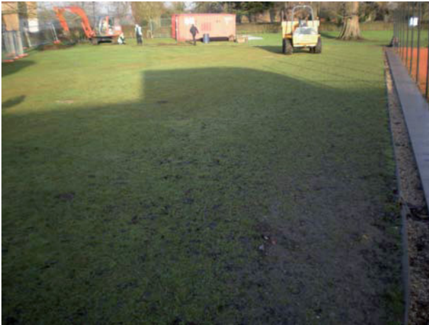
DP1 Area of new tennis court prior to works
