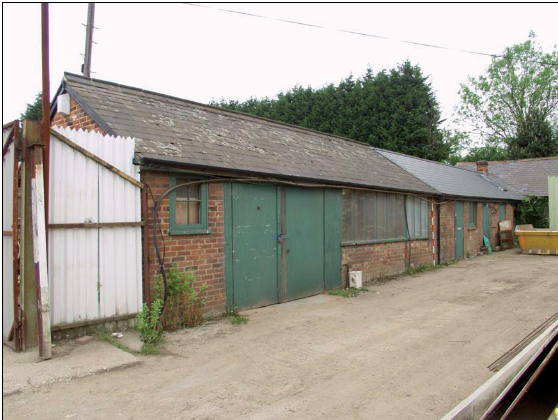
6 East elevation of Building 2, taken from the south-east (6)
