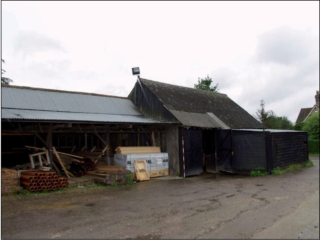
17 West elevation of Building 4, taken from the north-west (41)
