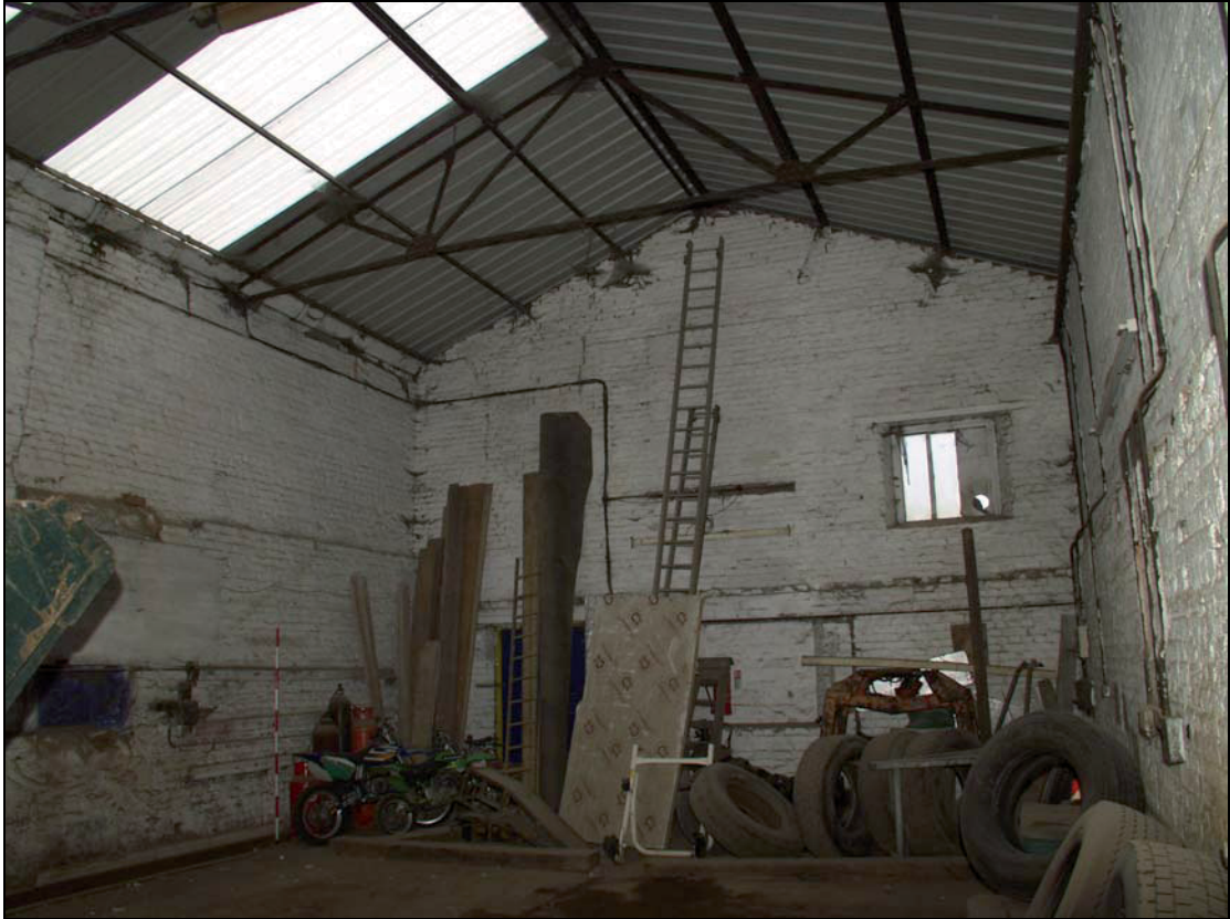
3 Building 1 – west bay, taken from the north-west (18)
