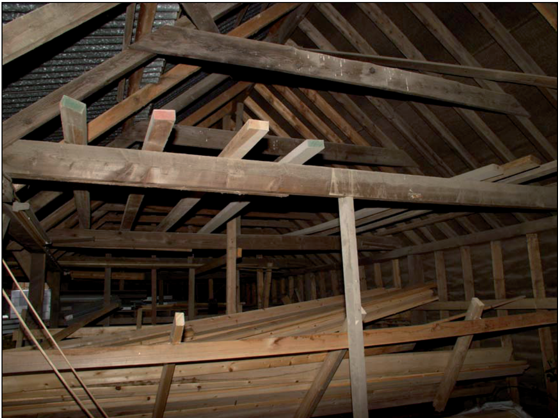
20 Building 4 – north section, taken from the south (35)
