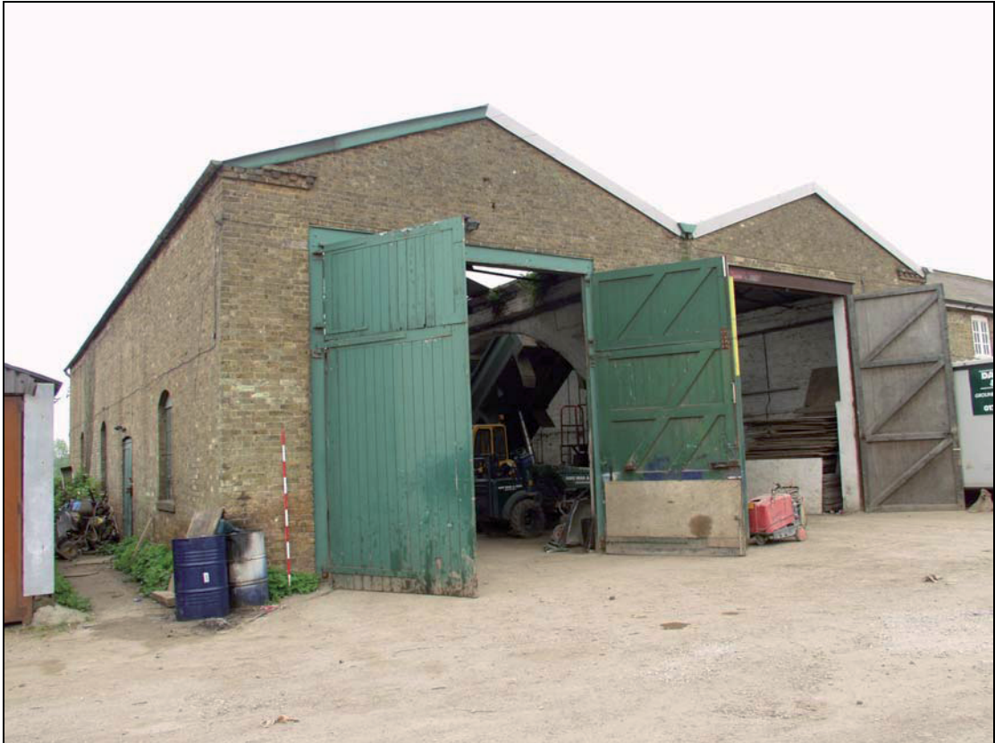
1 North and east elevations of Building 1, taken from the north-east (2)
