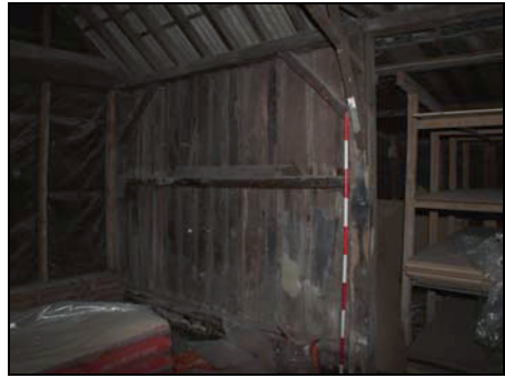
Wall framing and vertical boarding on west side of Building 4 – south section, taken from the north-east
