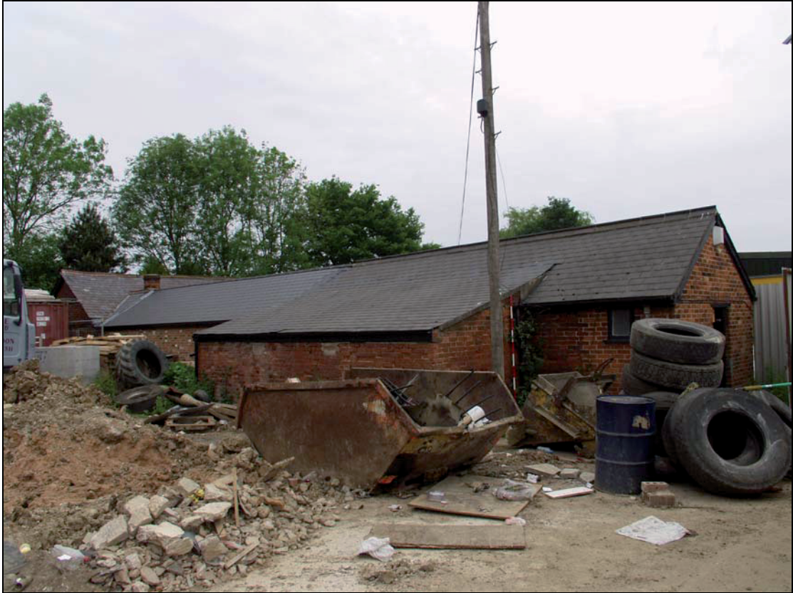
7 West elevation of Building 2, showing lean-to extension, taken from the south-west (10)
