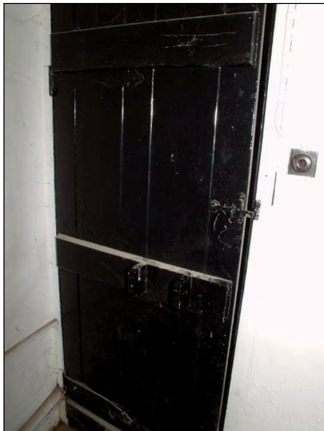
10 Early 20 th century boarded door within lavatory addition, Building 2, taken from the west (8)
