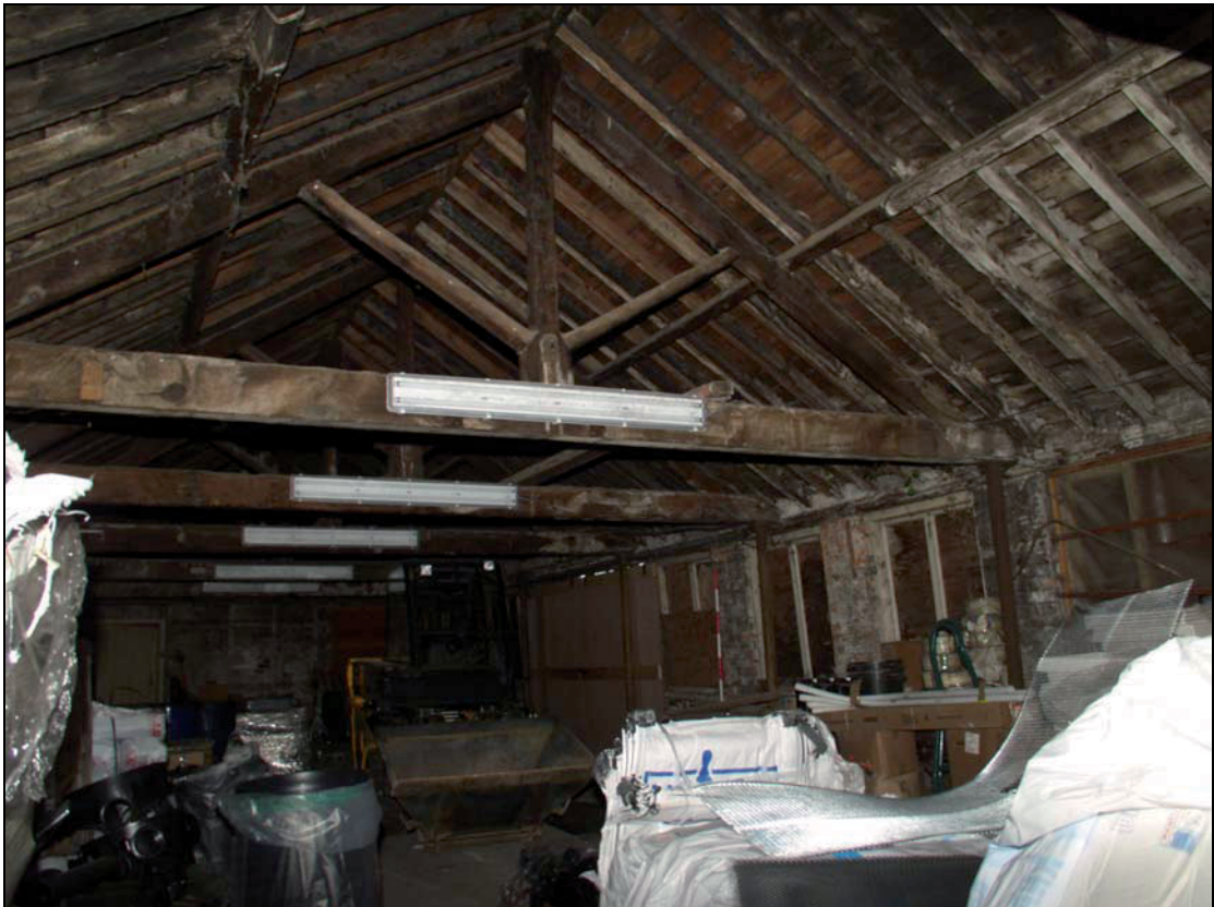
12 Interior of Building 3, taken from the north-west (27)
