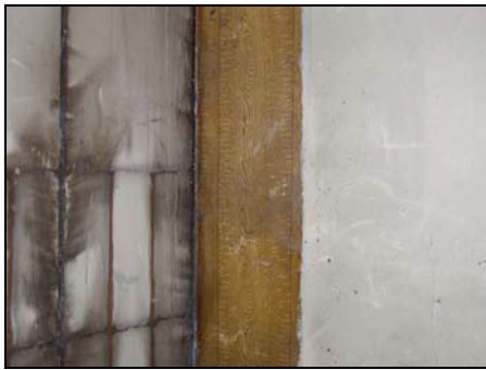
Grained match-line boarding on west wall of office in Building 3, taken from the east
