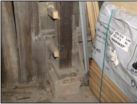
Lower butressing timber to post on west side of Building 4 – north section, taken from the north
