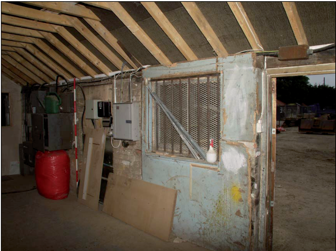
8 Interior of Building 2 – north section, taken from the south-west (4)
