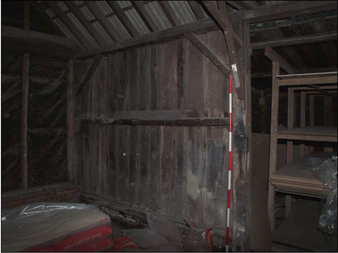
19 Wall framing and vertical boarding on west side of Building 4 – south section, taken from the north-east (38)
