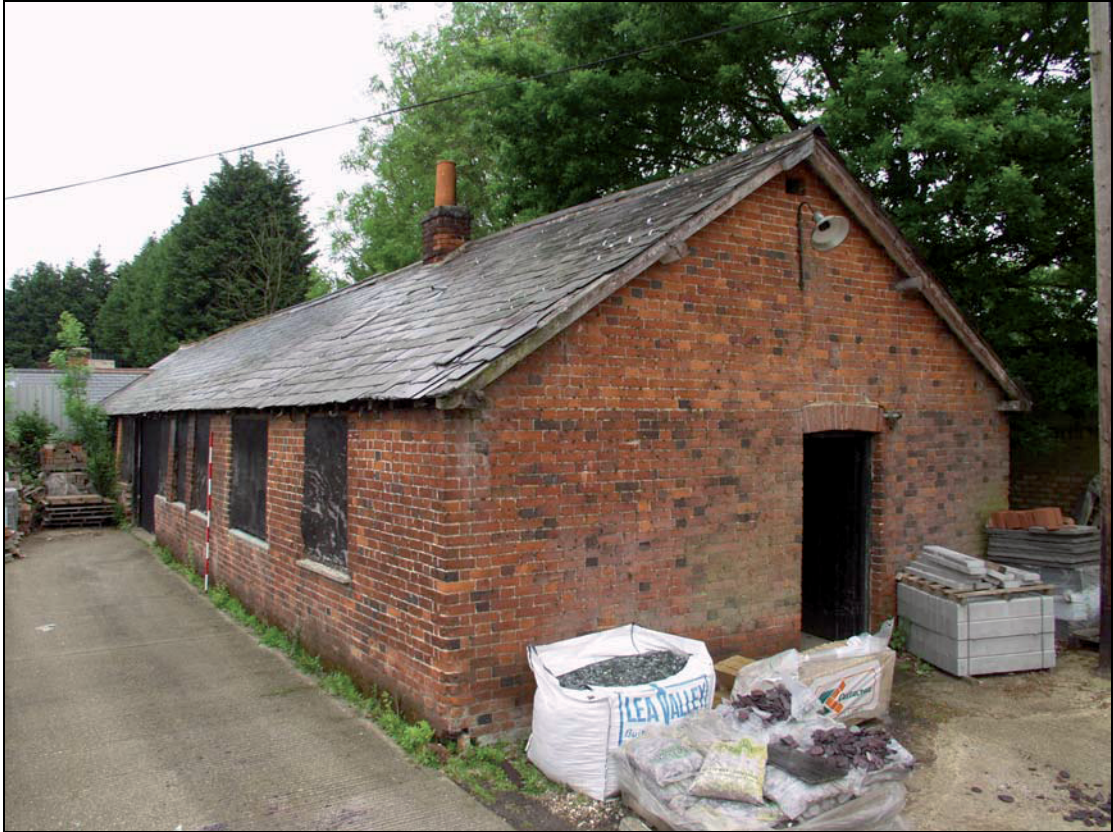
11 South and east elevations of Building 3, taken from the south-east (26)
