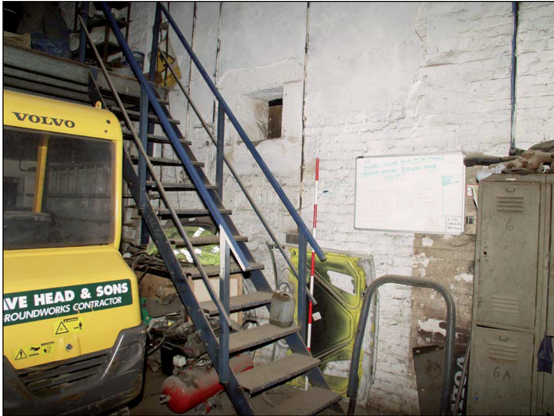
5 Stone-lined apertures in division wall in Building 1, taken from the north-east (23)
