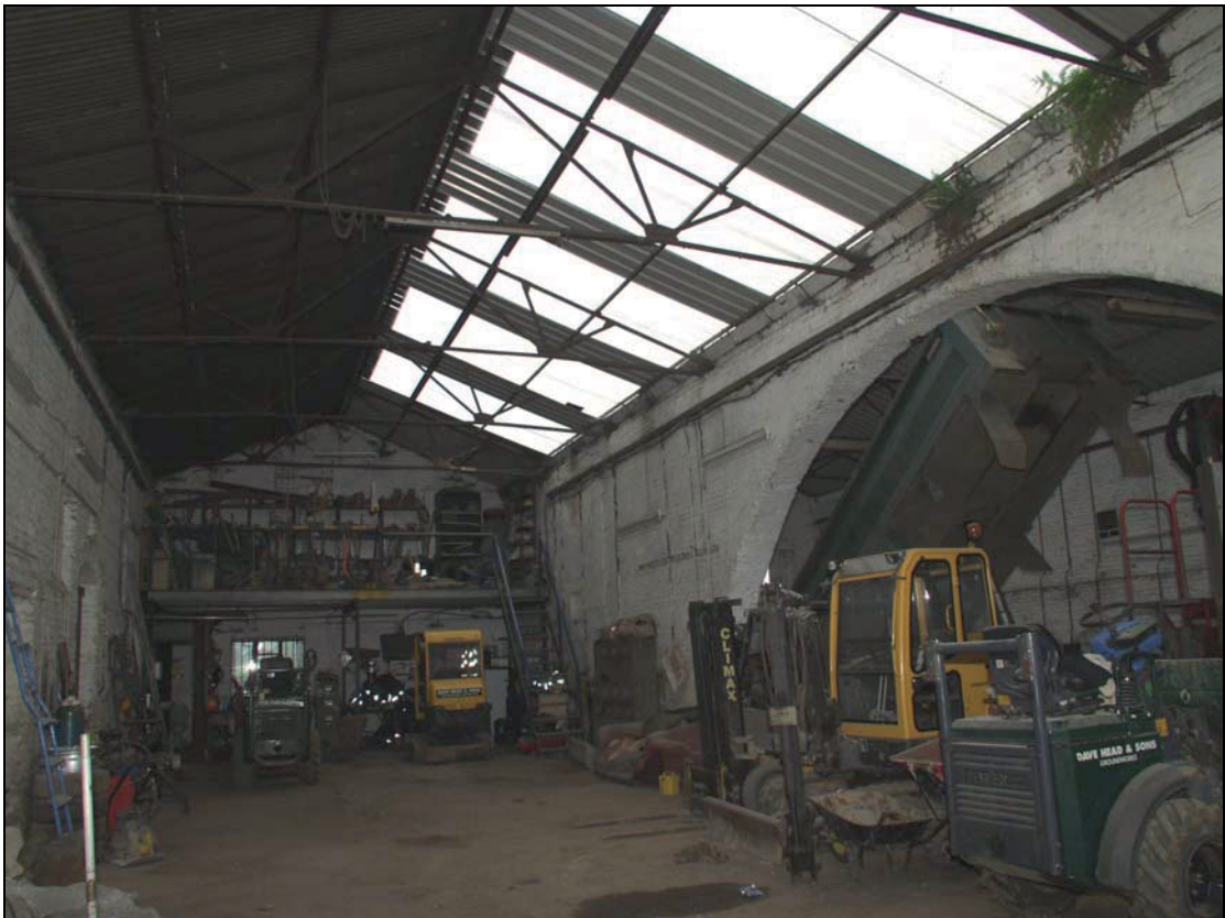
2 Building 1 – east bay, taken from the north (17)
