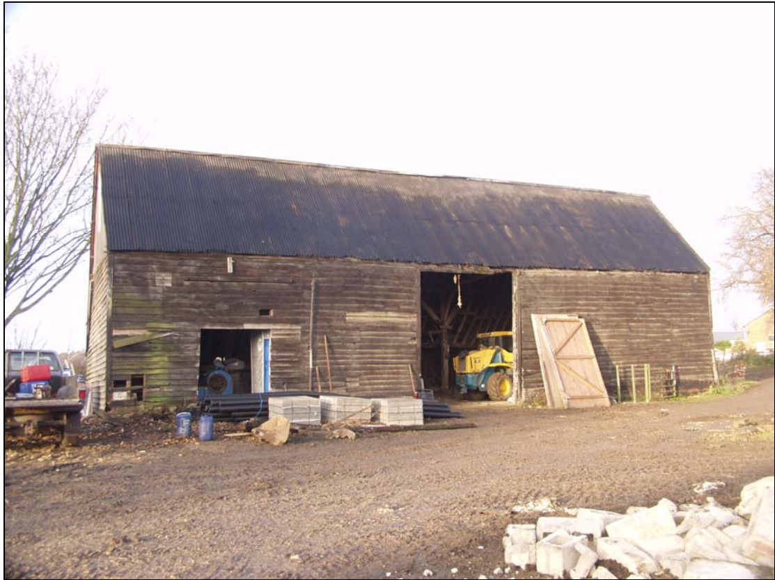
Plate 1 East elevation of Building 1, taken from the south-east (34)
