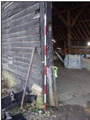
Detail of south door jamb showing housing for the threshing leap, taken from the north-east
