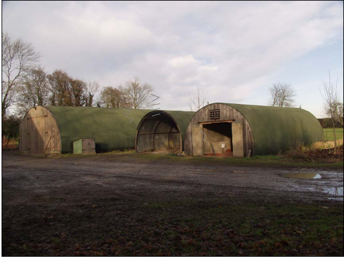
Plate 7 Exterior view of Buildings 2-4, taken from the south (1)
