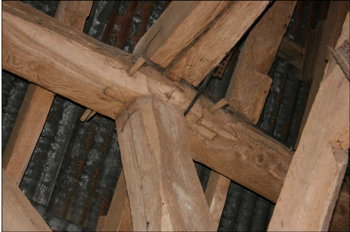
Plate 5 Detail of face-halved and bladed scarf joint in the arcade plate (west side of Truss 4, Building 1), taken from the south-east (62)
