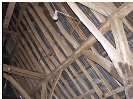
Detail of the roof pitch of Building 1 showing the bladed rafters, taken from the north-east
