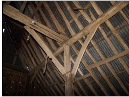
Construction detail of Truss 4 (west side of Building 1), taken from the north-east
