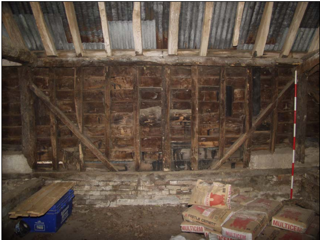
Plate 4 West wall of Bay 2 (Building 1), taken from the east (49)
