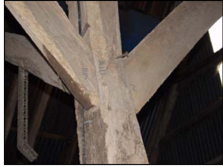
Assembly marks (emphasised) on the arcade braces (west side of Truss 4, Building 1), taken from the north-west
