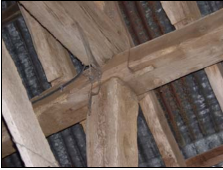
Detail of face-halved and bladed scarf joint in the arcade plate on the west side of Truss 3 (Building 1), taken from the north-east
