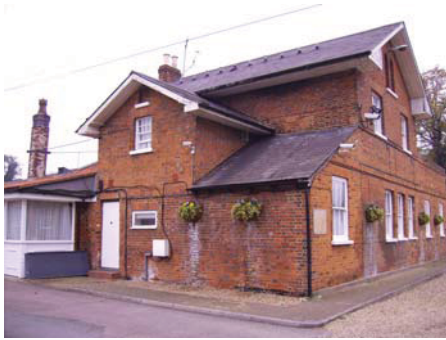
DP31 South-western frontage of the former stable building, which is adjoined to the main hotel building by a single storey extension, view north-east
