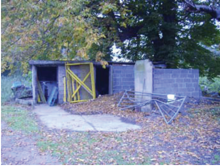
DP19 Breeze-block built outhouse or workshop located towards the centre of the hotel's grounds and besides the River Lea, view north
