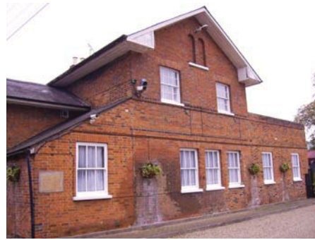
DP32 South-eastern frontage of the former stable building, which is known as The Coach House section of Bush Hall Hotel, view north
