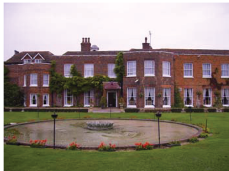
DP24 South-eastern and main frontage of Bush Hall Hotel, with the sunken fountain feature in the foreground, view north-westwards
