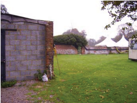
DP21 Corner of the modern extension to the outbuilding, with a prefab buildings, original garden walls and The Pavilion beyond, view east
