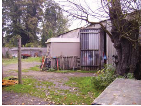
DP20 Modern extension to the outbuilding located to the north of Bush Hall Hotel and towards the northern section of the site, view eastwards
